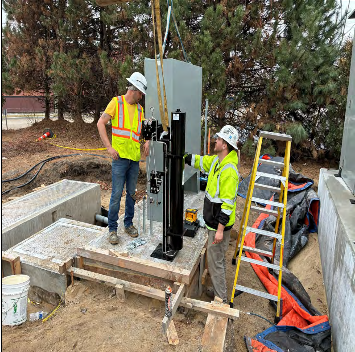
Figure 15 – Installing New Rexa Actuator on Equipment Pad @ Chapaton PS
