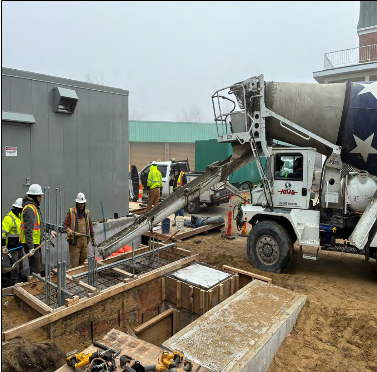
Figure 12 – Placing Concrete for Telemetry Access Hatch & Rexa Equipment Pad @ Chapaton
