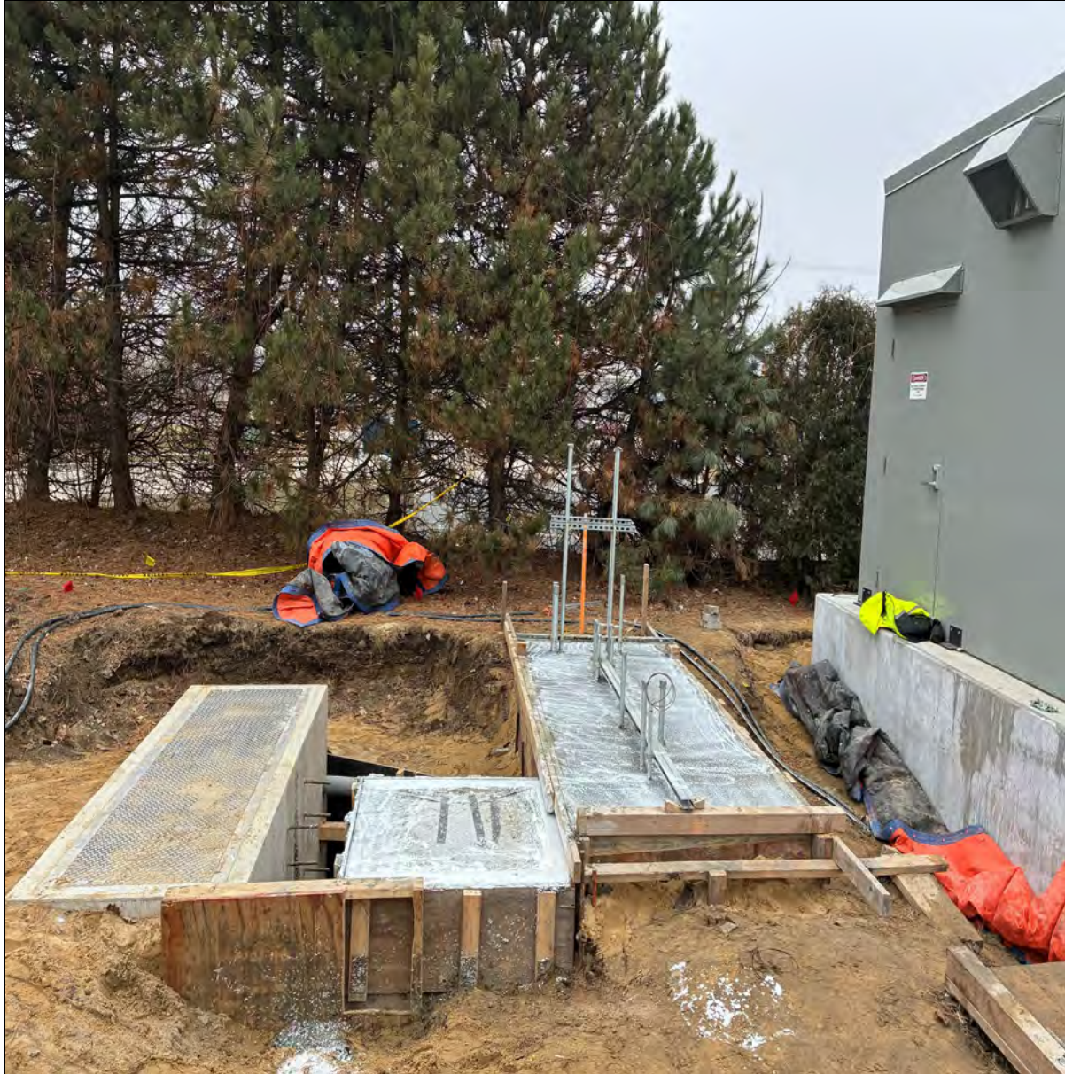
Figure 13 – Concrete for Telemetry Access Hatch & Rexa Equipment Pad @ Chapaton PS
