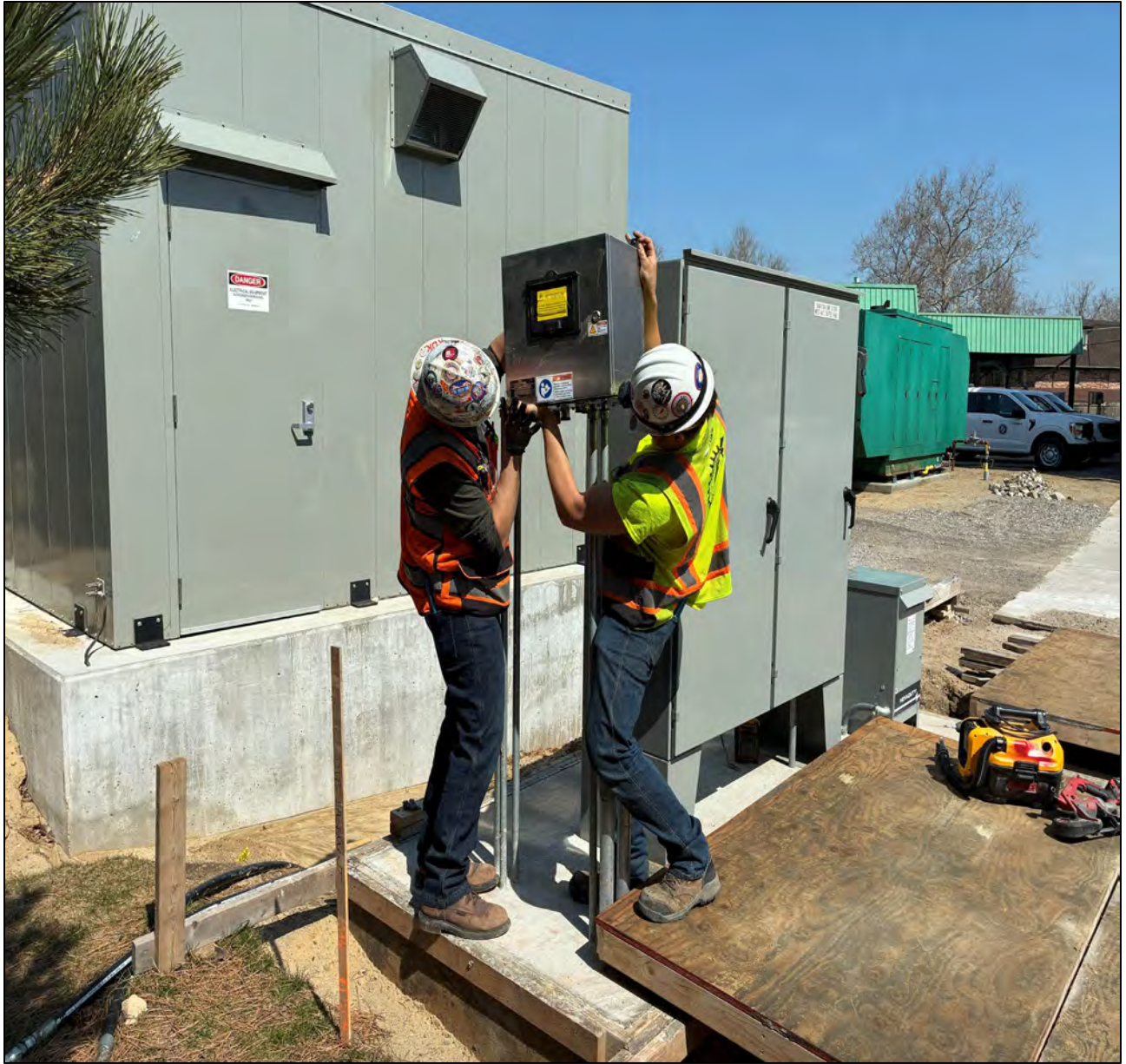
Figure 17 – Installing New Displays on Rexa Equipment Pad @ Chapaton PS
