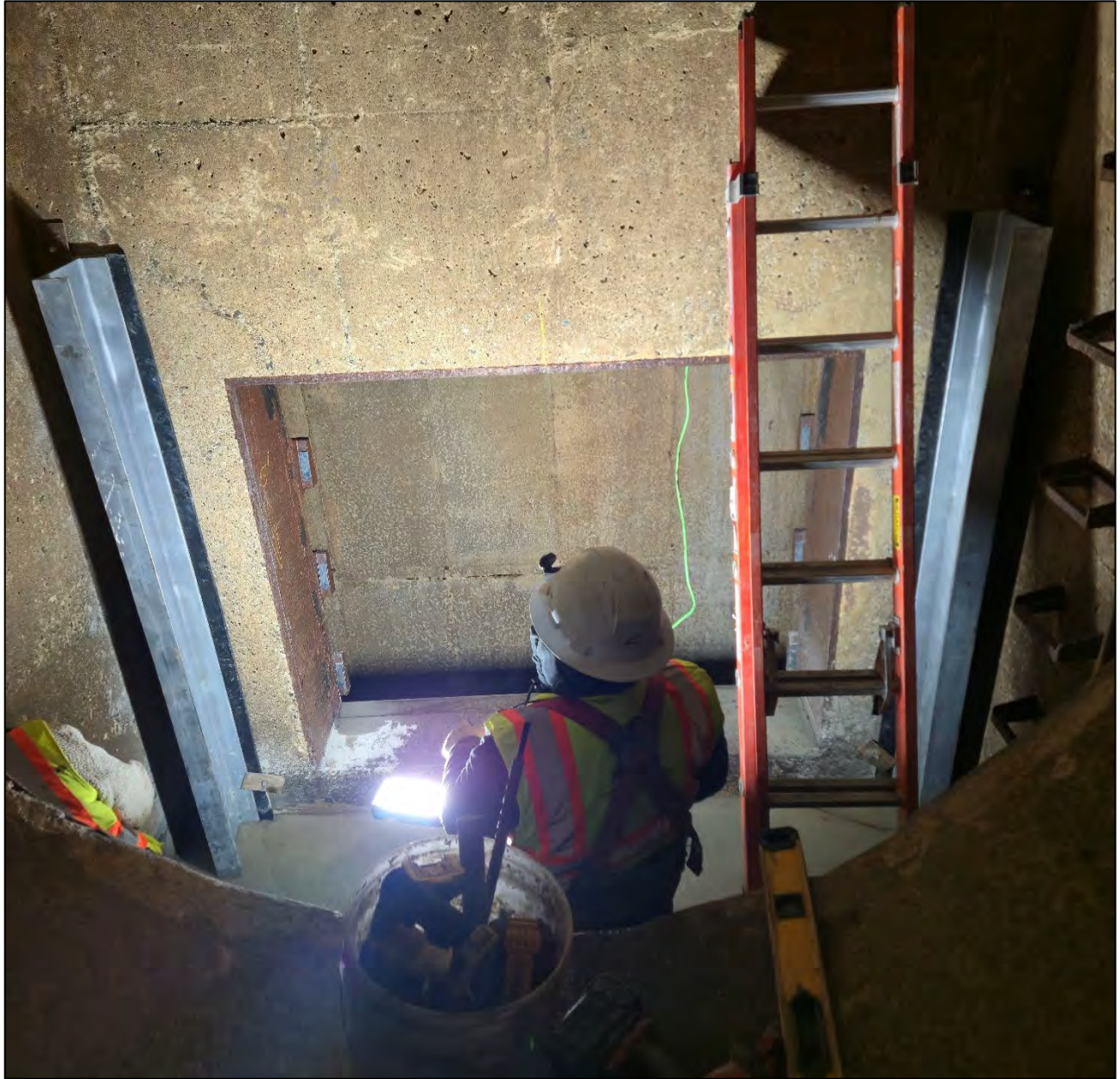
Figure 22 – Installing Stop Log Guide Rails in Station Gate Vault @ Chapaton PS
