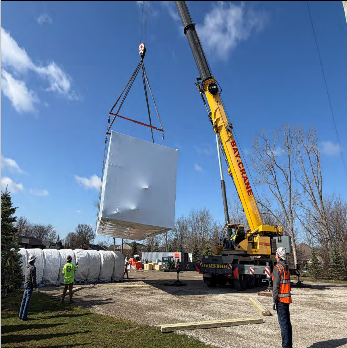
Figure 10 – Unloading E-House @ 15 Mile Fraser Bio-Filter Site
