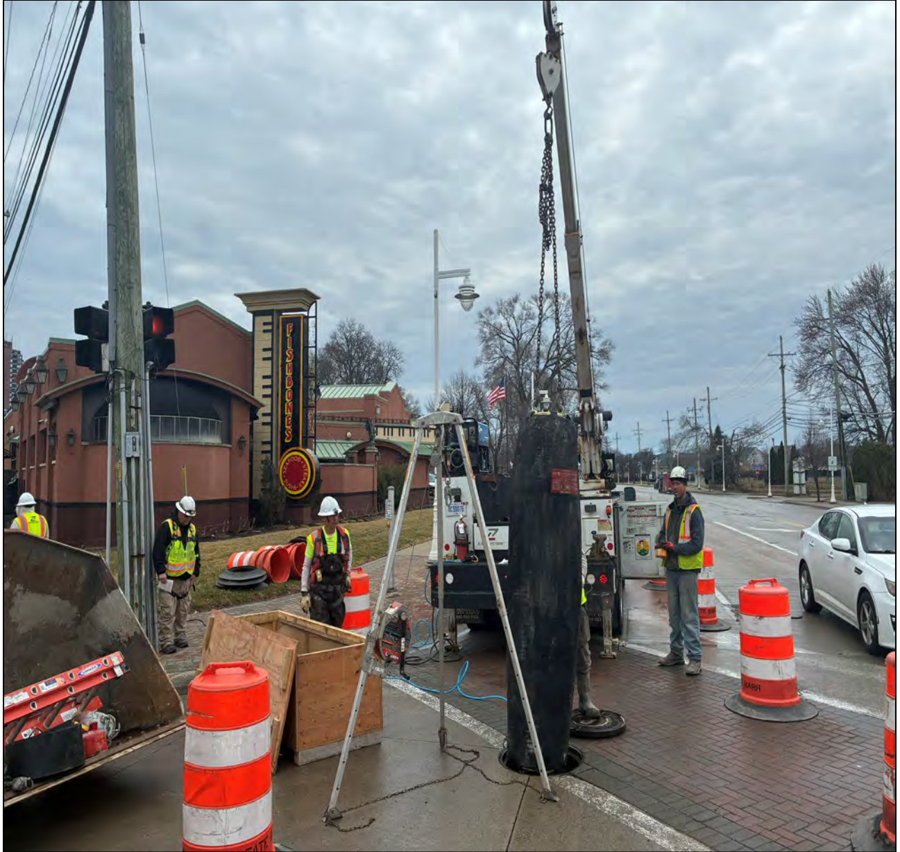
Figure 18 – Placing Temporary Pipe Plug into RTB Drain @ Chapaton PS
