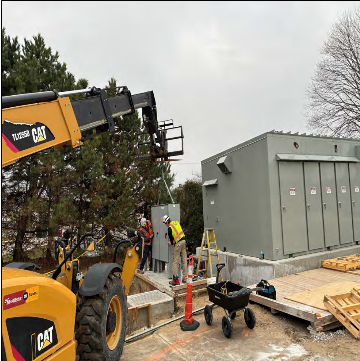
Figure 14 – Installing New Rexa Control Cabinet on Equipment Pad @ Chapaton PS
