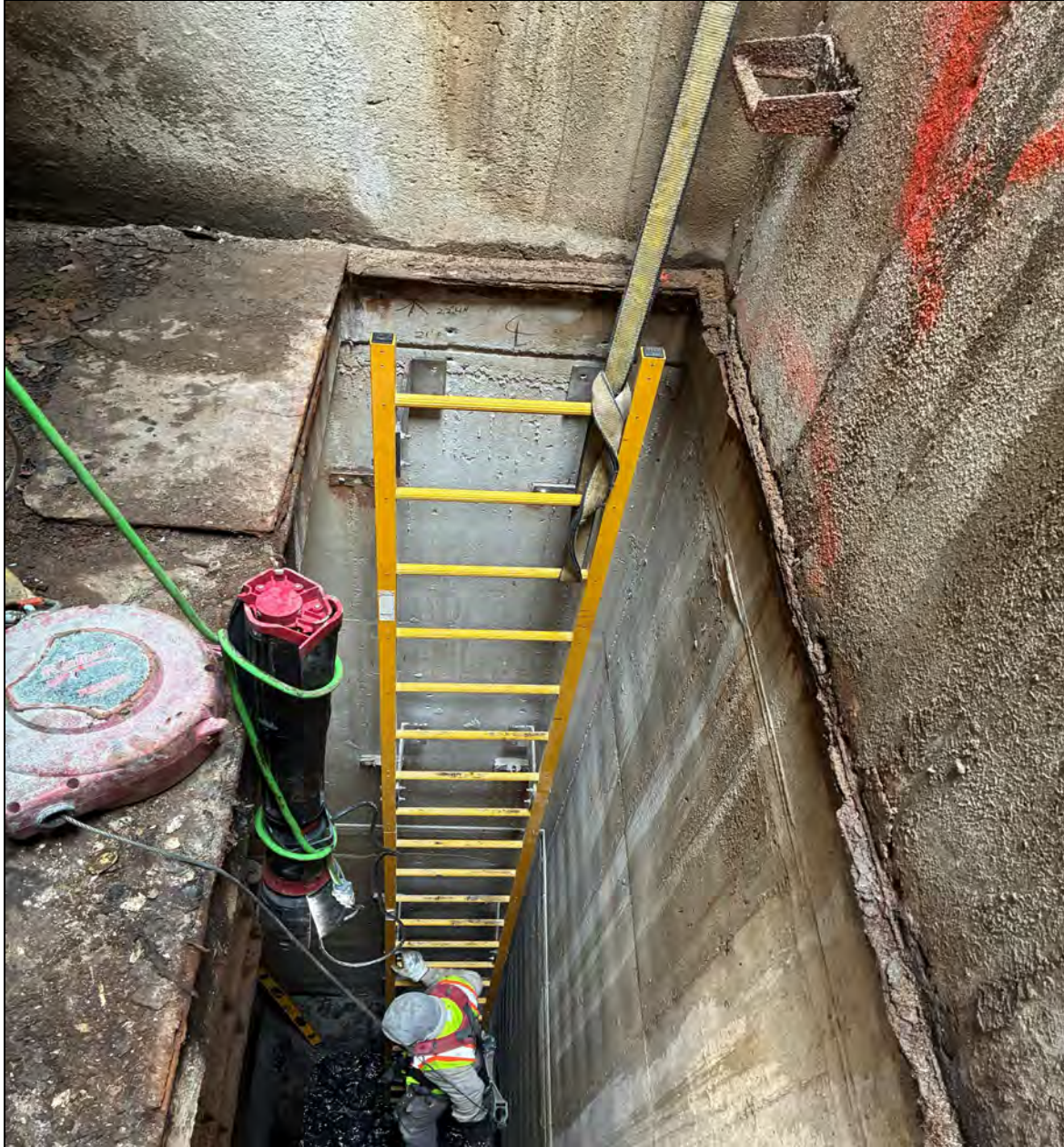
Figure 21 – Installing New FRP Ladder in Diversion Chamber @ Chapaton PS
