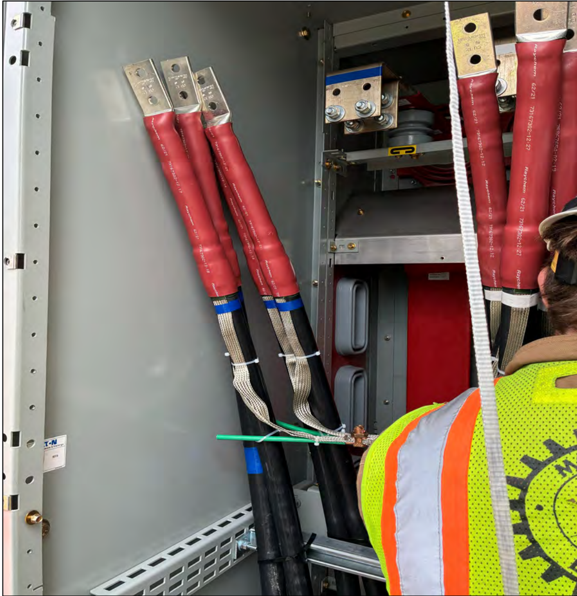
Figure 5 – Preparing Cable to Buss Bar Connections in Outdoor E-House @ Chapaton PS
