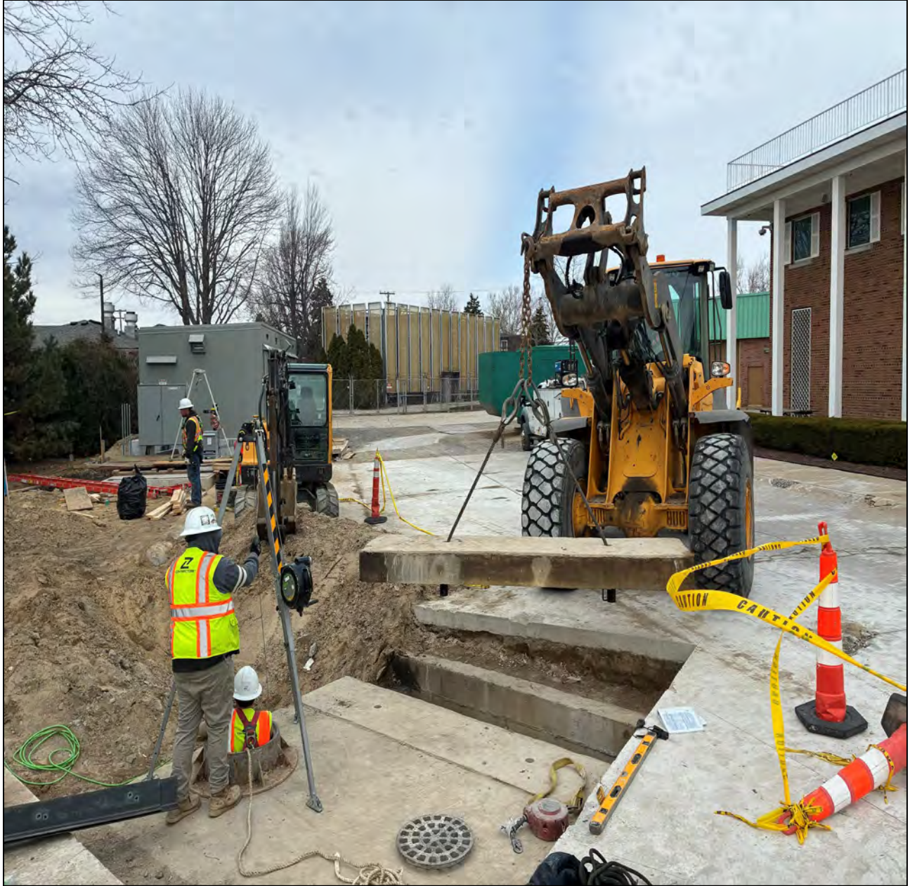
Figure 20 – Removing Station Gate Vault Roof Panels @ Chapaton PS
