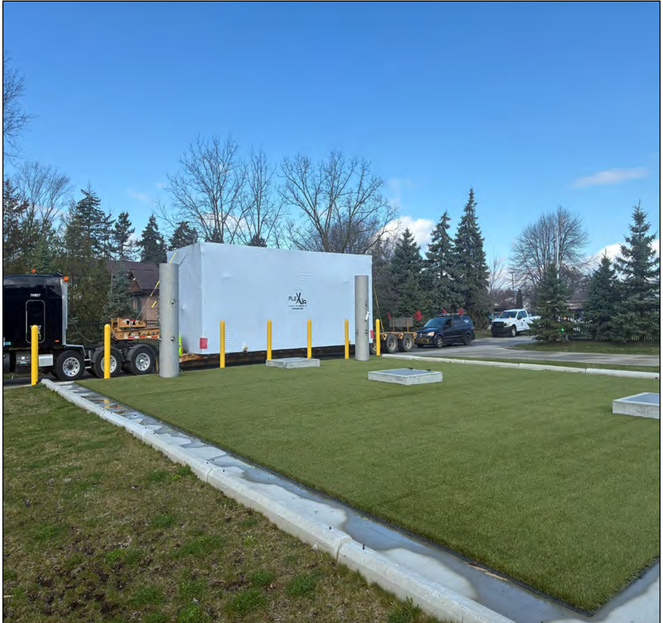
Figure 9 – Transporting 2MW E-House @ 15 Mile Fraser Bio-Filter Site
