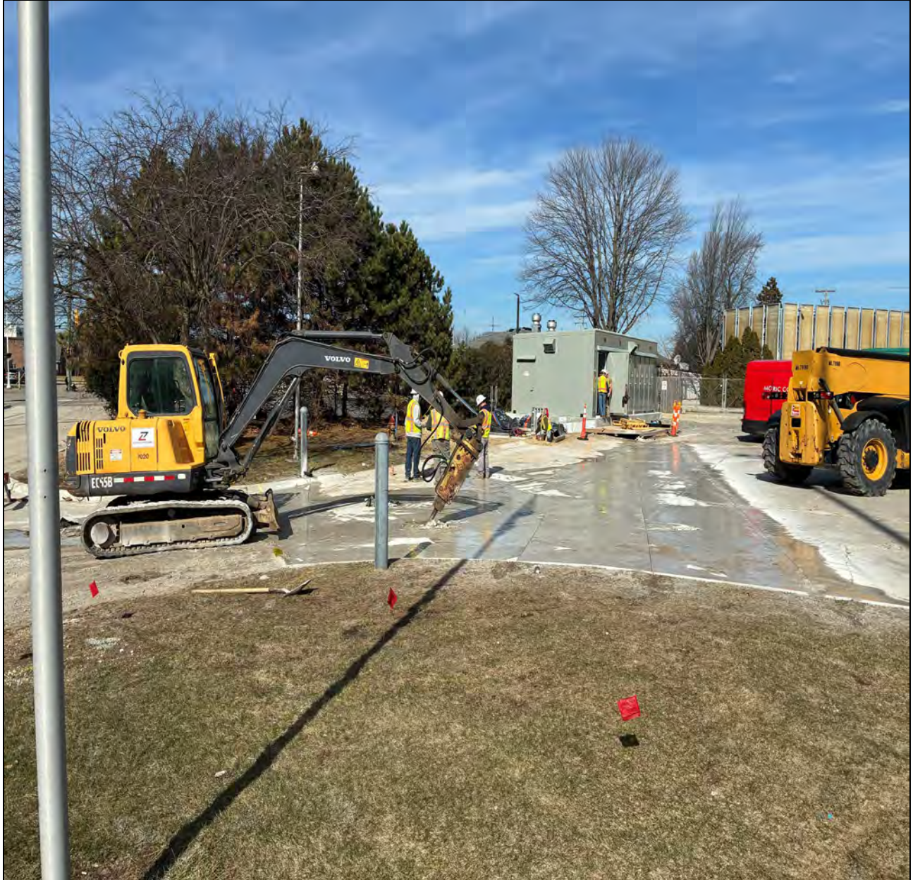
Figure 19 – Removing Concrete to Access Station Gate Vault @ Chapaton PS
