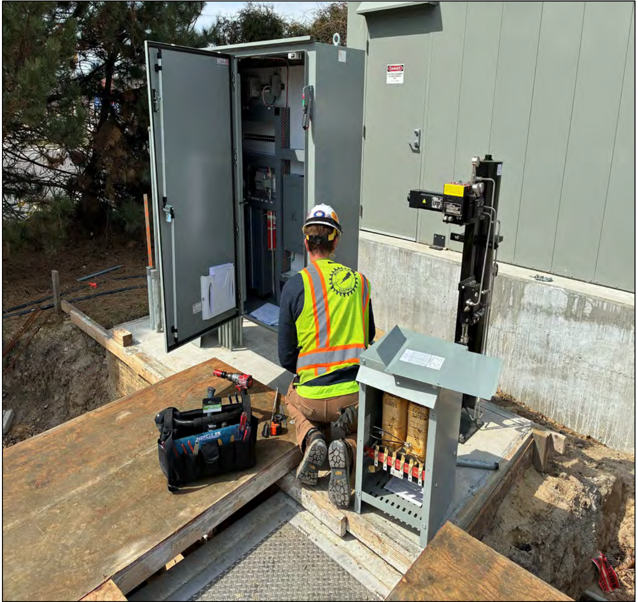
Figure 16 – Installing New Transformer on Rexa Equipment Pad @ Chapaton PS
