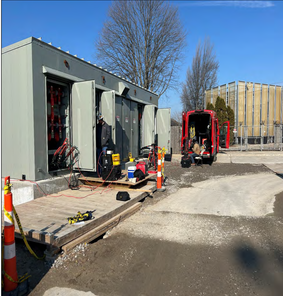
Figure 6 – Testing Cables Between DTE and Dist. Gear @ Chapaton PS
