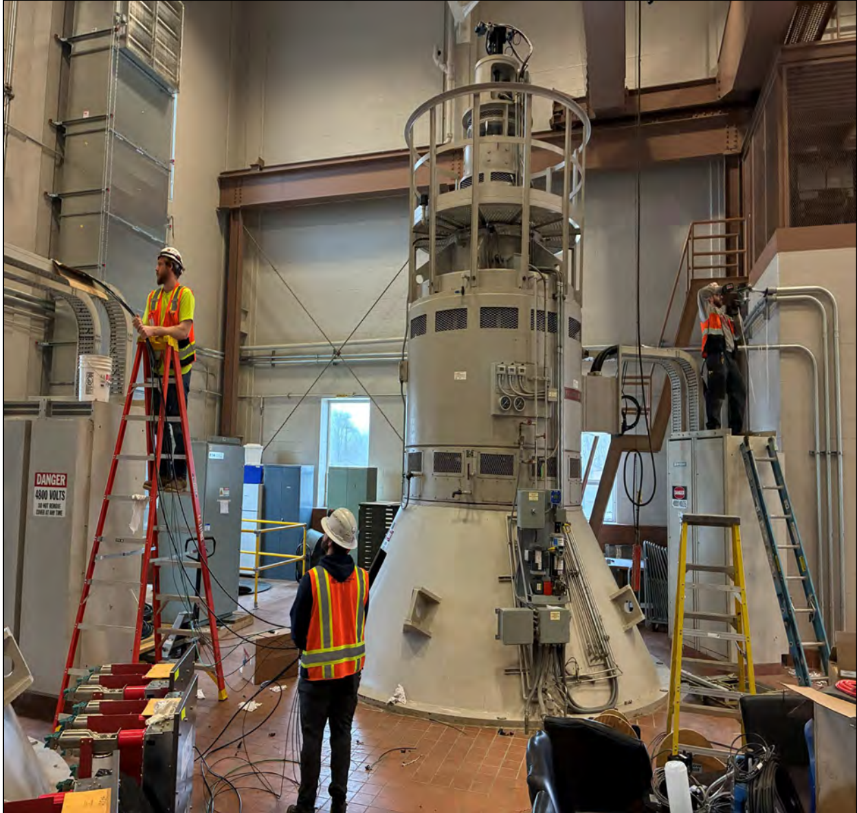
Figure 1 – Pulling Control Cable on Main Floor @ Chapaton PS
