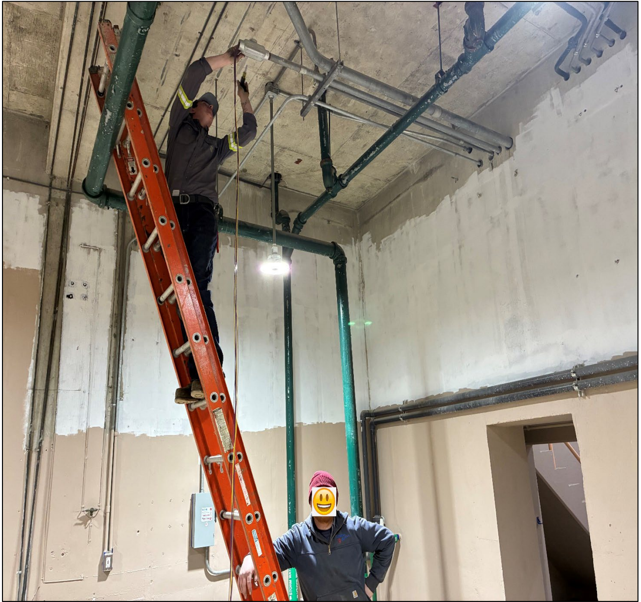
Figure 2 – Installing Electrical Conduits at Martin RTB Basement
