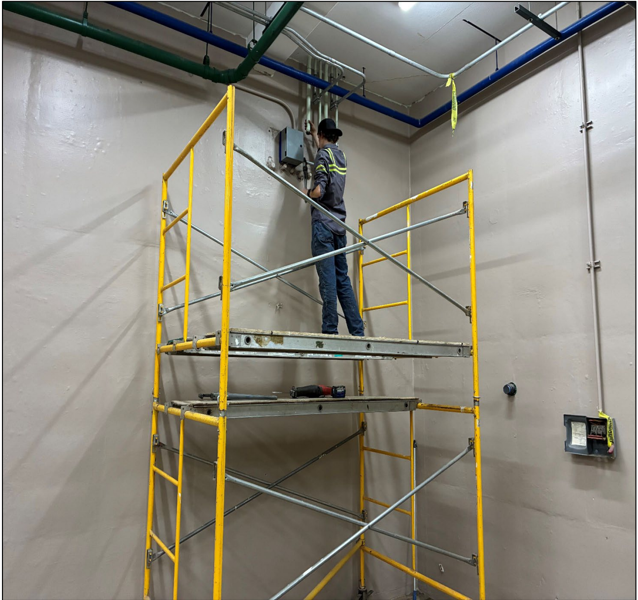
Figure 3 – Removing Abandoned Electrical Conduits at Martin RTB Basement
