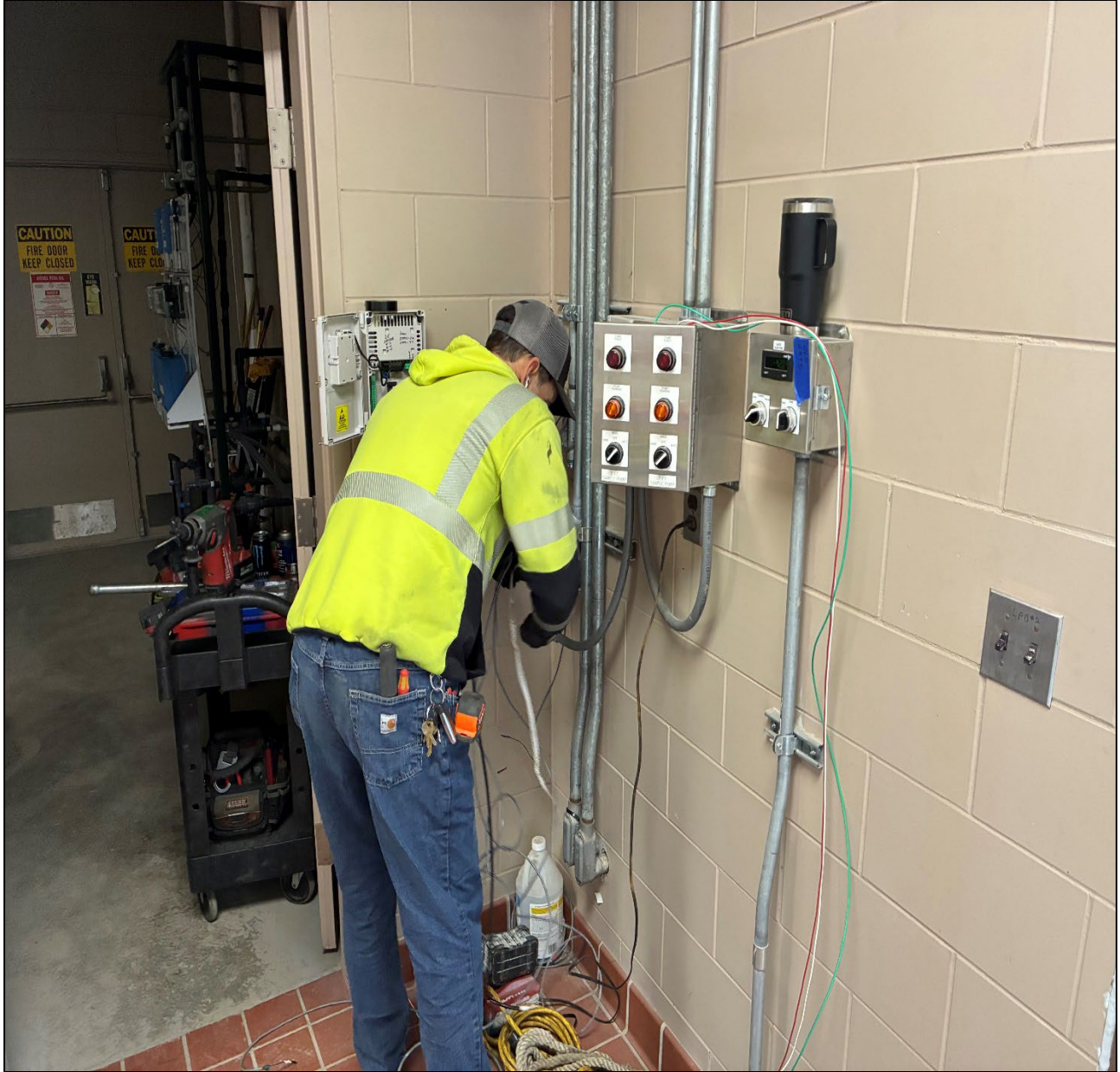
Figure 1 – Installing New Dewatering Gate Sensors and Controls
