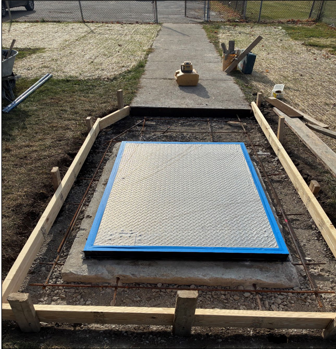
Figure 3 – Install New East Access Hatch at Martin Basin
