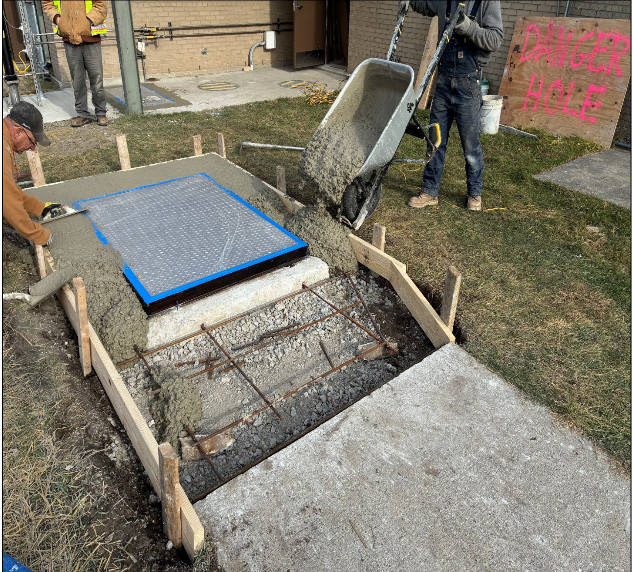
Figure 4 – Embedding New Access Hatches with Concrete at Martin RTB
