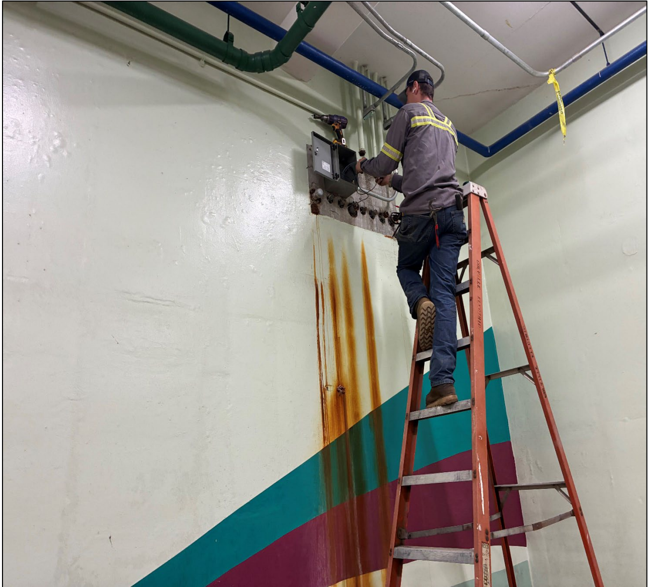
Figure 1 – Install New Electrical Junction Inside Martin Basement
