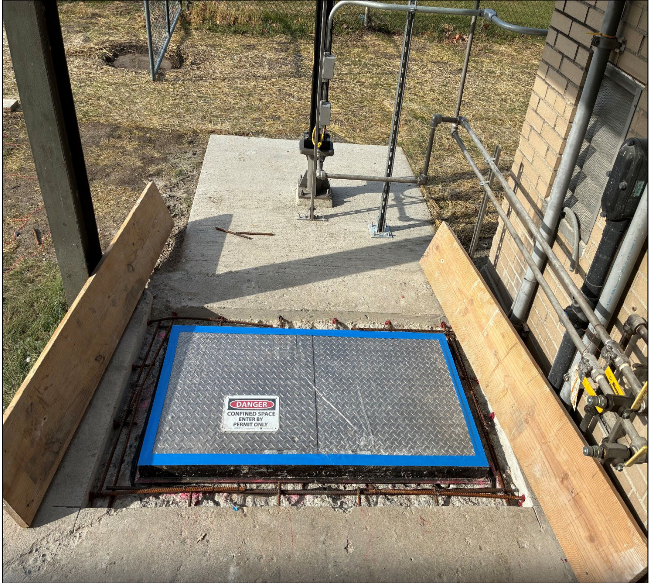
Figure 2 – Installed New Dewatering Gate Access Hatch at Martin Basin
