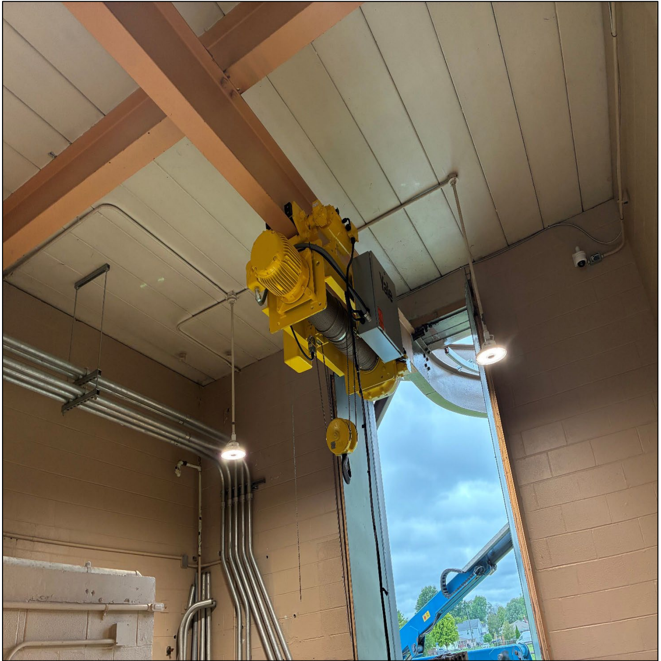
Figure 3 – New Martin RTB Trolley Hoist
