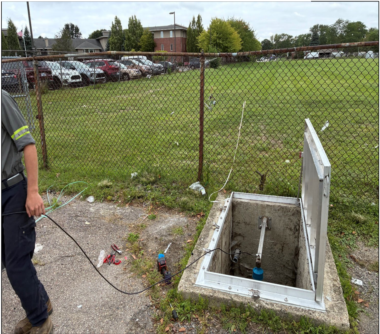
Figure 1 – Installing Martin RTB Level Sensor
