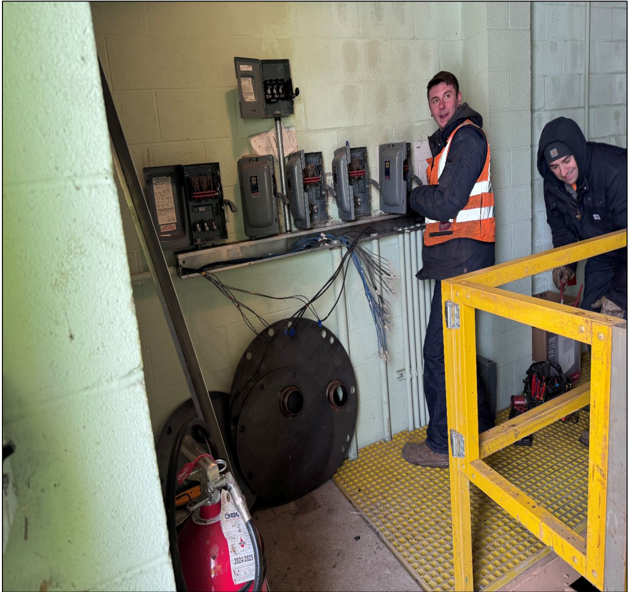
Figure 1 – Removing Electric Disconnects from Flushing Chamber A
