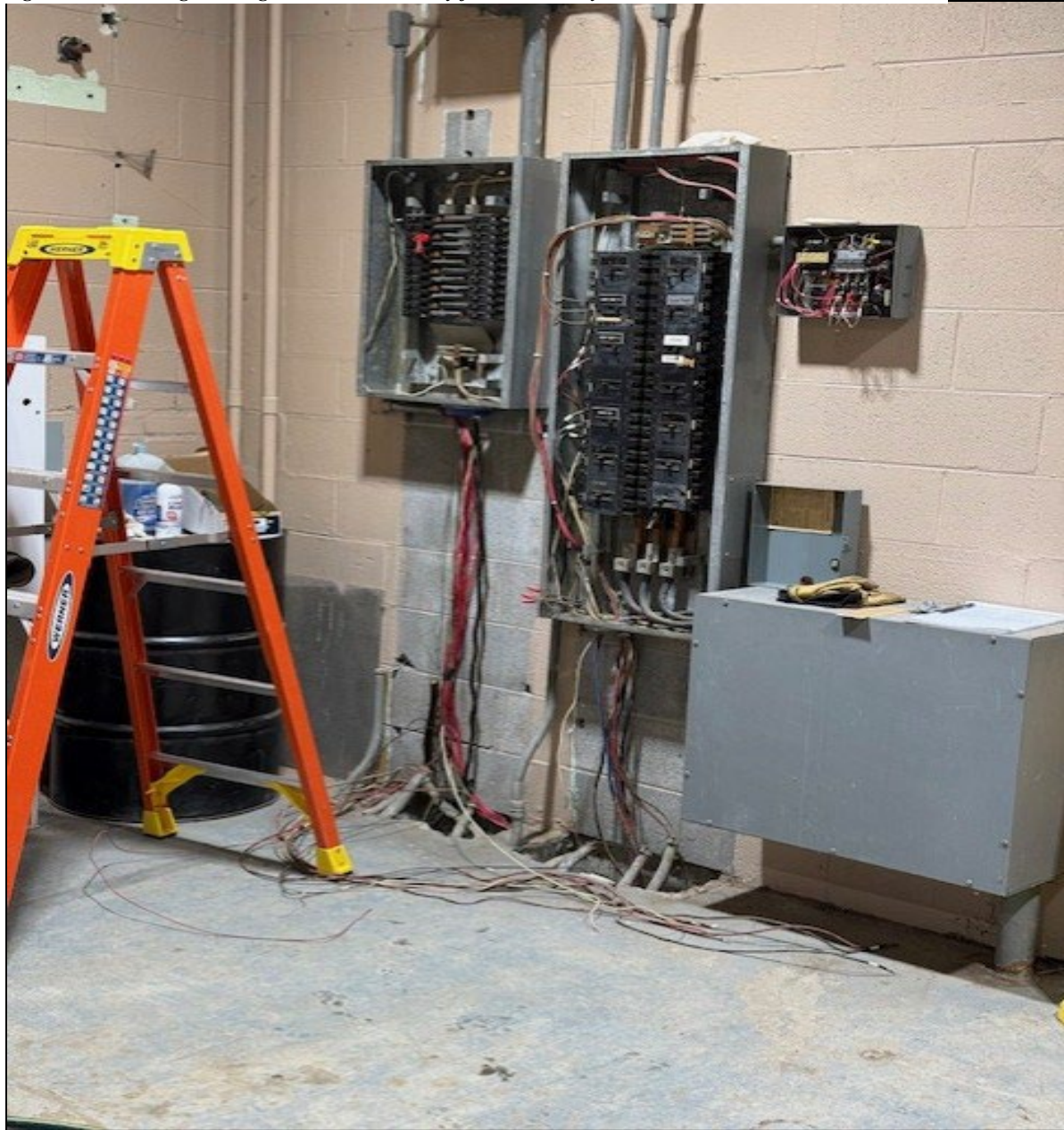
Figure 4 – Removing Existing Electrical in Facility for New Trolley Hoist Panel
