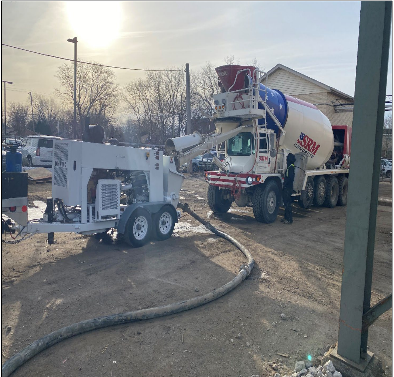
Figure 7 – Pumping Conc. Flow Fill Inside Abandoned Flushing Pipes
