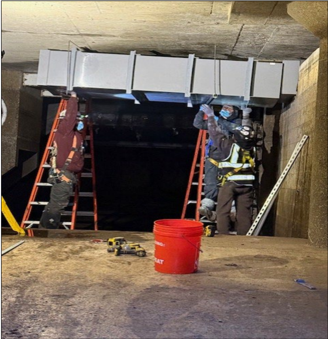
Figure 12 – Installing New Ventilation Ducts Inside Martin Basin
