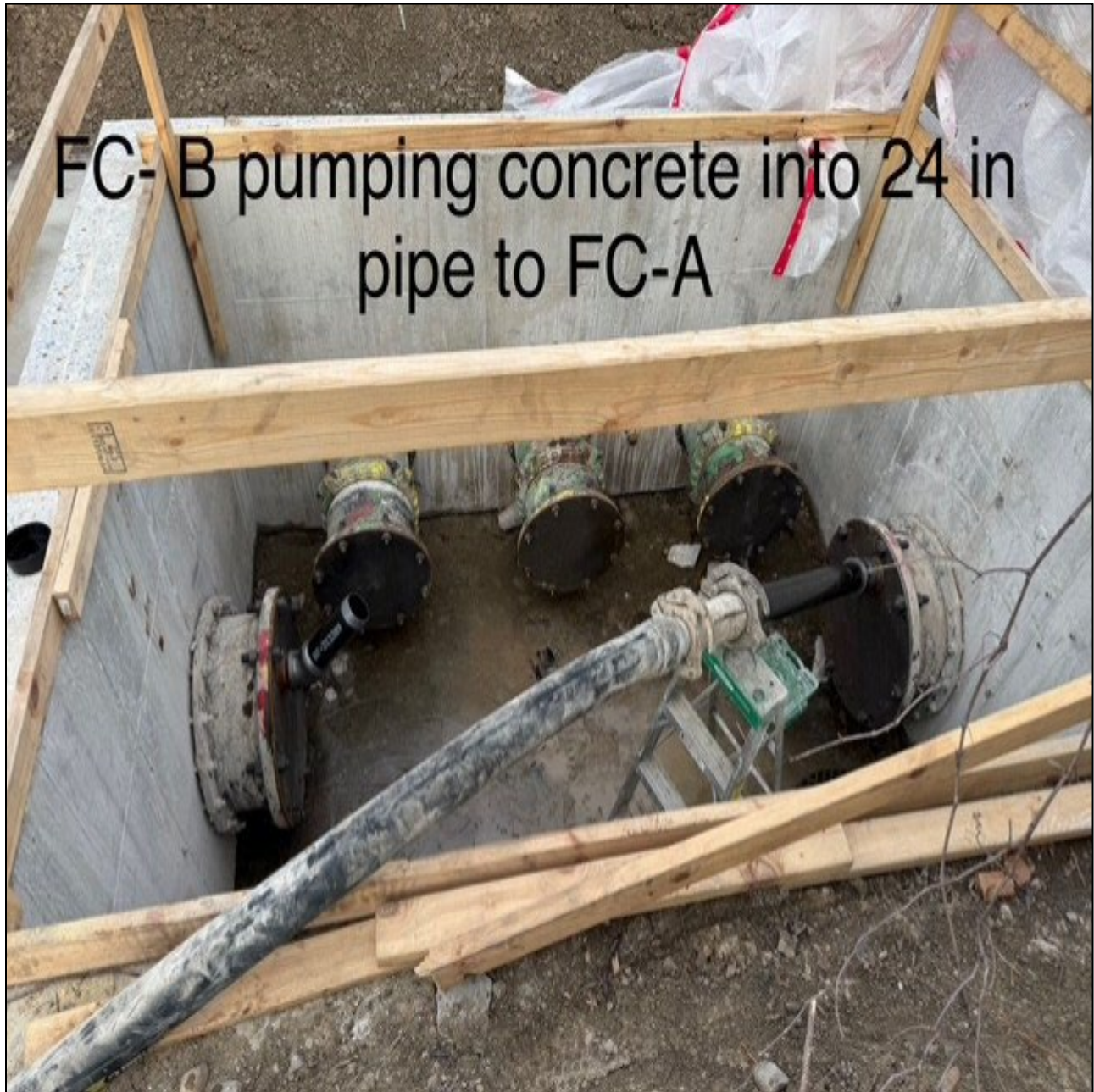
Figure 10 – Placing Conc. Flow Fill Inside Abandoned Flushing Pipes
