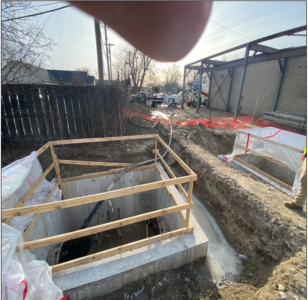
Figure 8 – Placing Conc. Flow Fill Inside Abandoned Flushing Pipes
