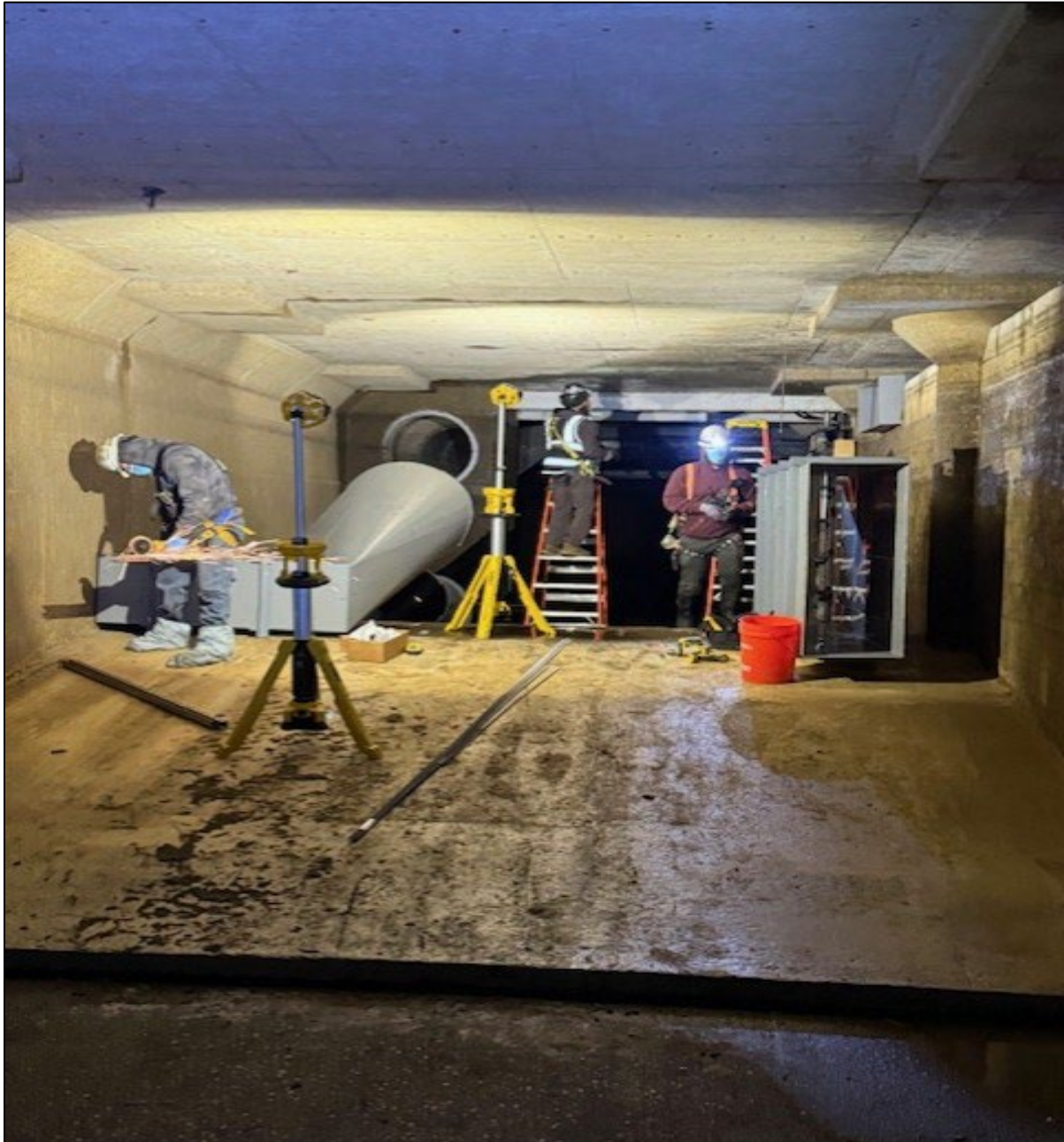
Figure 11 – Installing New Ventilation Ducts Inside Martin Basin
