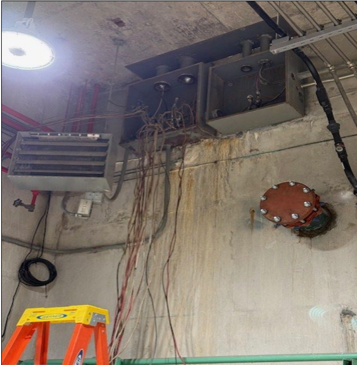
Figure 3 – Removing Electrical from Inside Facility Basement
