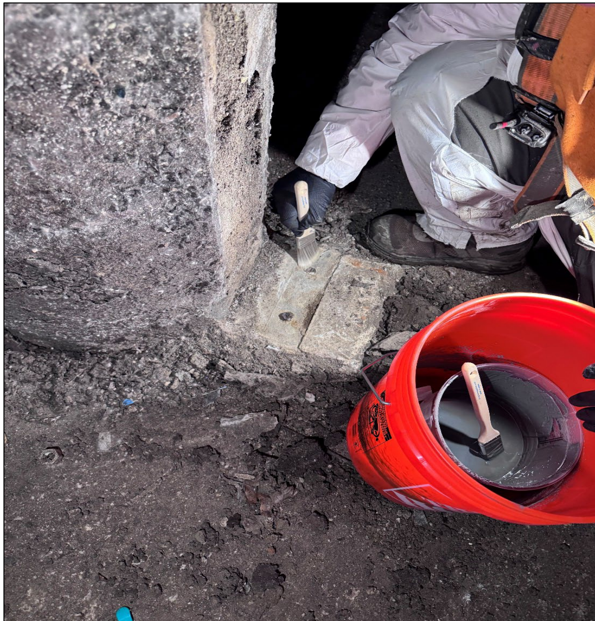
Figure 5 – Applying Corrosion Resistant Material to Abandoned Anchors in Basin.
