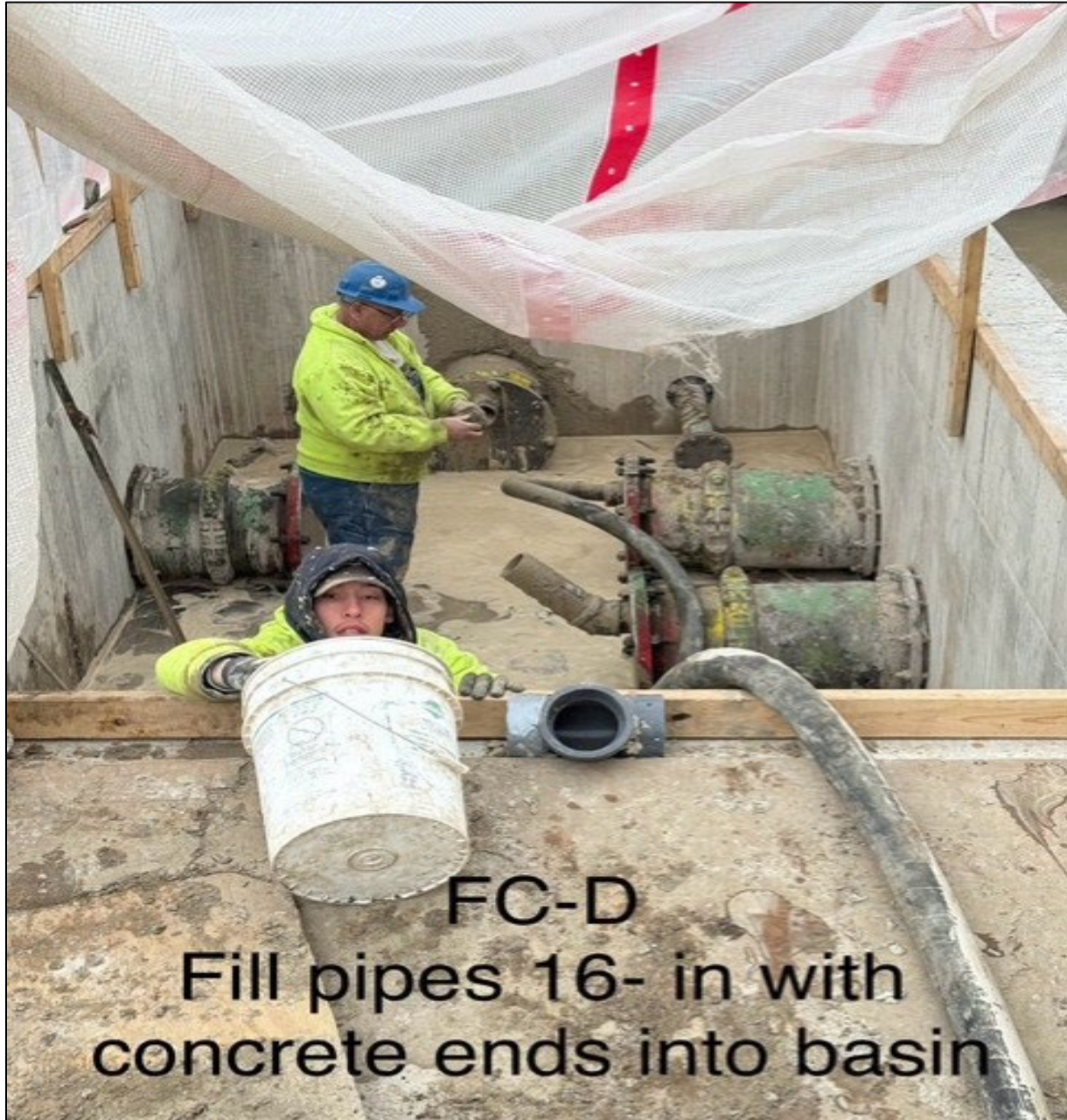
Figure 9 – Placing Conc. Flow Fill Inside Abandoned Flushing Pipes
