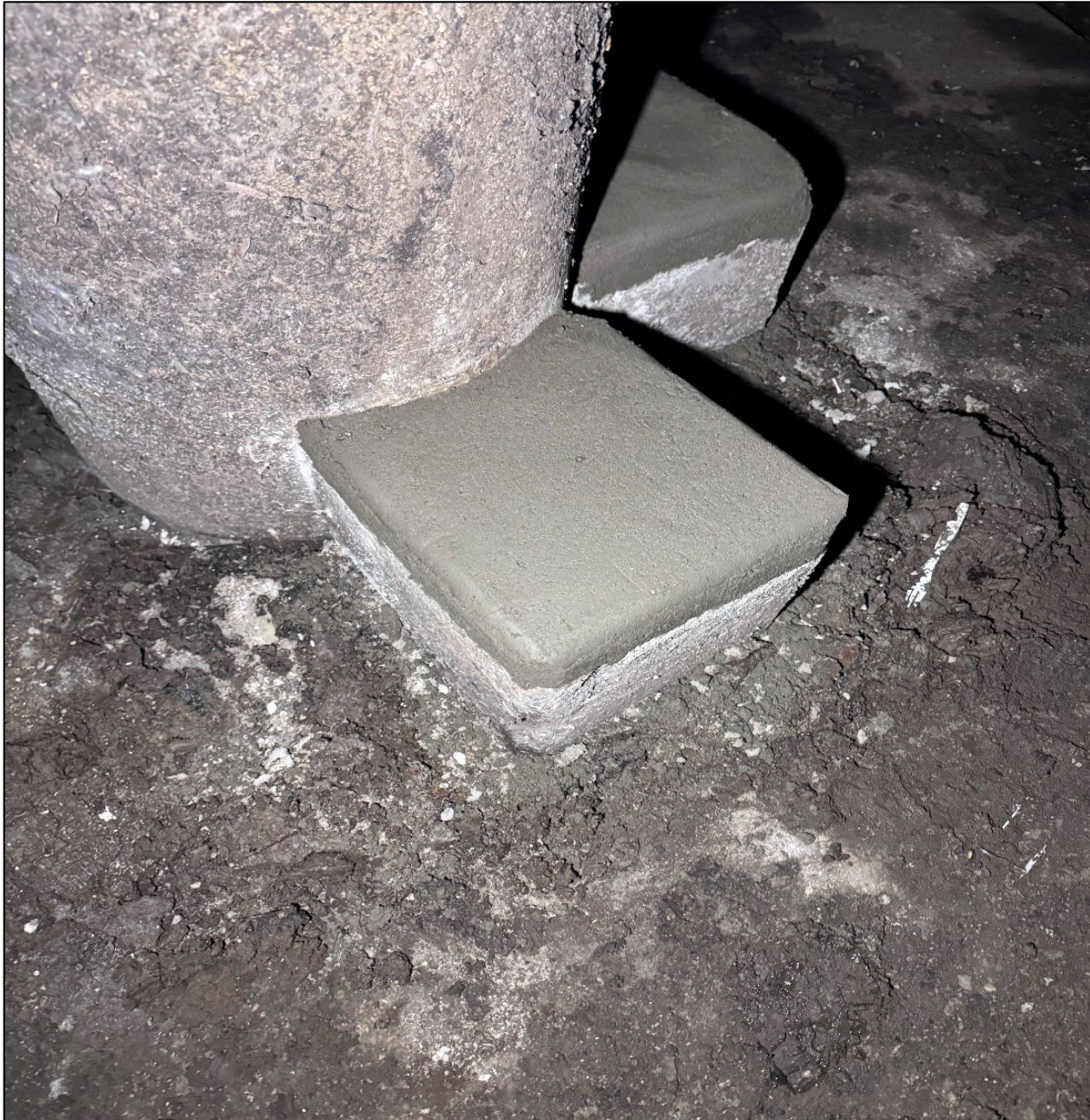
Figure 6 – Restoring Concrete Support Pad in Martin Basin
