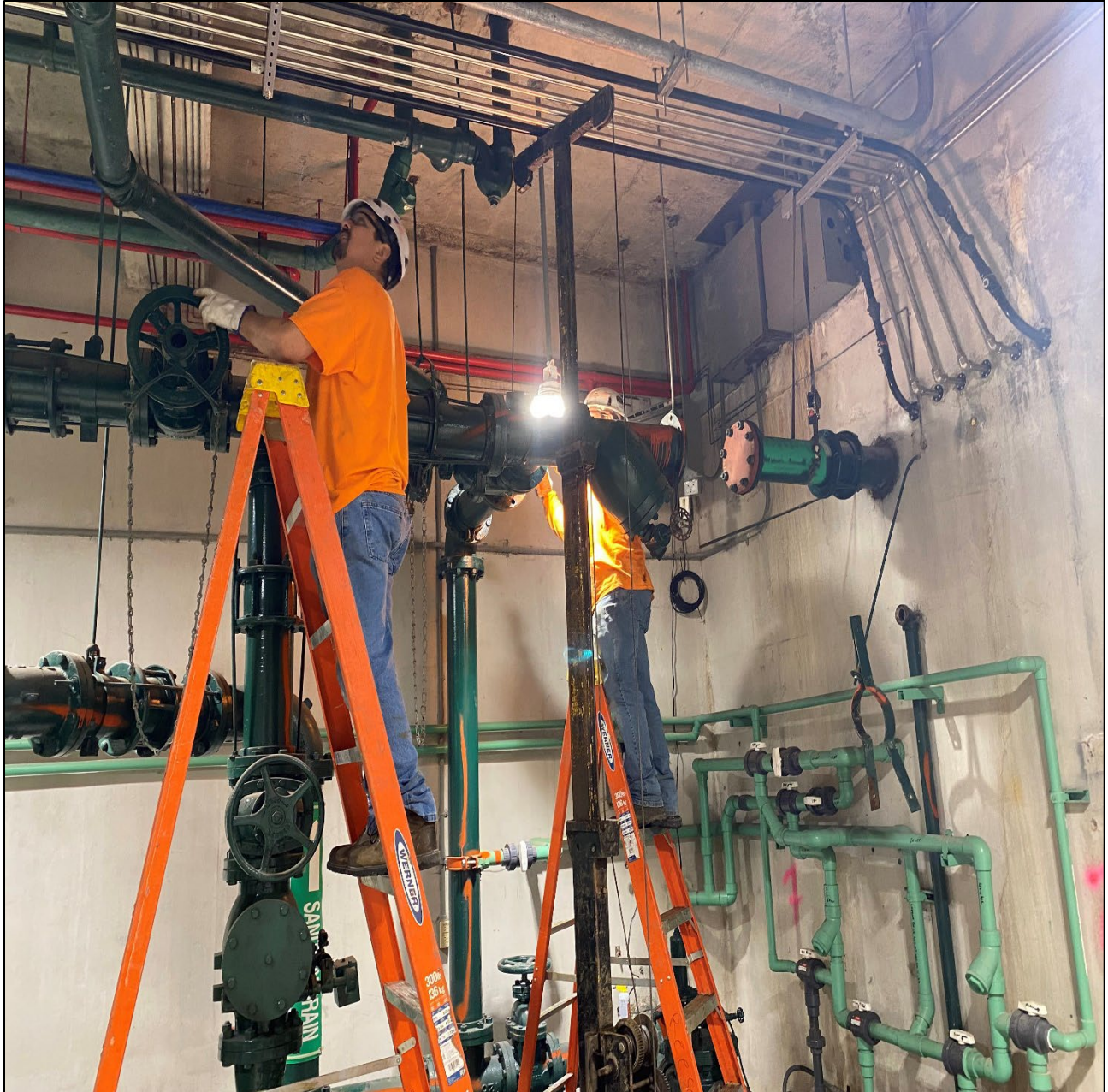
Figure 3 – Removing Existing 6-Inch Flushing Pipe In Station Basement
