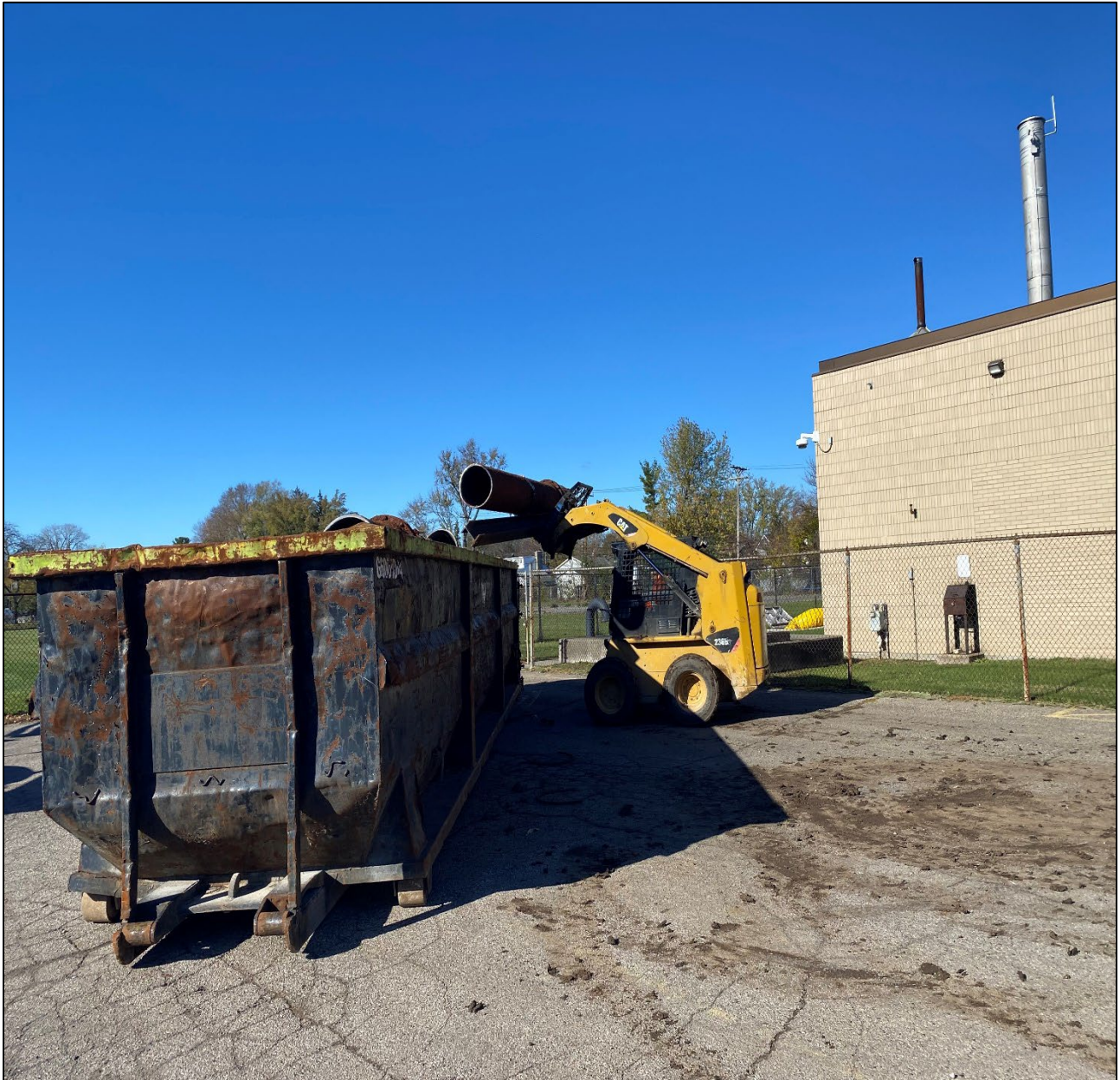
Figure 9 – Loading Out old Flushing Pipe & Supports at Martin Station
