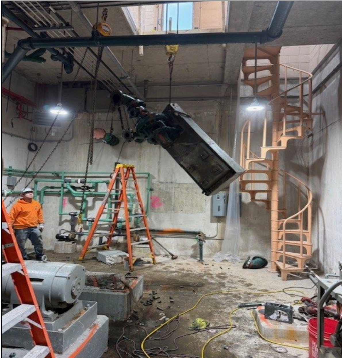
Figure 4 – Hoisting Old Equipment from Martin Basement Pipe Gallery
