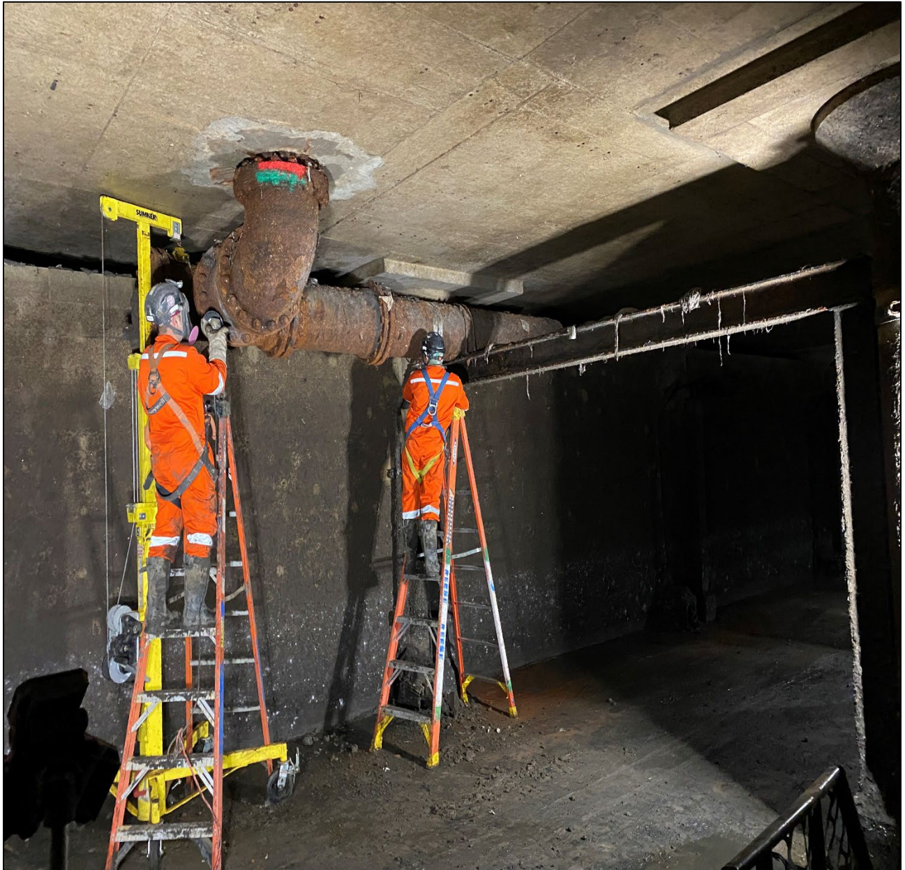
Figure 5 – Cutting Existing Flushing Pipe in Martin RTB
