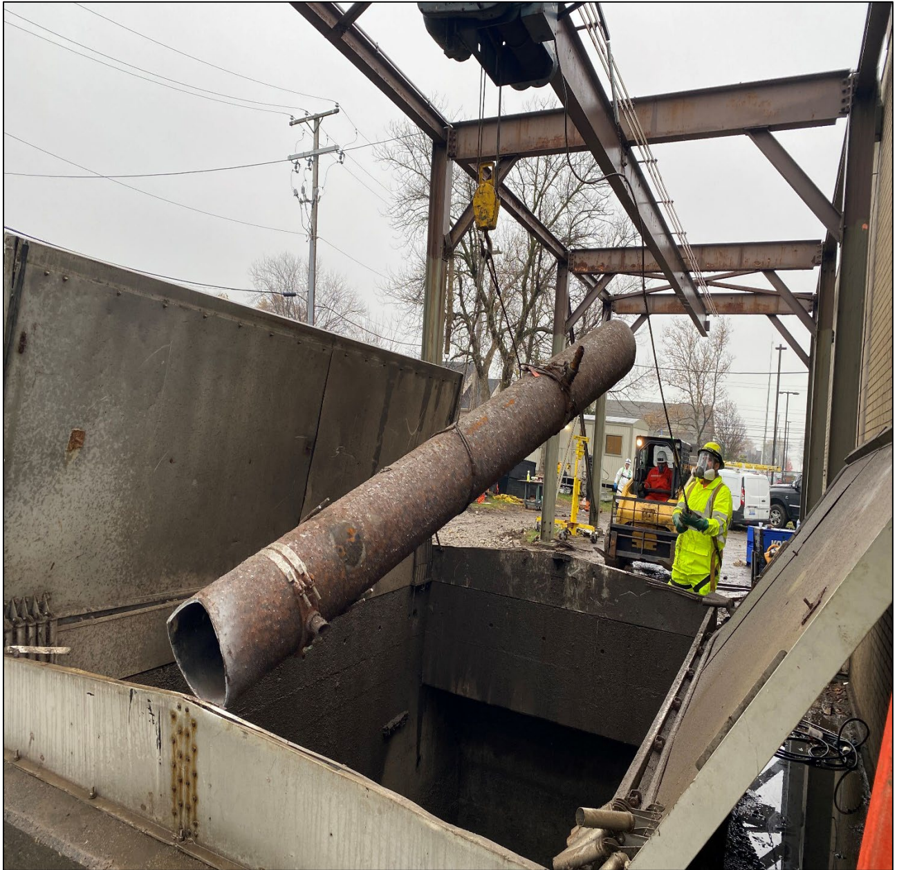
Figure 8 – Hoisting Flushing Pipe at Martin RTB Access Hatch
