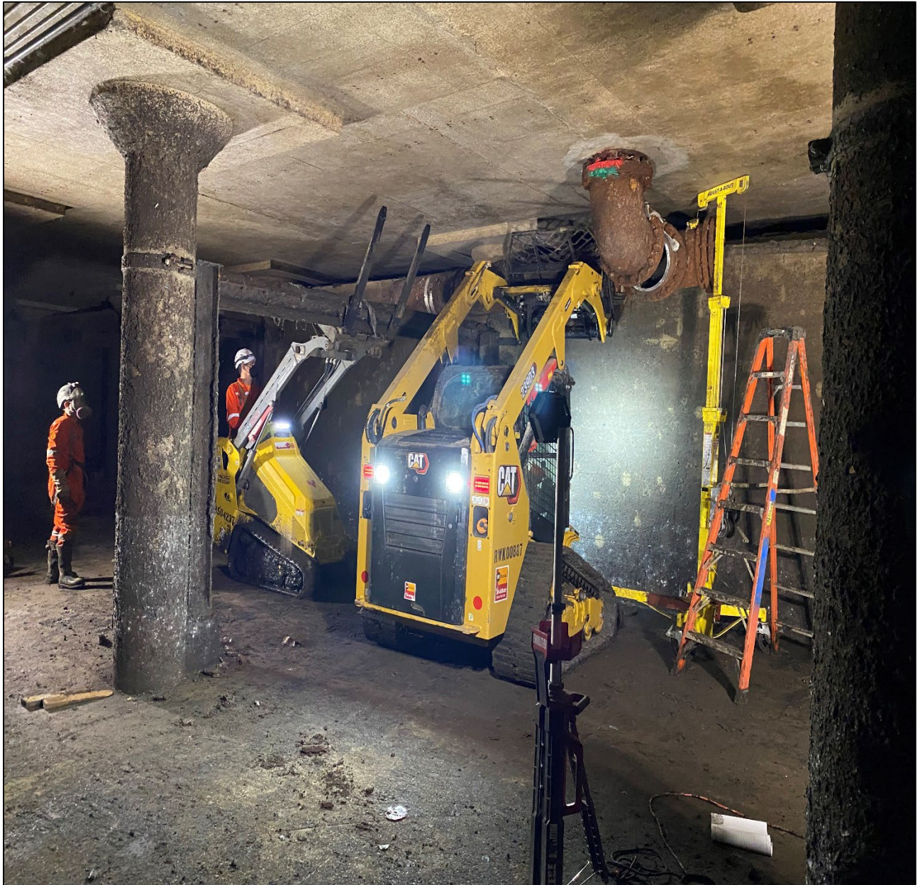
Figure 6 – Removing Existing Flushing Pipe in Martin RTB
