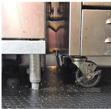
Floor mounted equipment elevated on 6-inch legs or on castors to move for cleaning.
