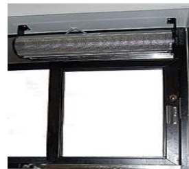
Air curtain over pass through window
