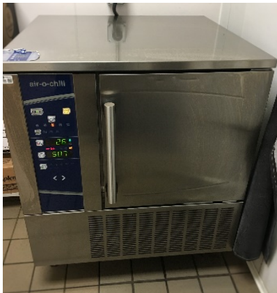
Exterior of Blast Chiller
