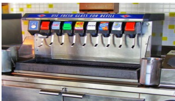
Equipment Sealed to Counter Top
