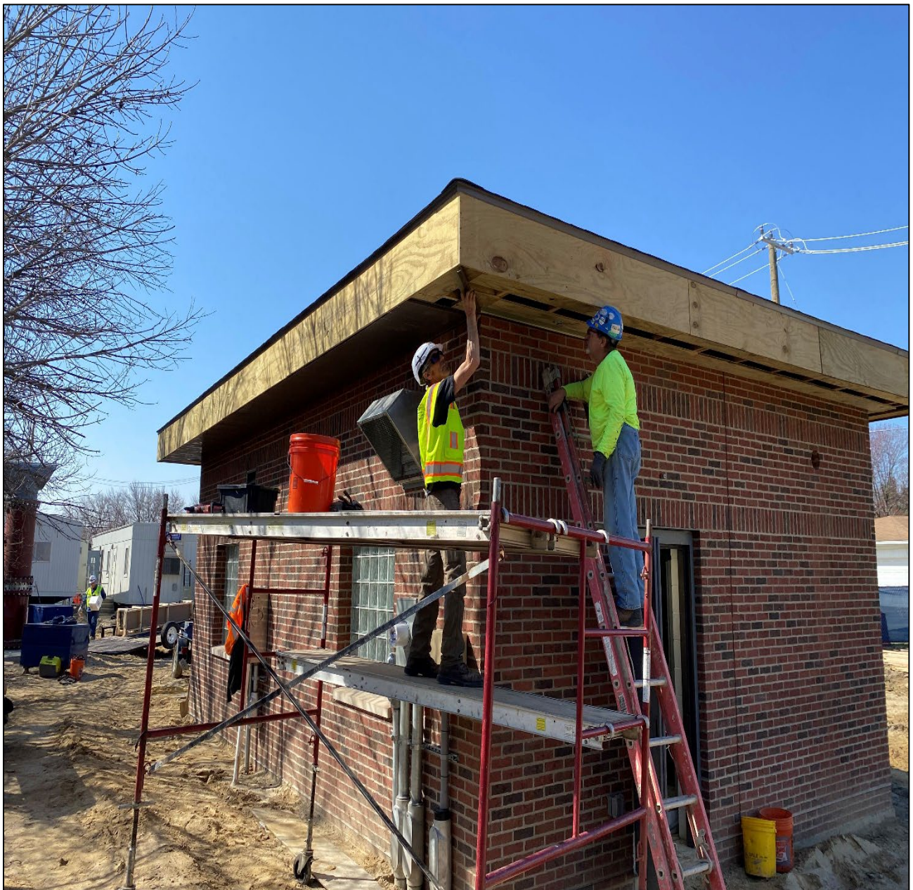
Figure 7 - Installing Exterior Finishes to Control Bldg. @ Beaconsfield Site
