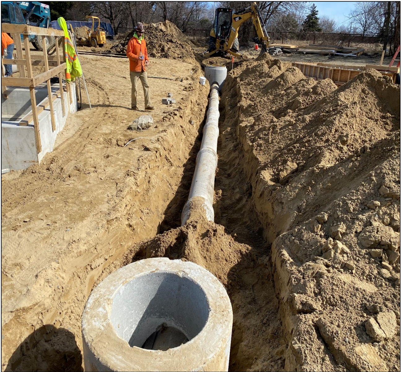
Figure 1 – Placing Concrete Storm Pipe @ Beaconsfield Rd.
