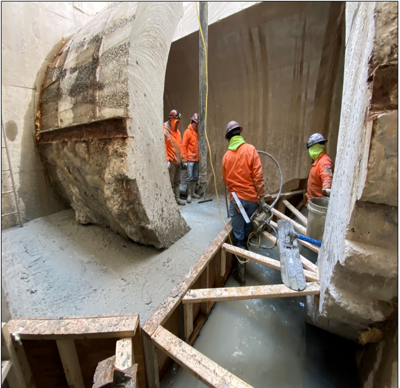
Figure 9 – Placing Concrete Bench @ Beaconsfield 11.5 FT Tunnel
