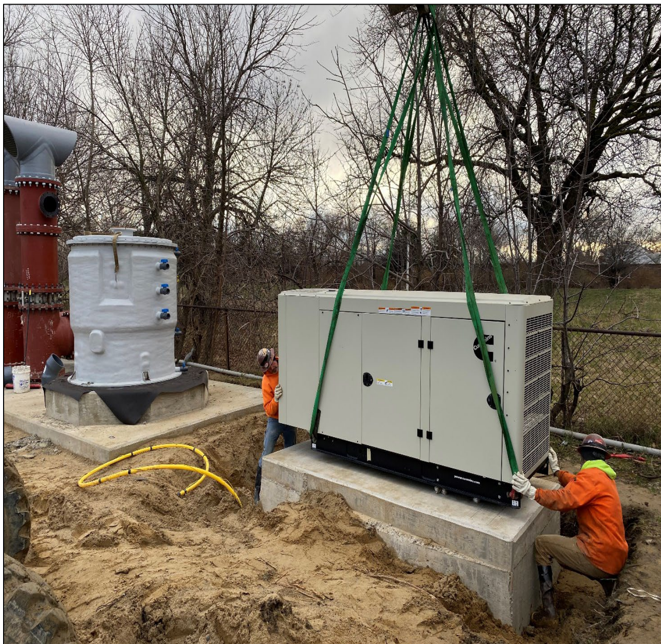
Figure 5 – Placing Backup Generator @ Beaconsfield Site
