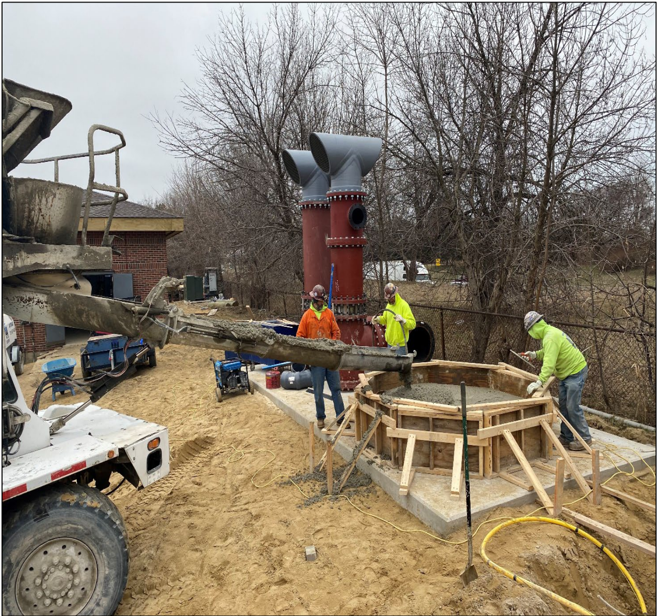
Figure 2 – Placing Concrete Media Canister Pad @ Beaconsfield Site
