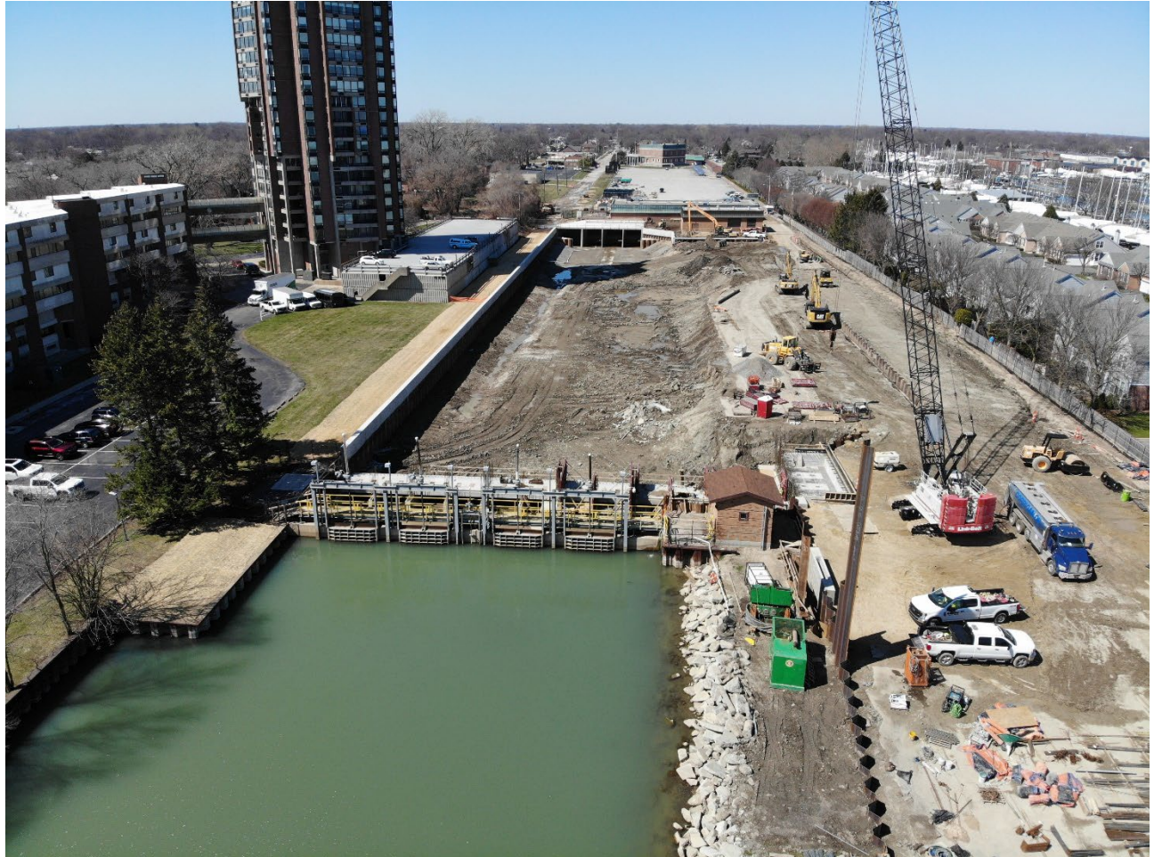
Figure 24 – Drone Aerial at 100 FT Facing West (03/28/24)
