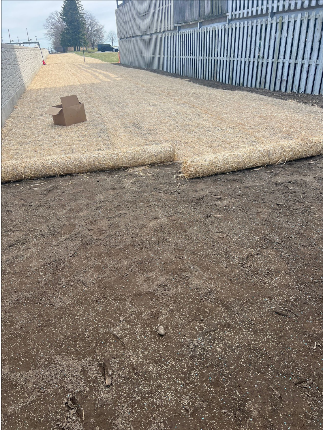
Figure 18 – Southside restoration along parking structure
