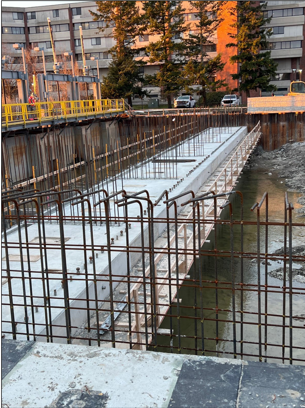
Figure 13 – Gate Slab pour completed and stripped
