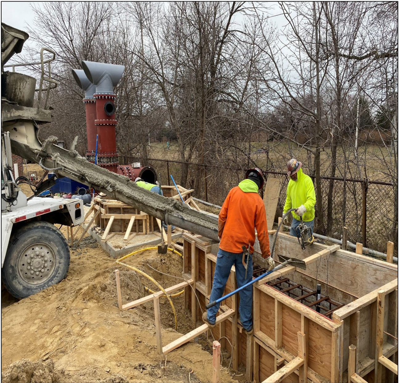
Figure 4 – Pouring Concrete Generator Pad @ Beaconsfield Site
