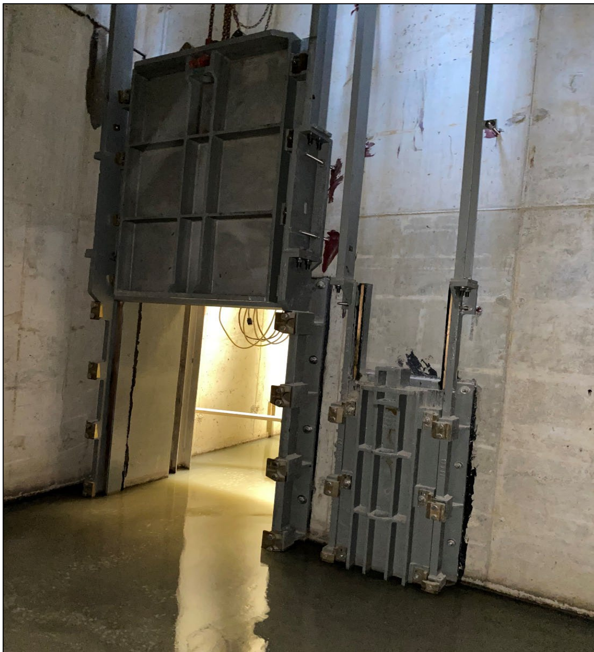
Figure 6 – Installed Sluice Gates for Tunnel Bypass @ Beaconsfield 11.5 FT Tunnel
