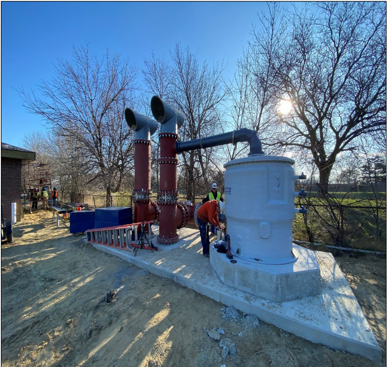
Figure 3 – Installing Odor Control Media Tank @ Beaconsfield Site
