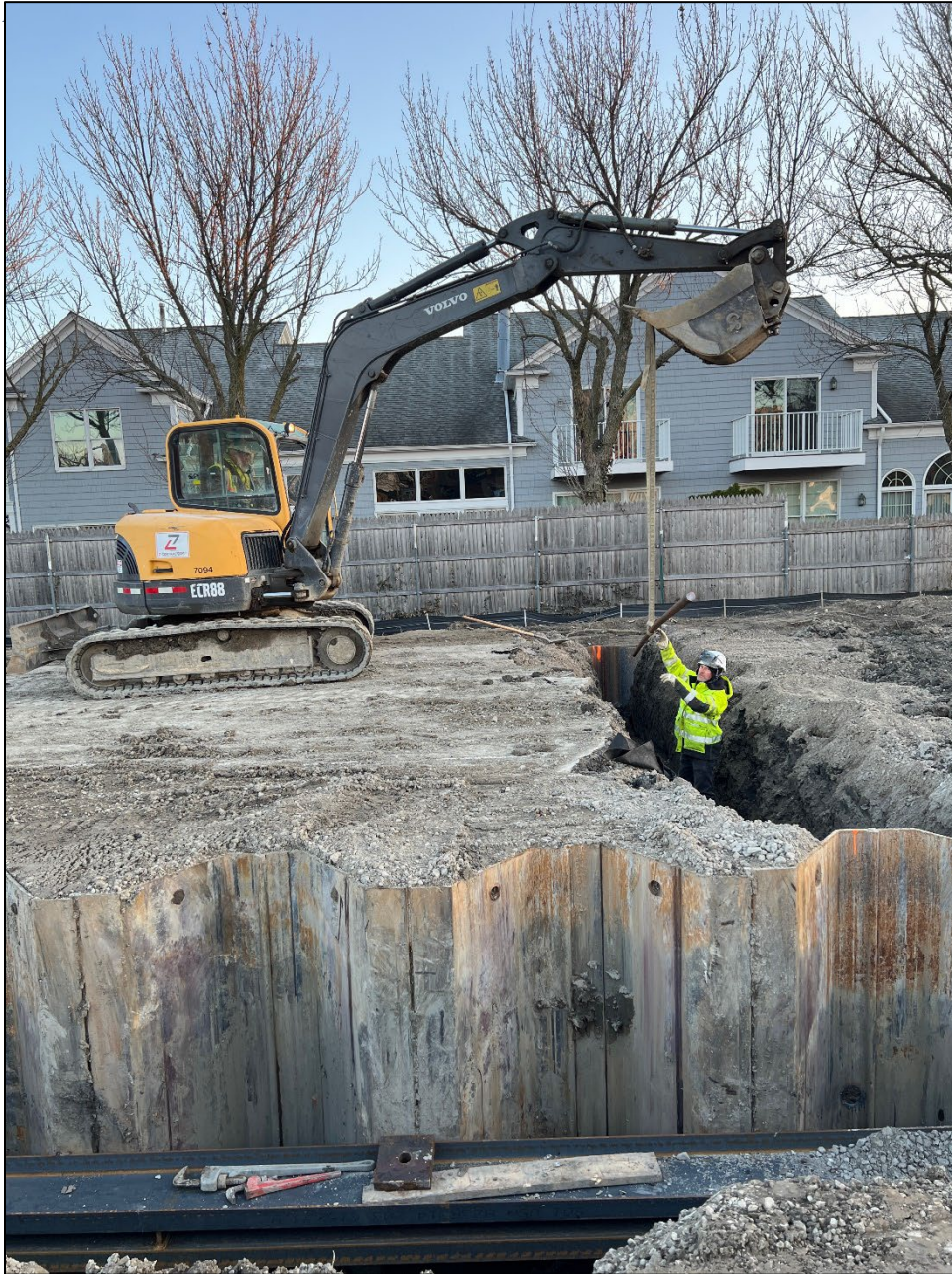
Figure 16 – Walers and Tieback installation
