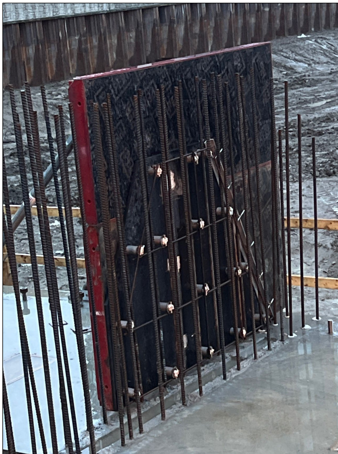
Figure 20 – Abutment Plate assembly installed (future weir gate location)
