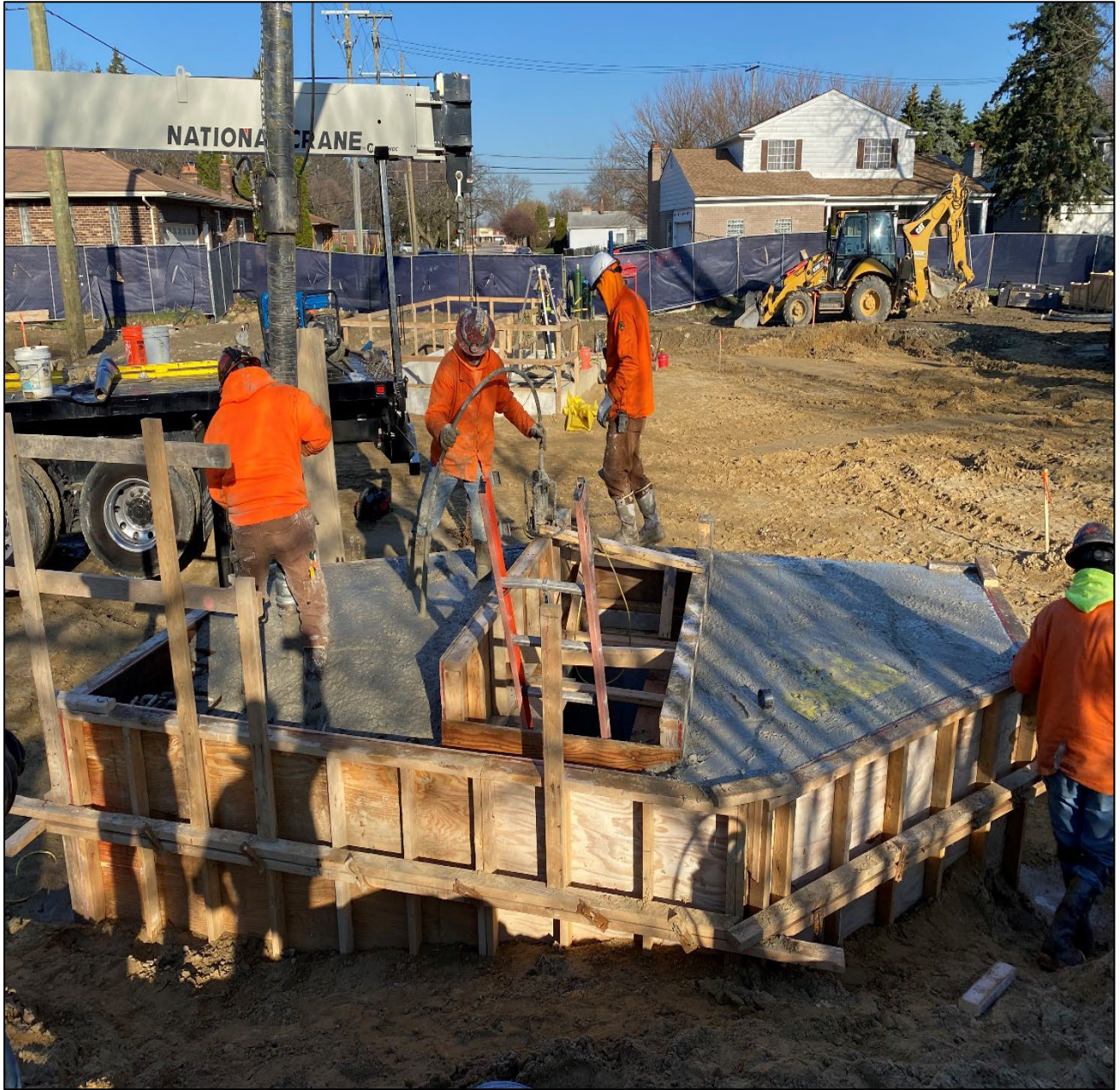
Figure 10 – Placing East Access Vault Roof Conc. @ Beaconsfield Site
