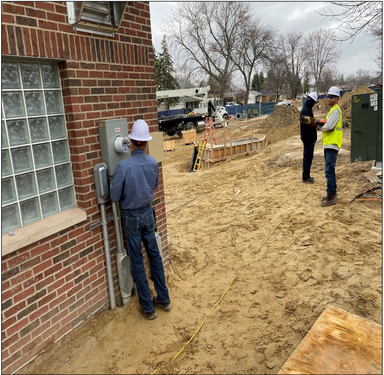
Figure 8 – DTE Installing Meter & Powering Control Bldg. @ Beaconsfield Site
