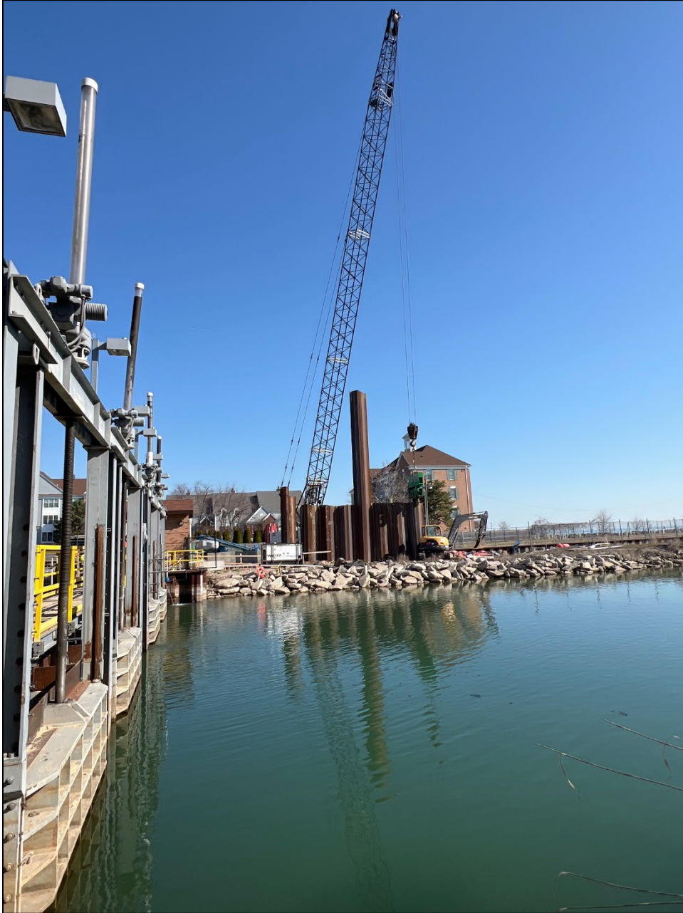
Figure 15 – Last line of new sheeting tied into existing Boat Ramp sheeting
