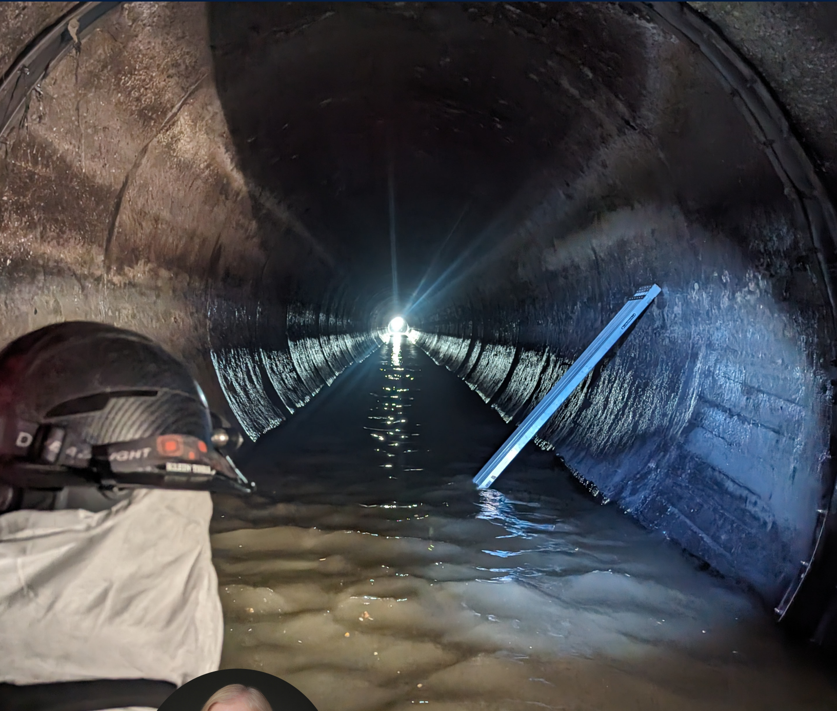
Pictured: "Light at the end of the tunnel" - watching the first piece of HOBAS pipe being installed down the pipe at the Segment 5 Sewer Rehabilitation Project
