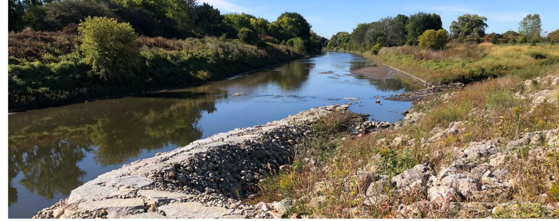
The Sterling Relief and Red Run Drain Habitat Restoration and Trail Connector Project incorporated green infrastructure to stabilize the banks, reduce erosion and create habitat. Due to the flashiness, the water flows, velocity, and high-water elevation can change quickly. The project protects a closed landfill while managing channel-forming flows and providing protection from the fluctuation of flows.
