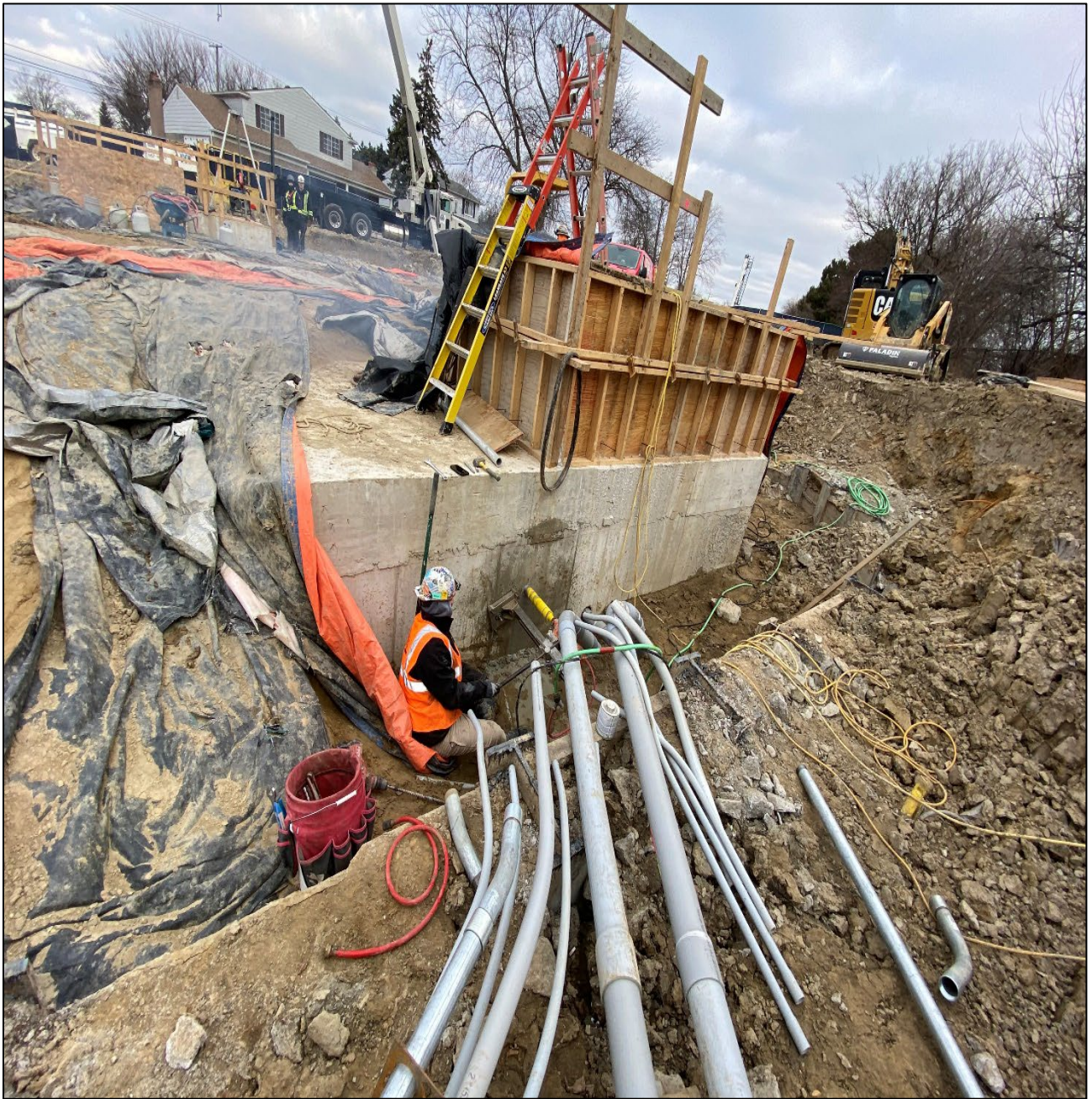
Figure 3 – Installing Conduit for Controls to Access Vault @ Beaconsfield Rd.
