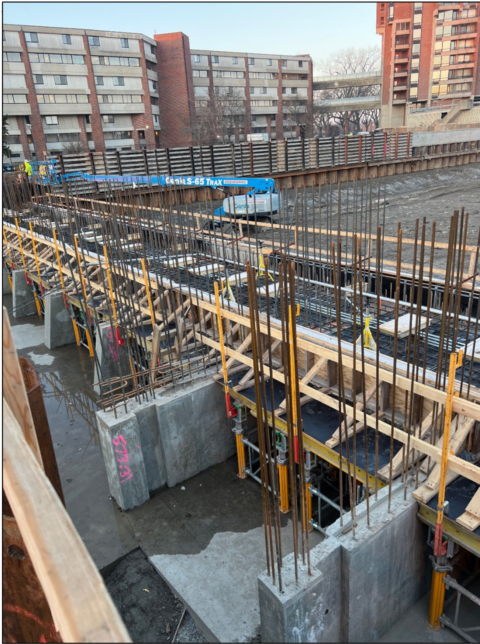
Figure 19 – Gate Structure formwork and reinforcement
