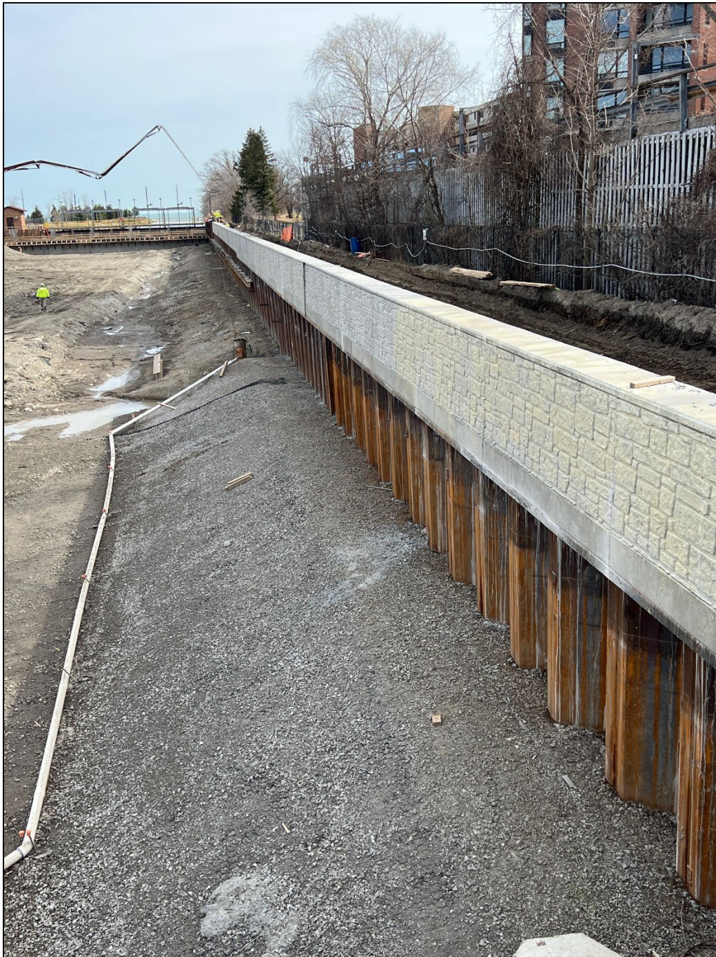
Figure 17 – South Side concrete cap finished
