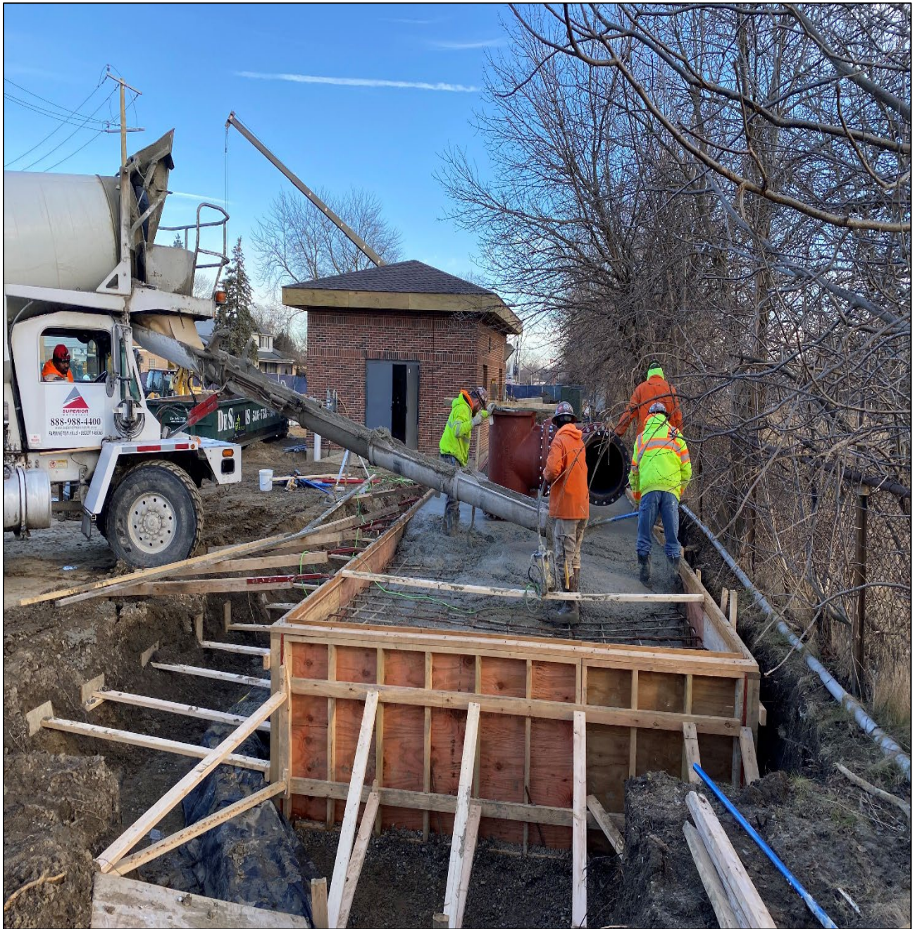
Figure 1 – Placing Conc. Pad for Odor Control Equipment @ Beaconsfield Rd.
