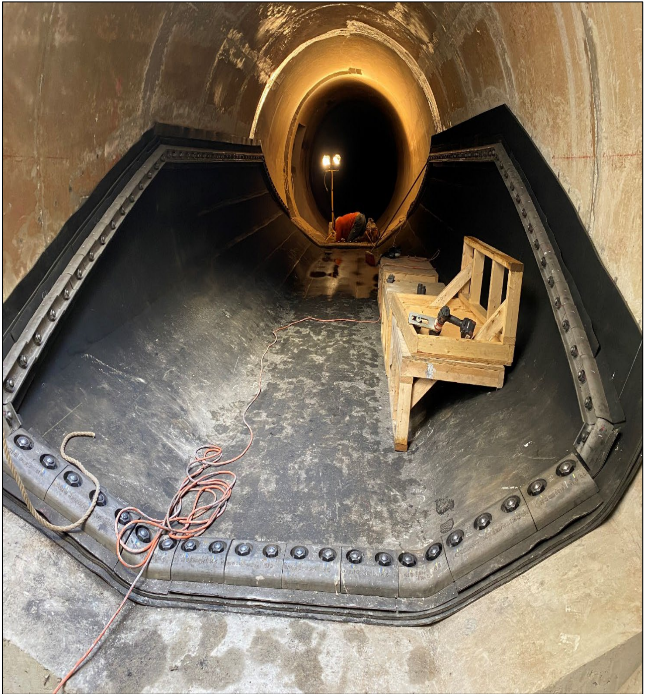
Figure 11 – Installed Inflatable Sewer Gate @ 11.5FT Tunnel
