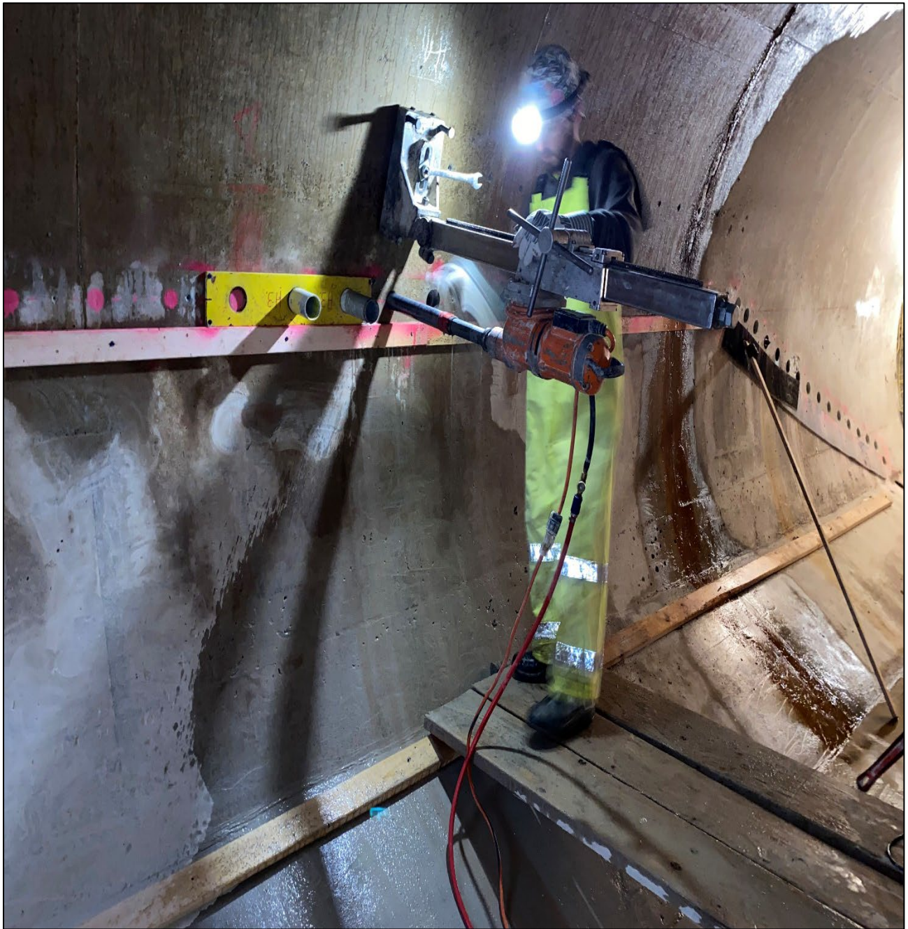
Figure 6 – Coring Conc. for Inflatable Dam Anchors @ Beaconsfield 11.5 FT Tunnel
