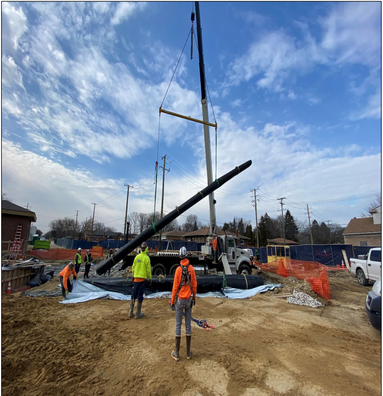
Figure 8 – Hoisting Membranes into 11.5 FT Tunnel @ Beaconsfield Rd.
