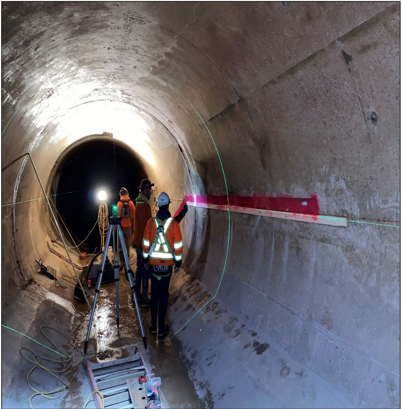
Figure 5 – Setting Inflatable Dam Anchor Template @ Beaconsfield 11.5 FT Tunnel
