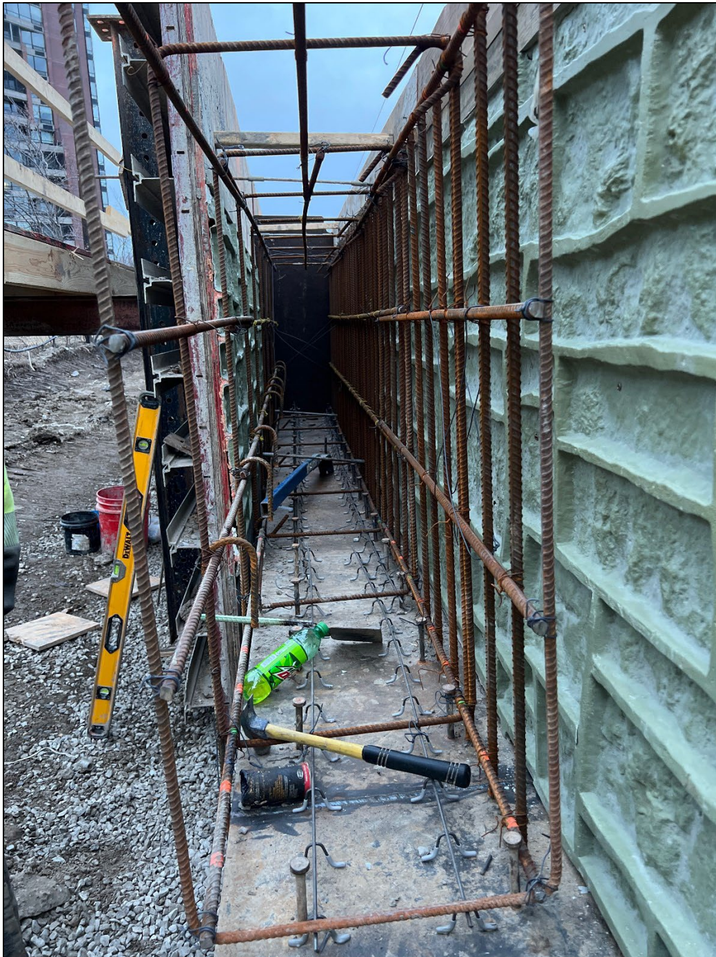
Figure 15 – South Side concrete cap reinforcement
