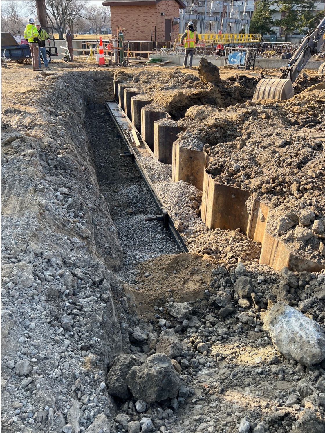
Figure 21 – Tie-back wall, walers, and tie-rods
