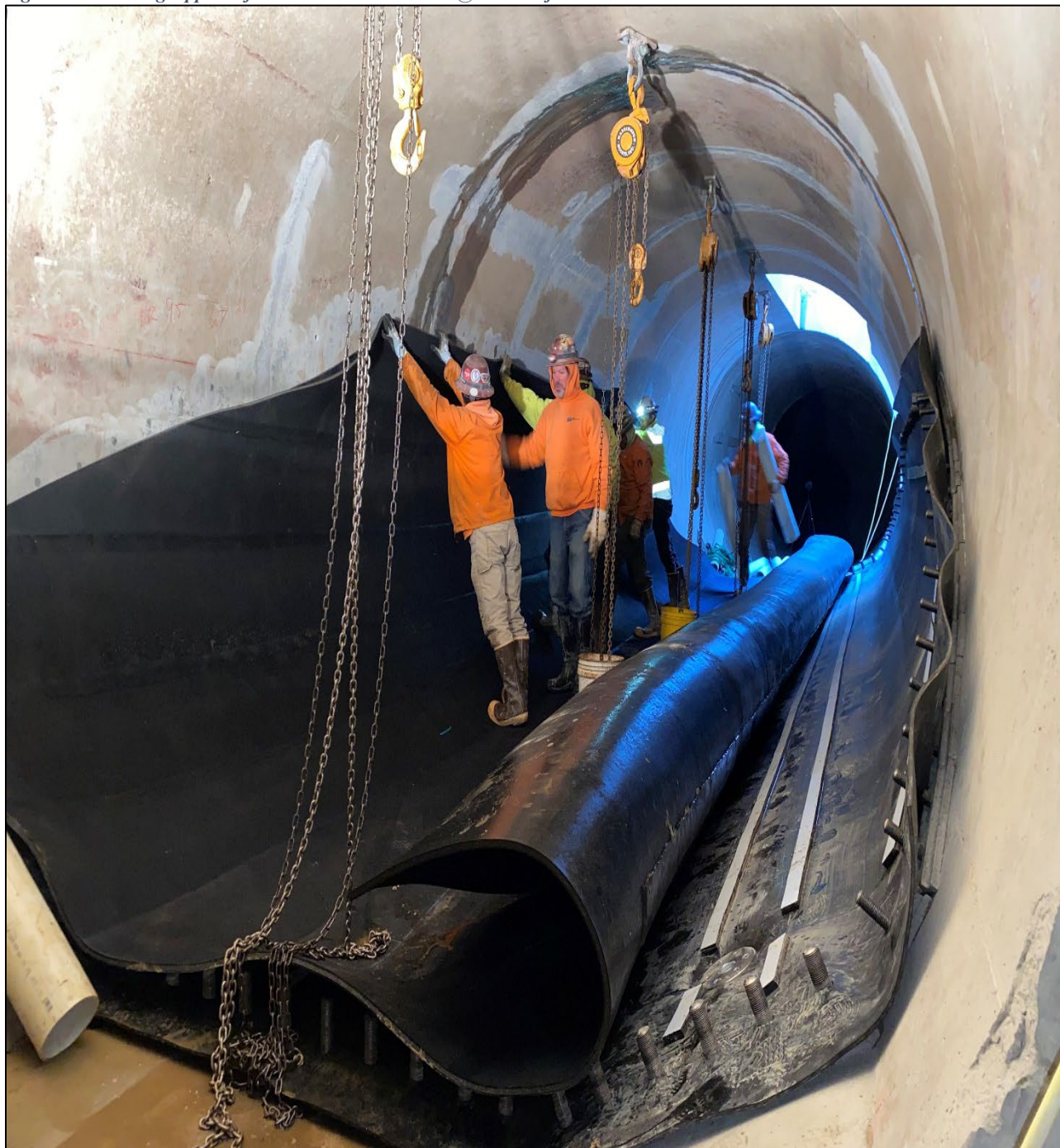
Figure 10 – Placing Upper Inflatable Dam Membrane @ Beaconsfield 11.5 FT Tunnel
