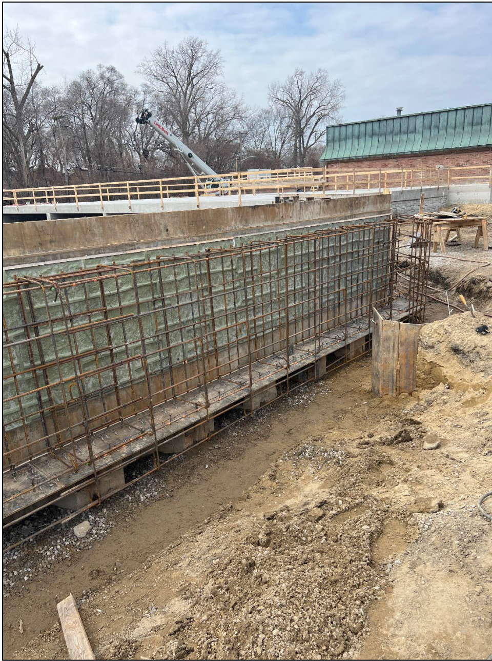
Figure 18 – North Side concrete cap forms
