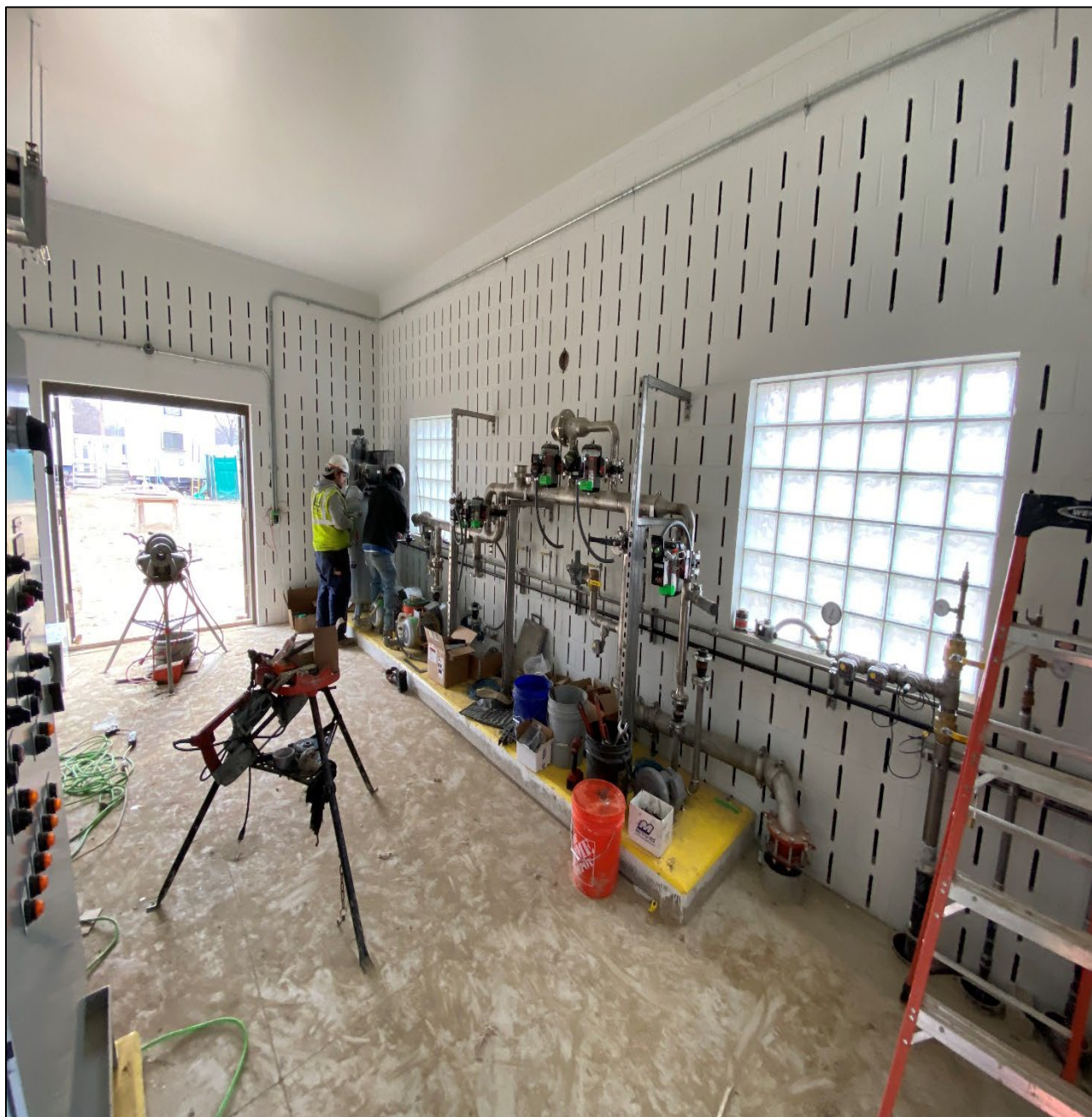
Figure 4 – Installing Process Equipment for Inflatable Dam @ Control Building
