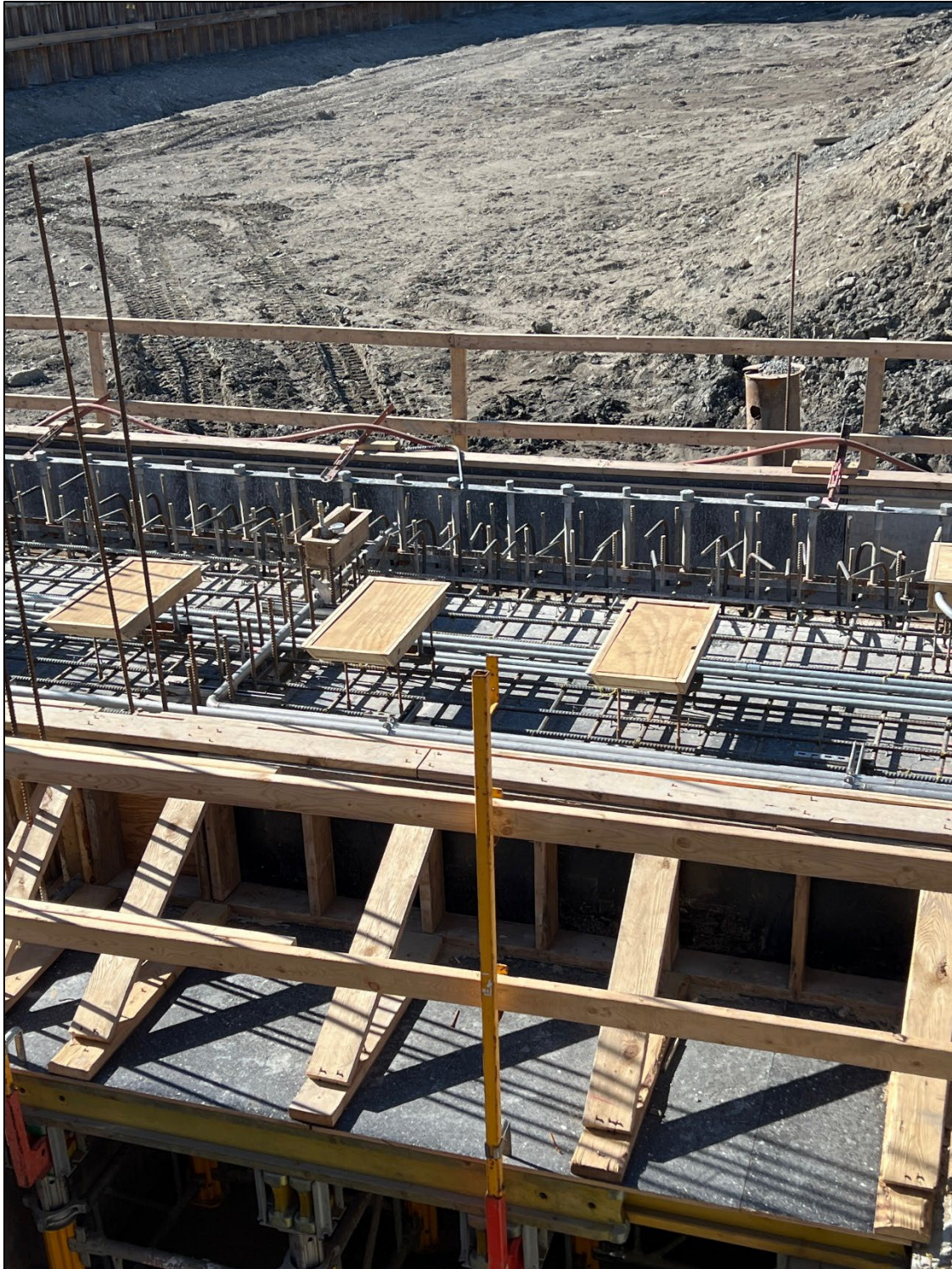
Figure 20 – Gate Structure conduits, air lines, and boxouts
