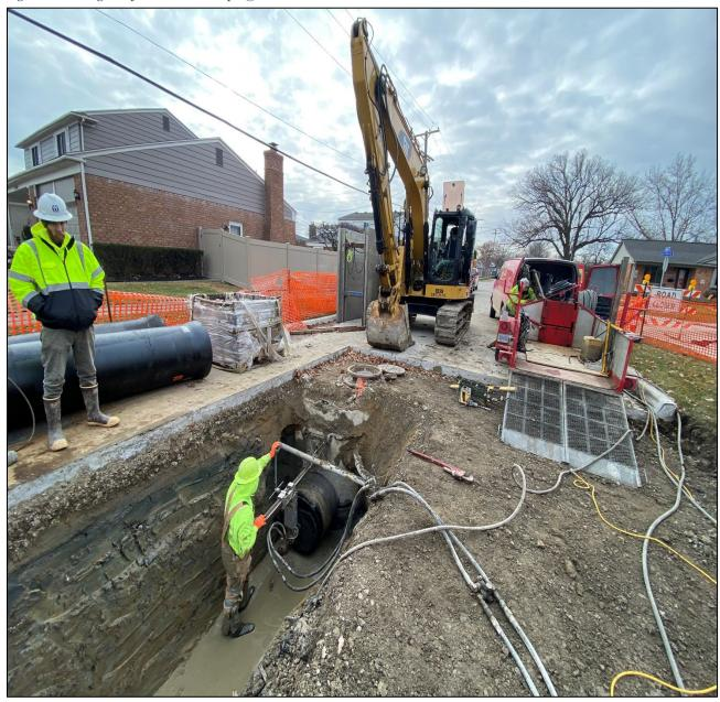
Figure 10 –Installing 24in Ventilation Pipe @ Malvern Street
