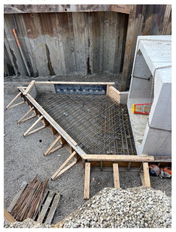
Figure 19 – Repurposed 9-Mile Drain into Storm Sewer Discharge Chambers with Hatches, stoplog grooves, etc.
