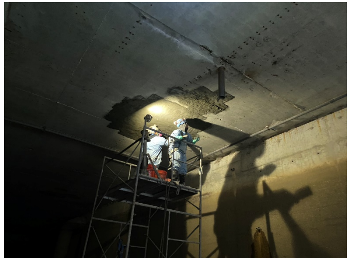
Figure 2 – Aeration Chamber – Concrete ceiling repairs
