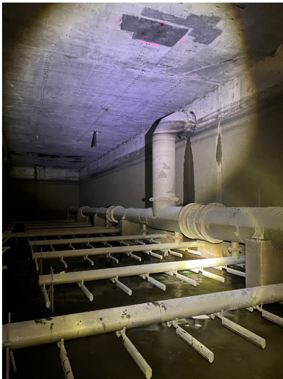
Figure 3 – Aeration Chamber – Concrete ceiling repairs
