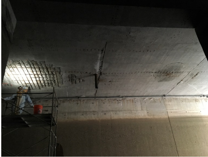
Figure 1 – Aeration Chamber – Demo / Prep for ceiling repairs
