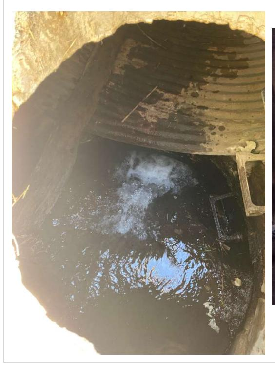
Appears to be failing Between the CMP and The  $30^{\circ}$  RCP
