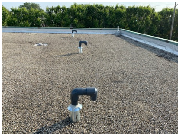
Figure 2 – Installed new chlorine storage tank roof vents
