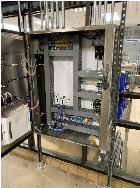
Figure 1 – Removed & Replaced faulty VFD #4
