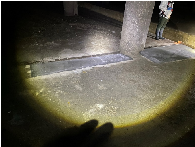
Figure 5 – Concrete floor repair
