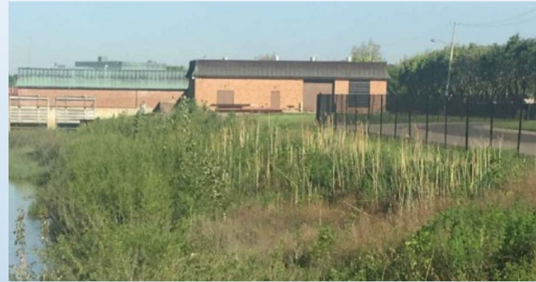
Existing Chapaton Treatment Canal – North Bank
