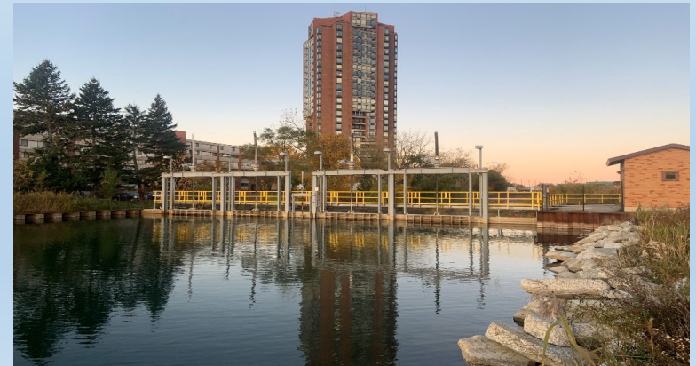
Existing Outfall Gates – Lake Level 576.5+
