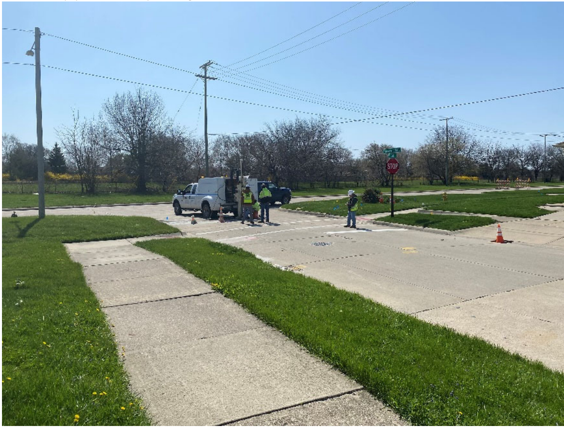
Photos of pipe location probing at Beaconsfield & Oak on 04.28.22
