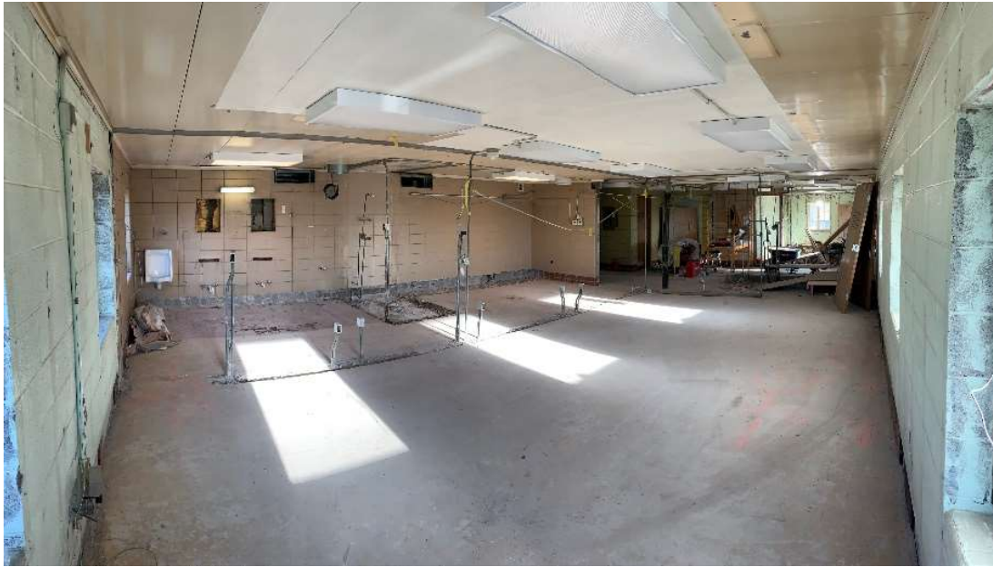
Figure 6 – All existing walls demolished and removed – Future Kitchen Area
