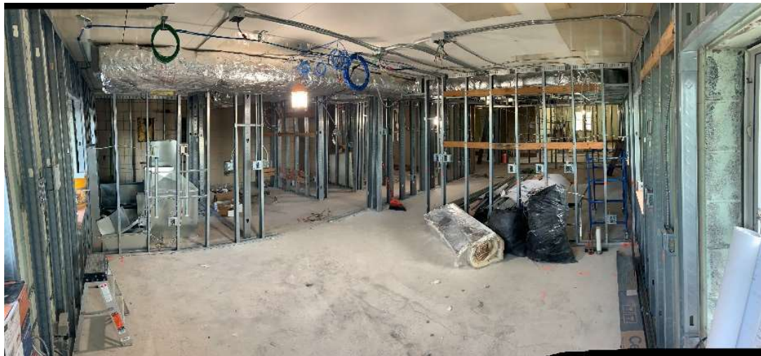
Figure 7 – New framing, electrical, plumbing, and HVAC – Future Kitchen Area
