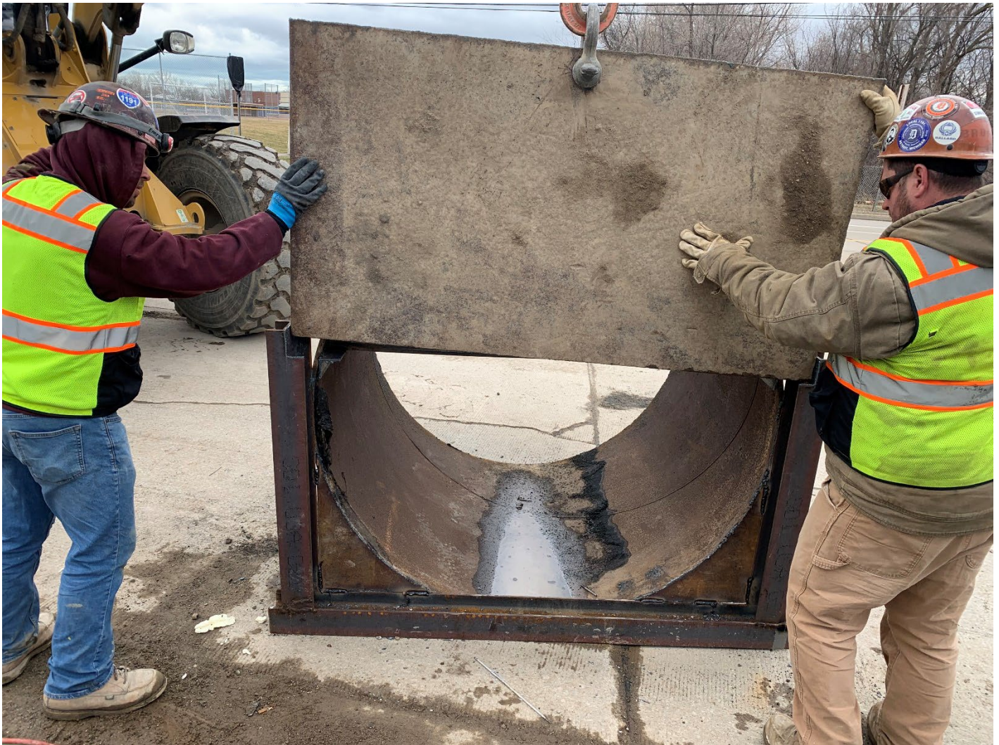
Figure 11 – Temporary Weir at MH-01 for Annulus Grouting of 54-inch HOBAS
