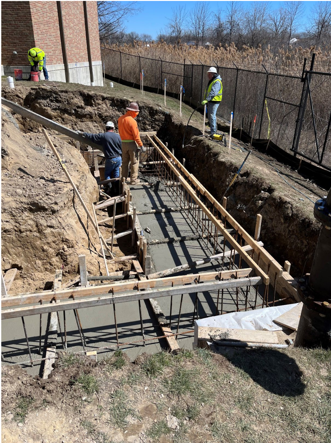
Figure 15 – Clintondale PS Foundation Work
