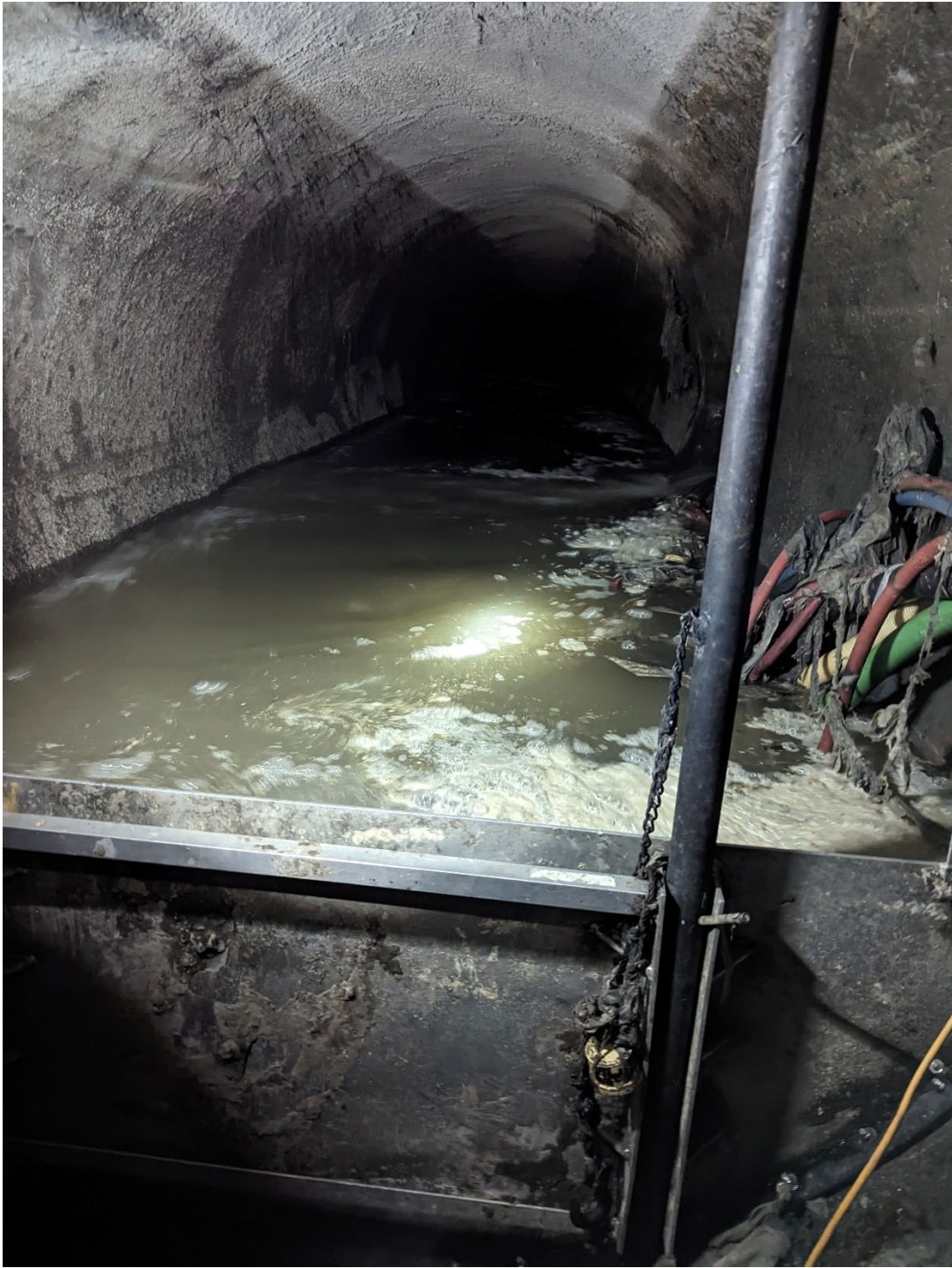
Figure 4 – Section of 8-foot Pipe that has been Spray-lined
