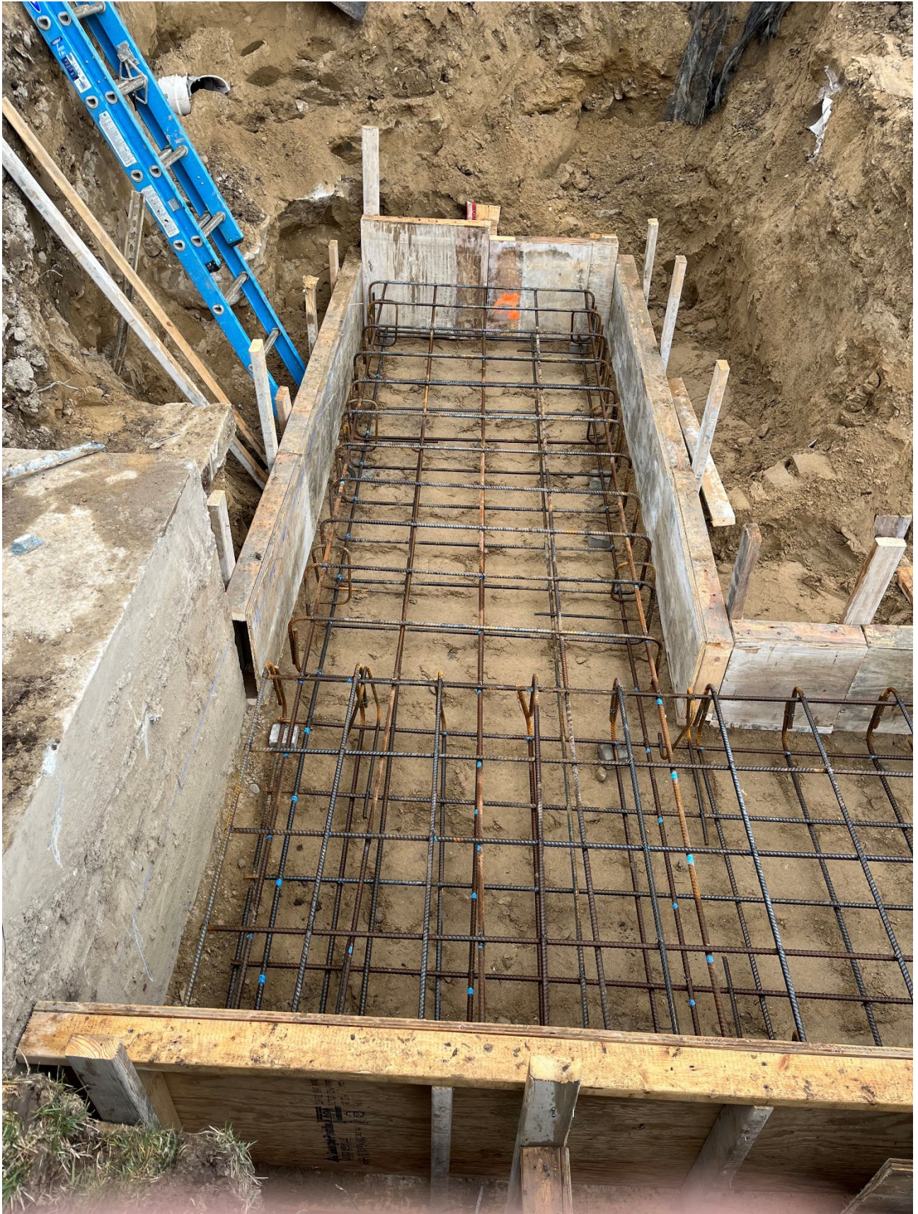
Figure 14 – Clintondale PS Foundation Work
