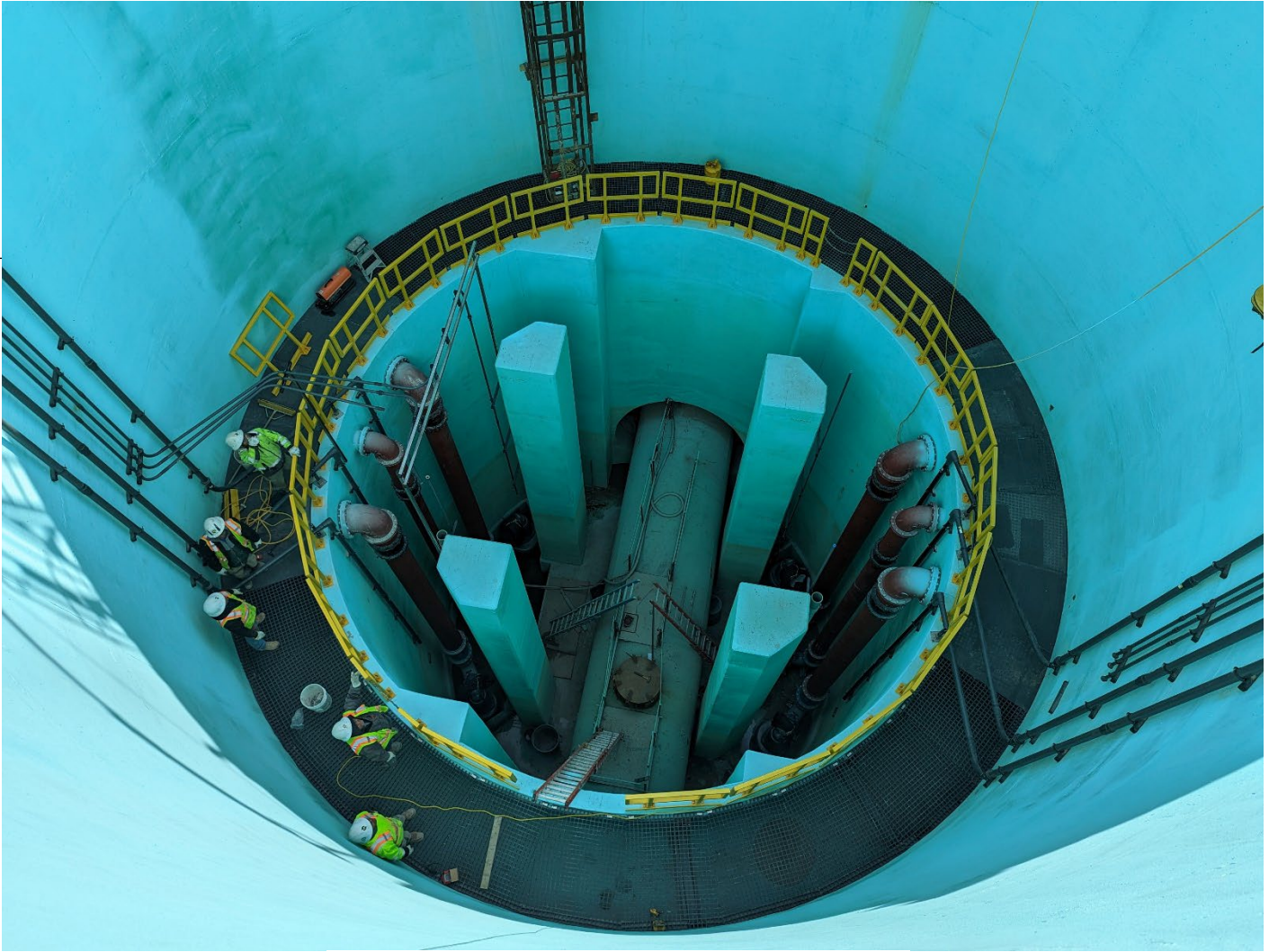
Figure 1 – CS-12 Structure – Perimeter Flume Grating Installed
