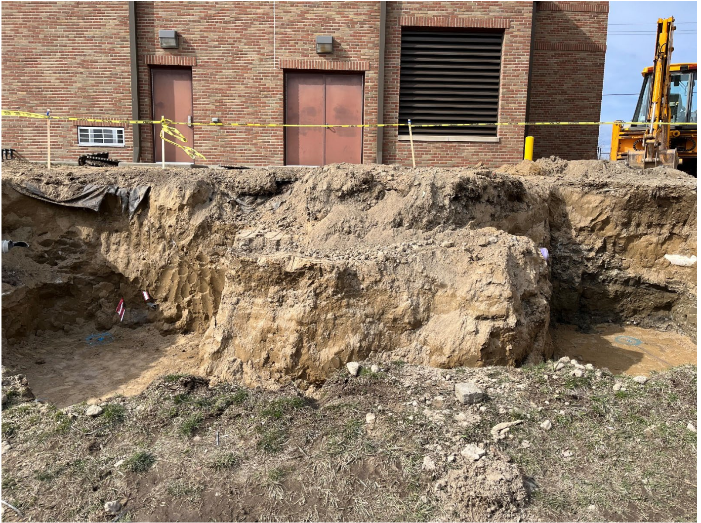
Figure 13 – Clintondale PS Foundation Excavation Work
