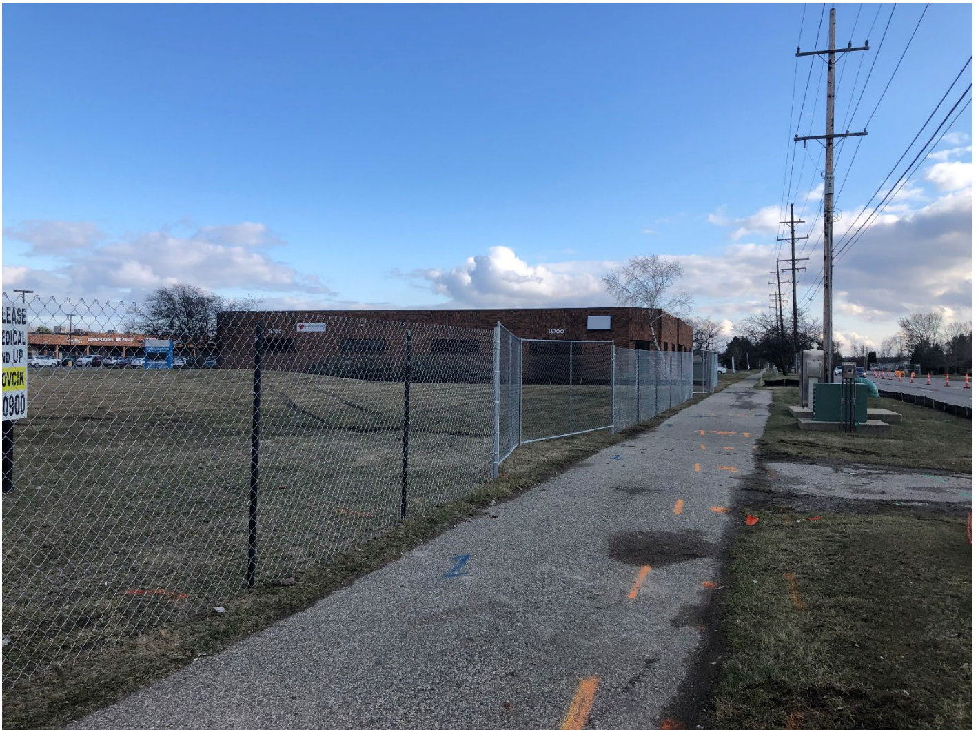
Figure 16 – 21 Mile & Garfield Temporary Construction Fence
