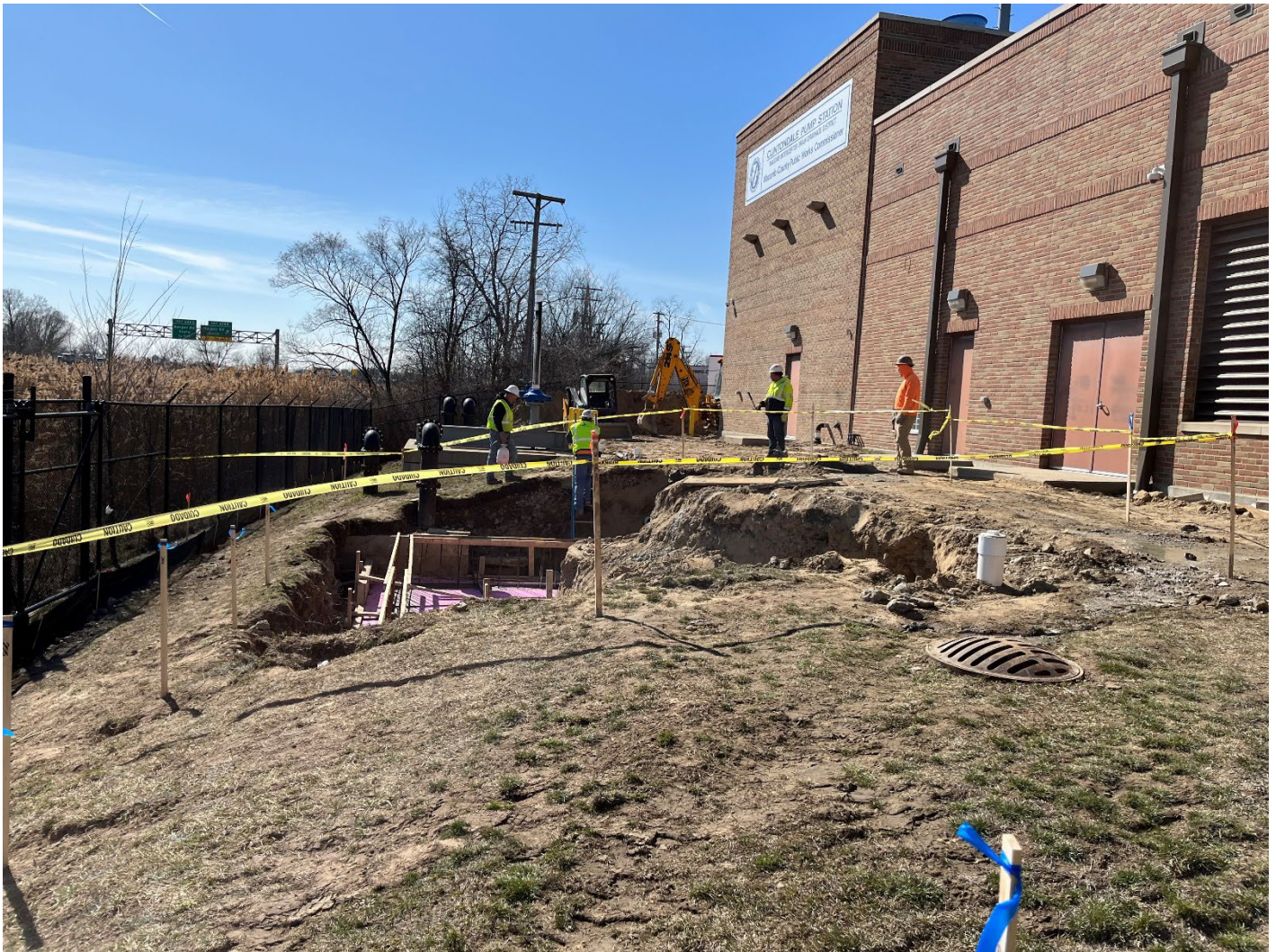
Figure 12 – Clintondale PS Foundation Work
