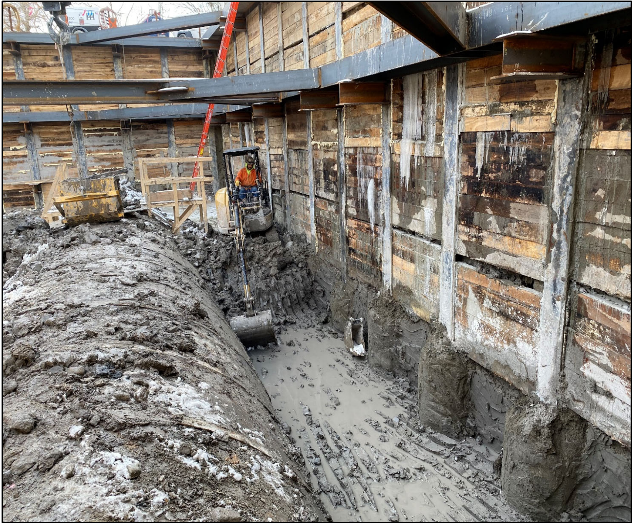
Figure 2 – Excavating South Side of 11.5FT Tunnel
