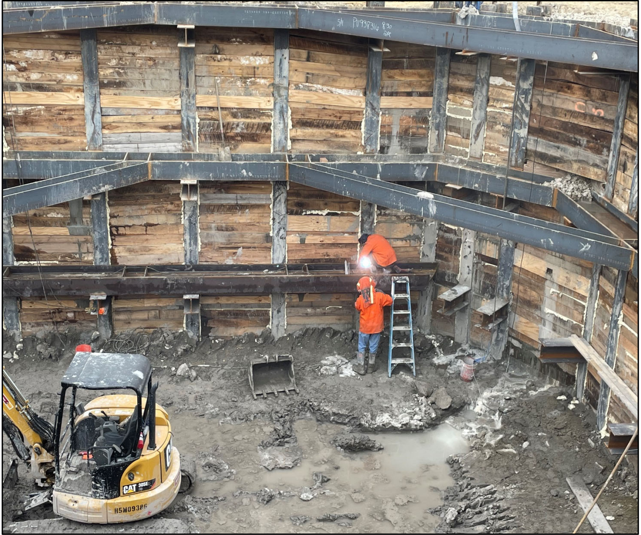
Figure 4 – Welding Lower Level Shaft Support I-Beams
