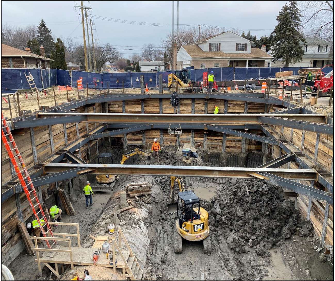
Figure 3 – Exposed Tunnel Excavated to Approx. 25FT
