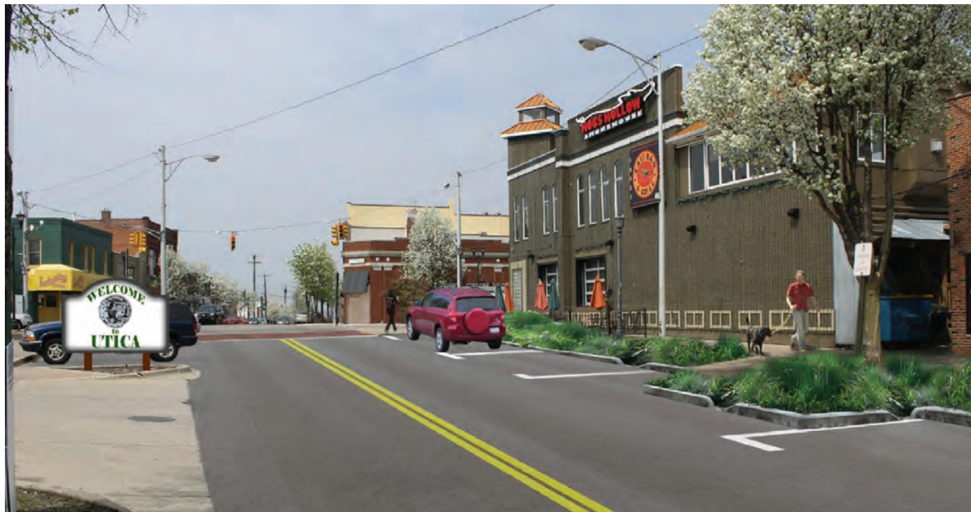
Bio-retention cells, as seen along Auburn Road, would result in at 84 percent reduction.
