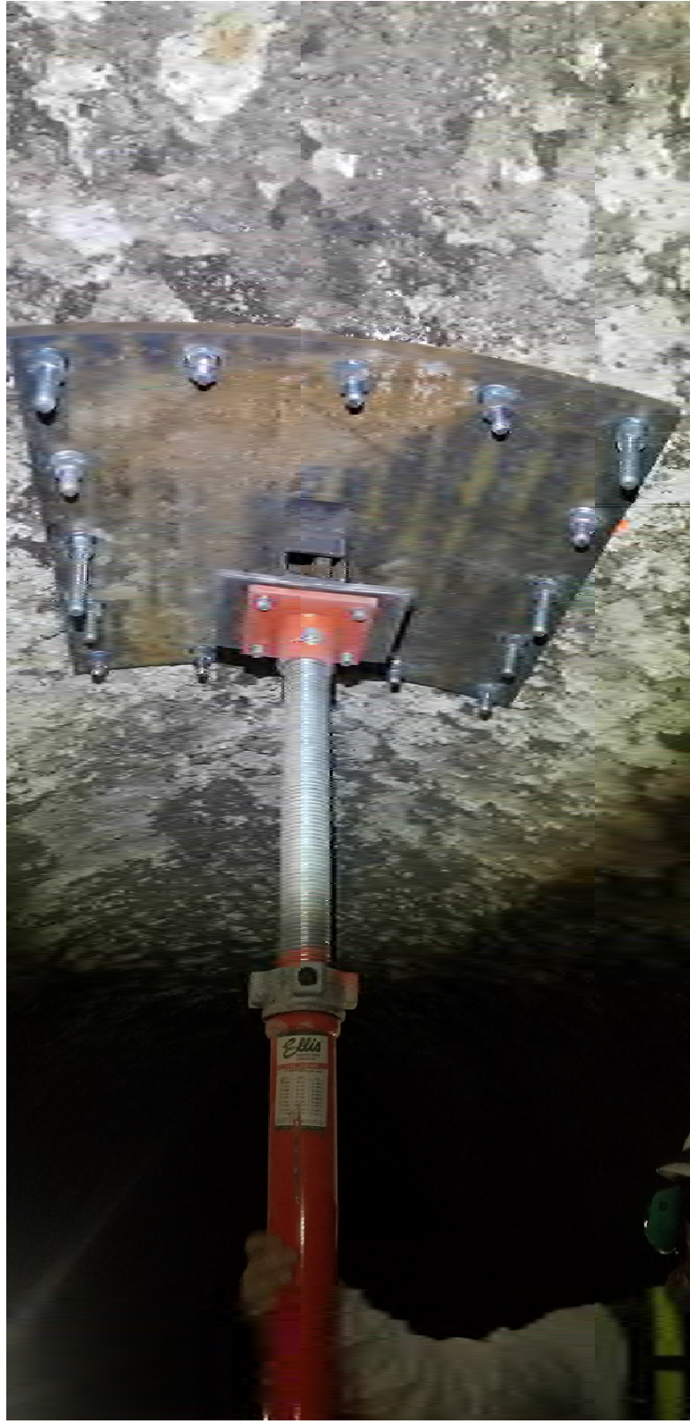
Figure 4 - Top Plate for Half-Height Bulkhead at MH-05
