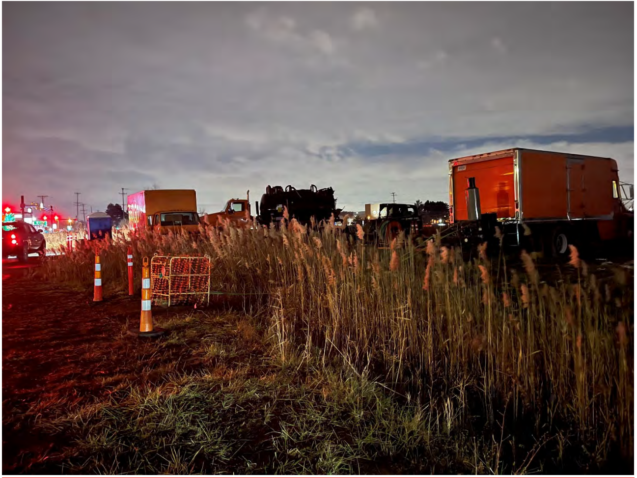
Figure 5 - Garfield Interceptor MH-19 Setup Near Hall Road
