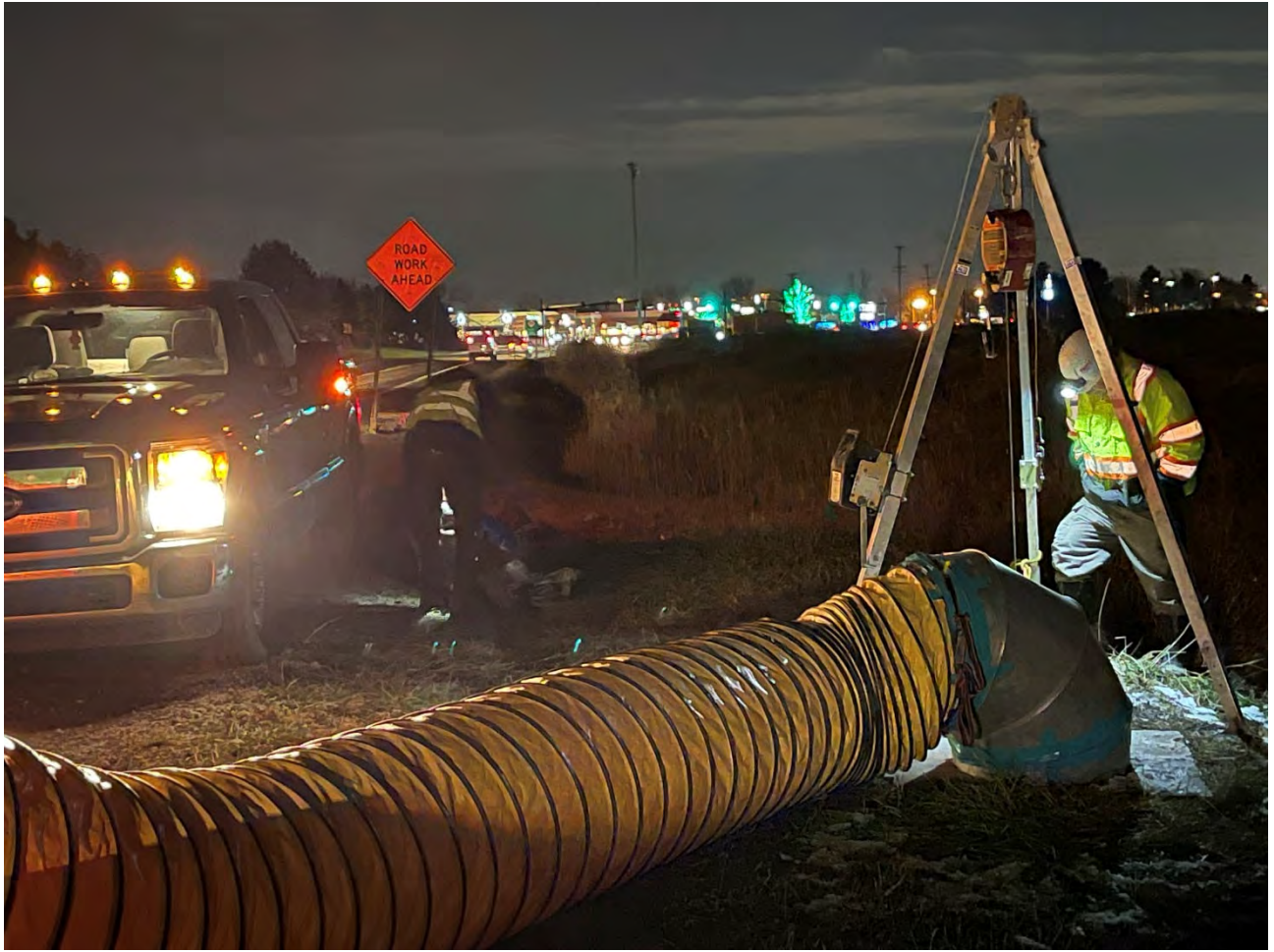
Figure 6 – Confined Space Entry & Ventilation Setup
