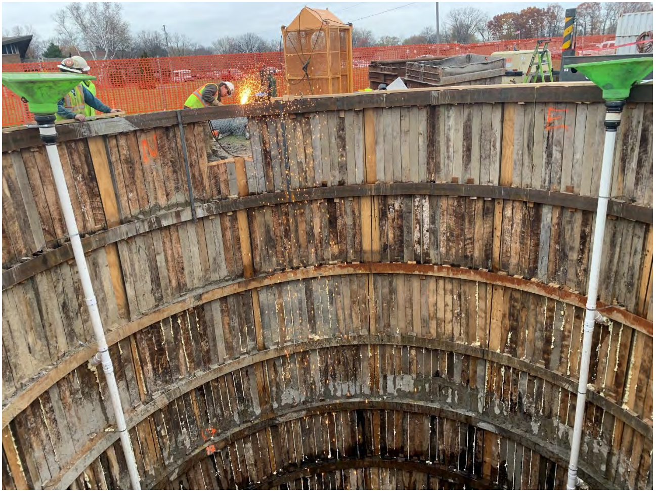
Figure 8 – Work on the Temporary Earth Retention System (TERS)
