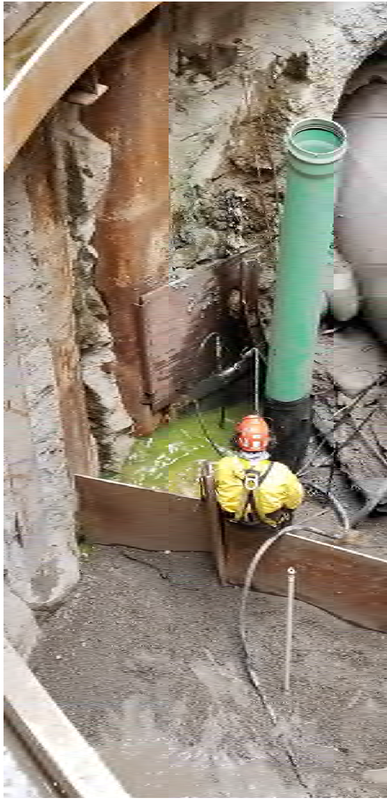
Figure 2 – Chemical Grouting at the Tunnel Eye
