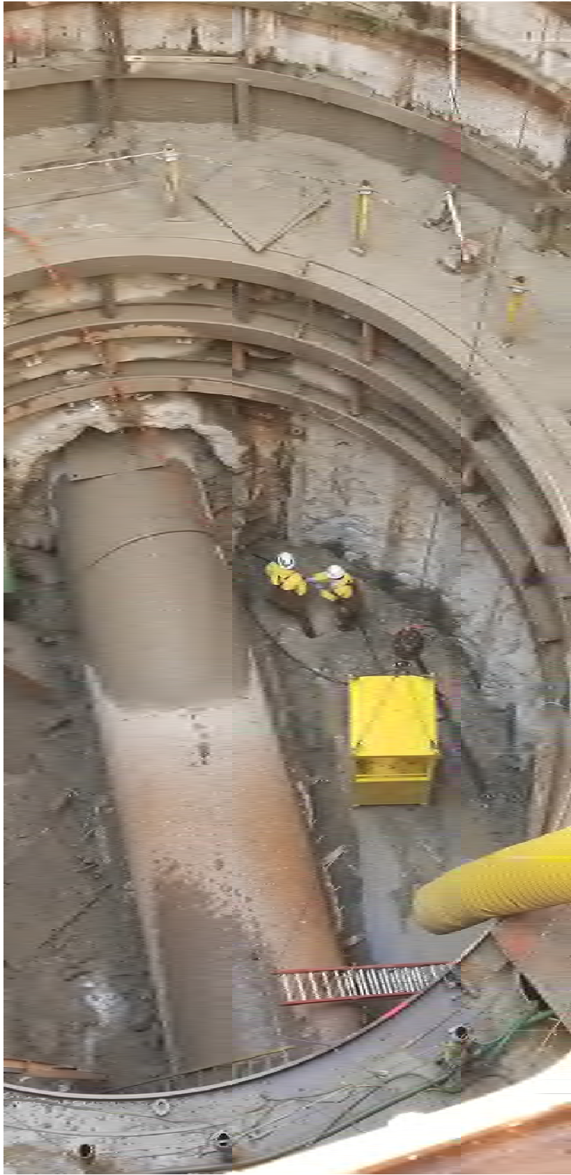
Figure 1 - Chemical Grouting at the Tunnel Eye
