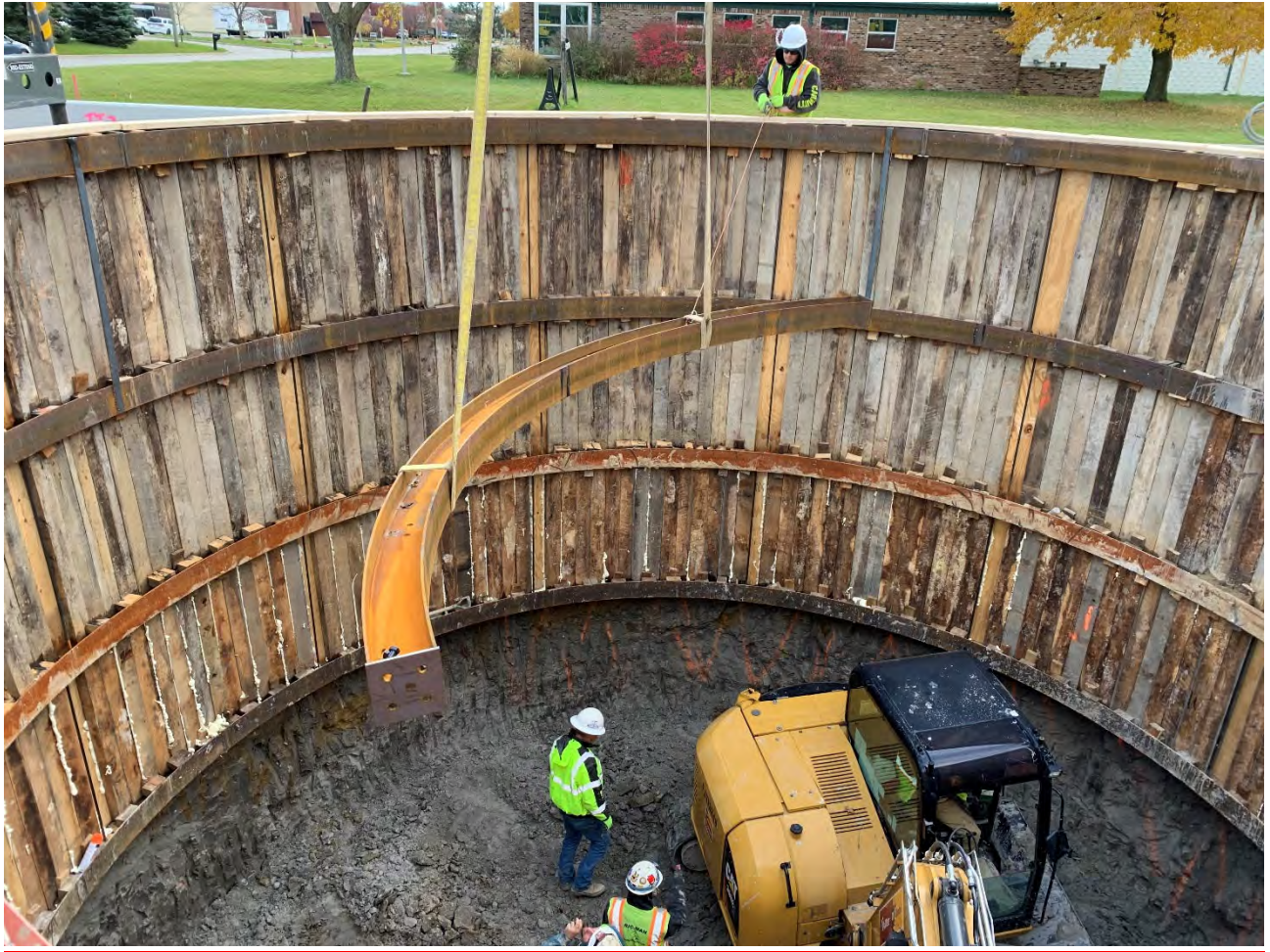
Figure 9 – Construction of the CS-13 TERS
