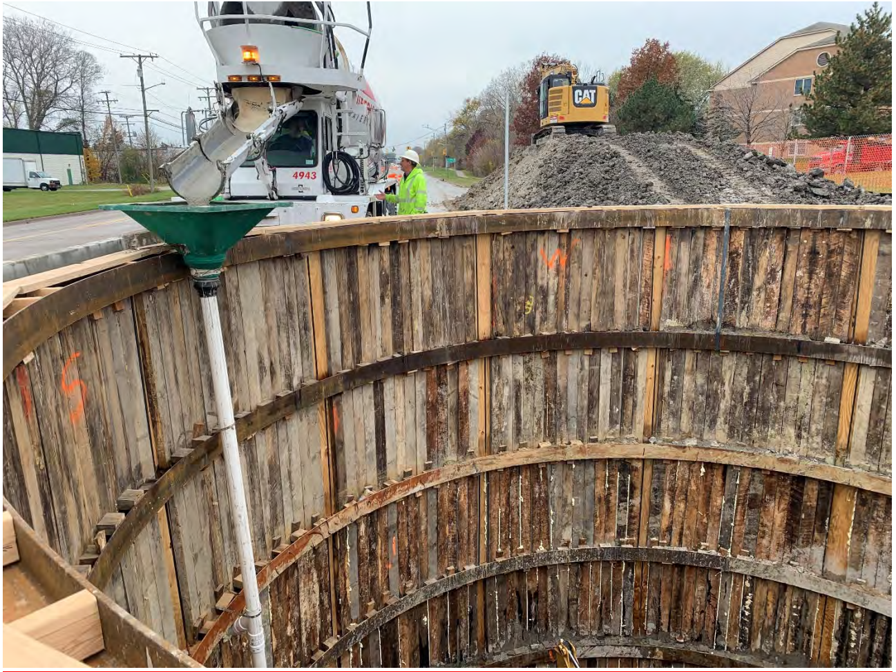
Figure 12 – Grout Placement Behind the TERS
