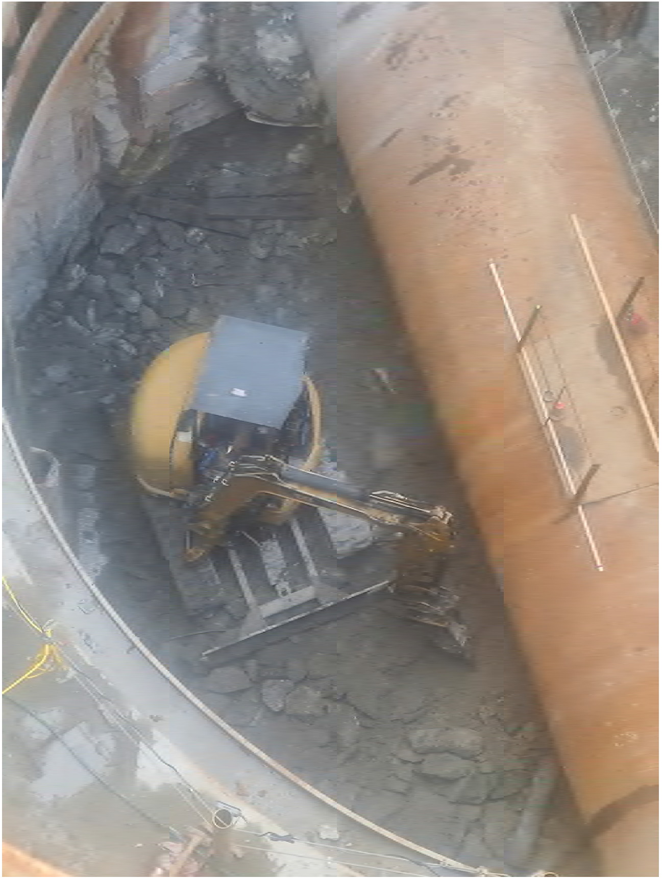
Figure 3 – Demolition of the existing Concrete Interceptor within the CS-12 Shaft
