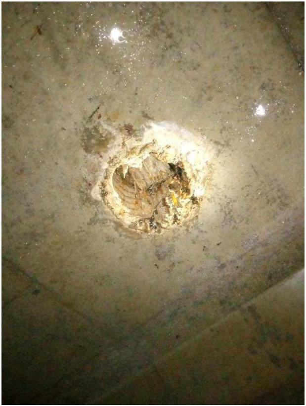
Figure 2 - Tap Prior to Repair
