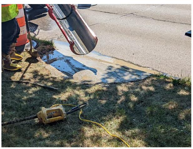
Figure 4 - Placement of Concrete Flowable Fill - Approximately 6 Yards
