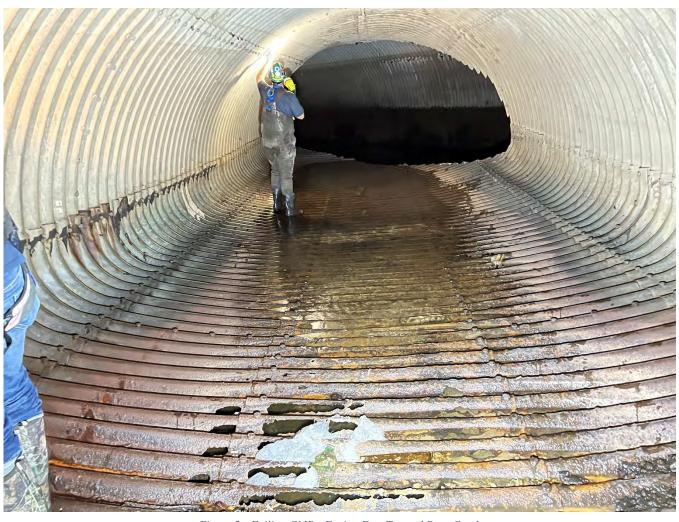
Figure 2 - Failing CMP - Facing East Toward Bear Creek
