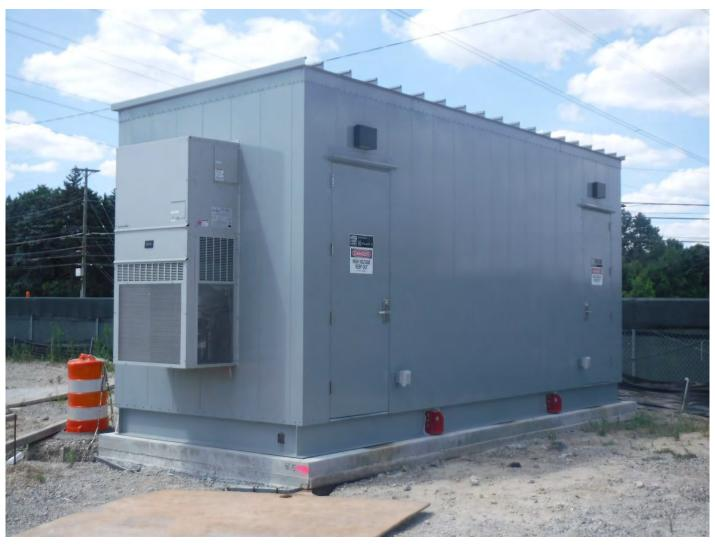
Figure 13 - CS-12 Pump Station MCC Enclosure
