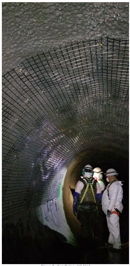
Figure 8 - Installation of C-Grid
