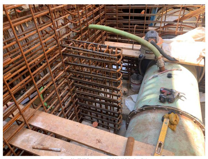
Figure 16 - CS-13 Construction - Wall Lift #1 Rebar Installation
