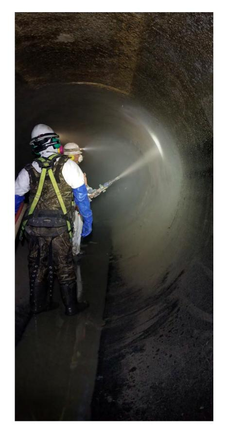
Figure 7 - Spray-Lining Base Layer
