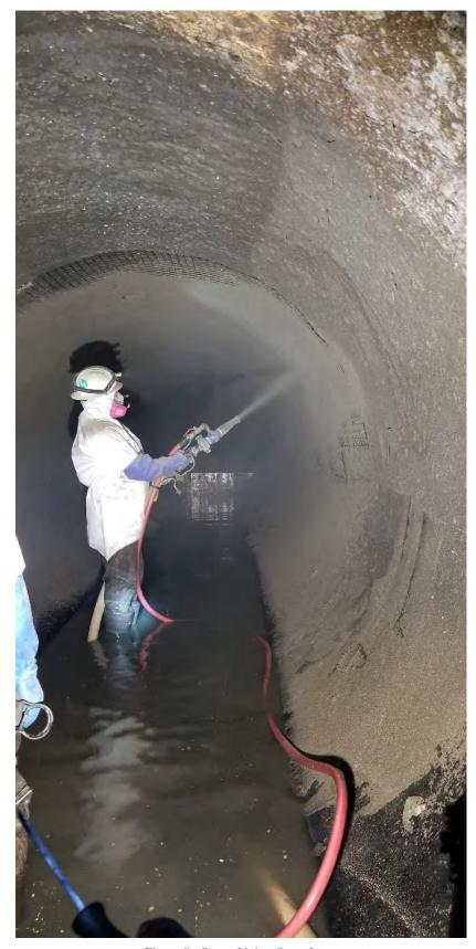
Figure 9 - Spray-Lining Outer Layer
