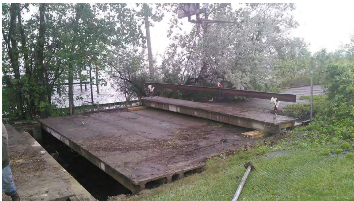
Concrete plank removal
