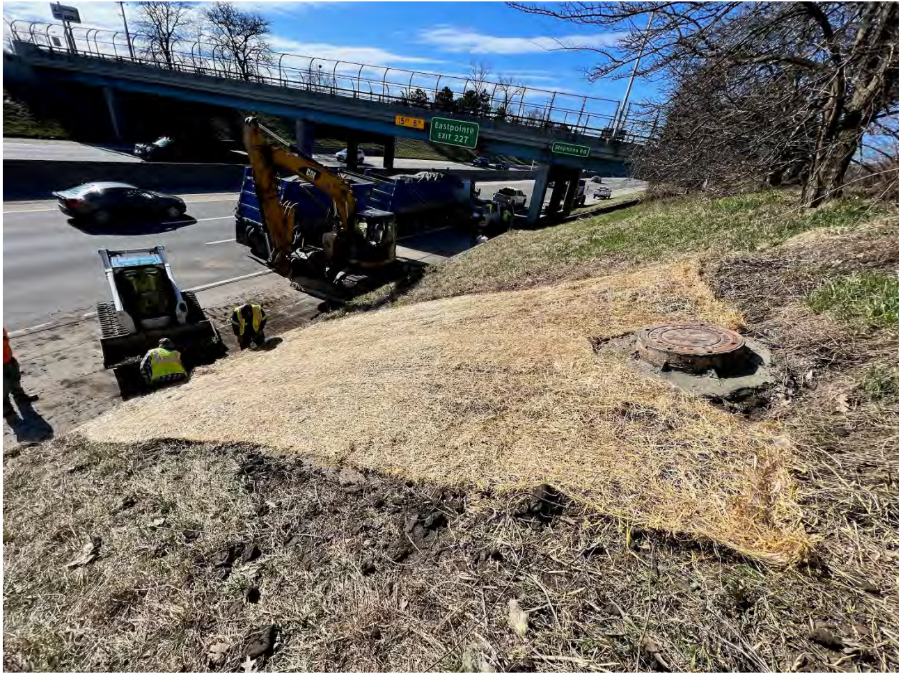
Figure 4 - Manhole Repaired & Grade Restored
