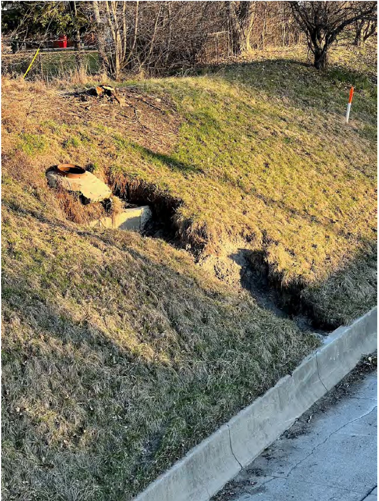
Figure 3 - Damaged Manhole
