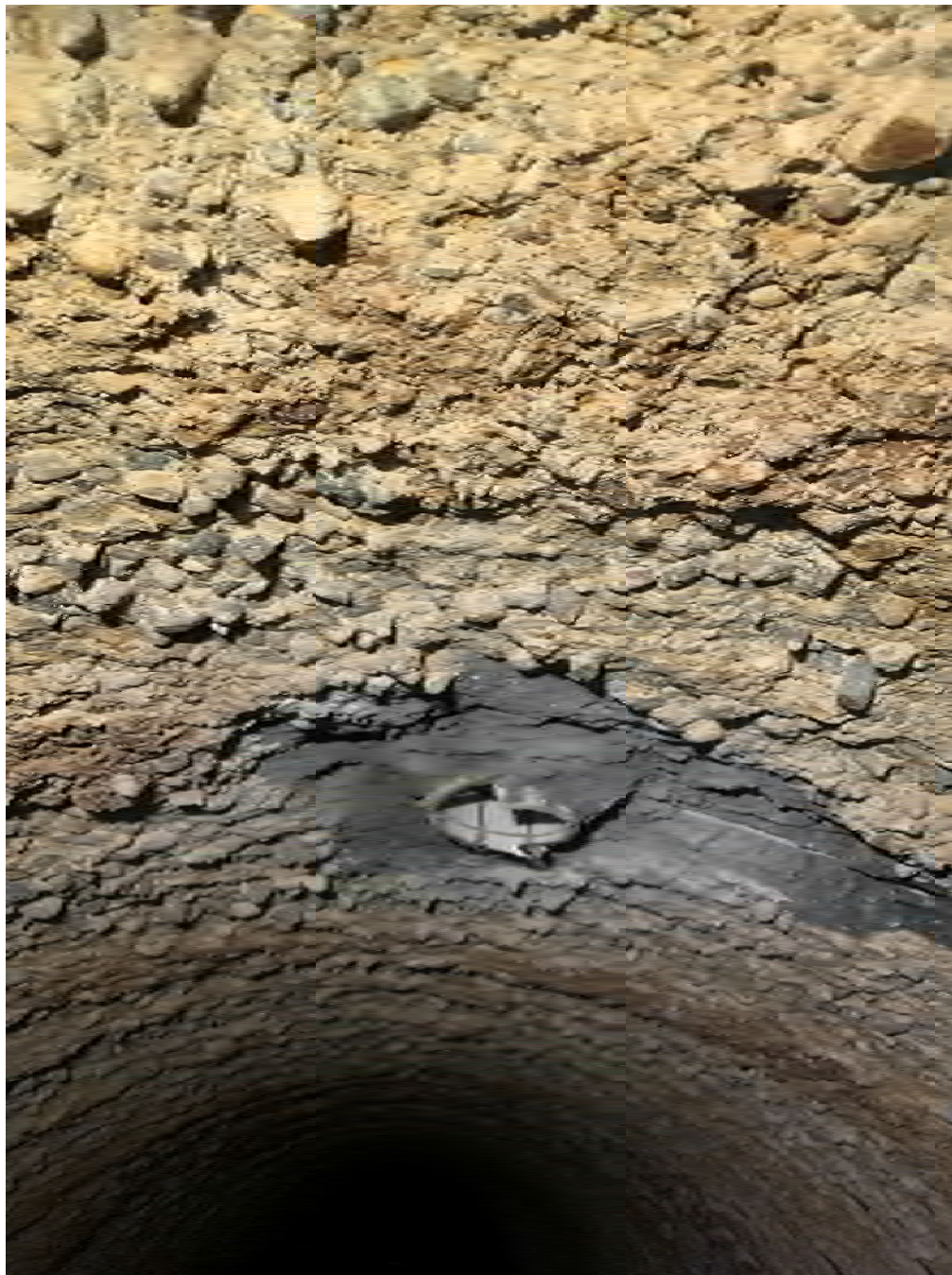
Figure 11 - Drop Grout Port
