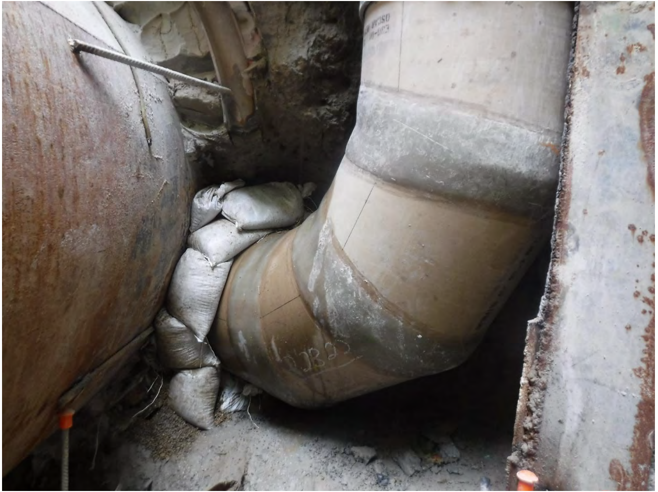
Figure 6 – Drop Pipe at Southwest Corner of CS-12
