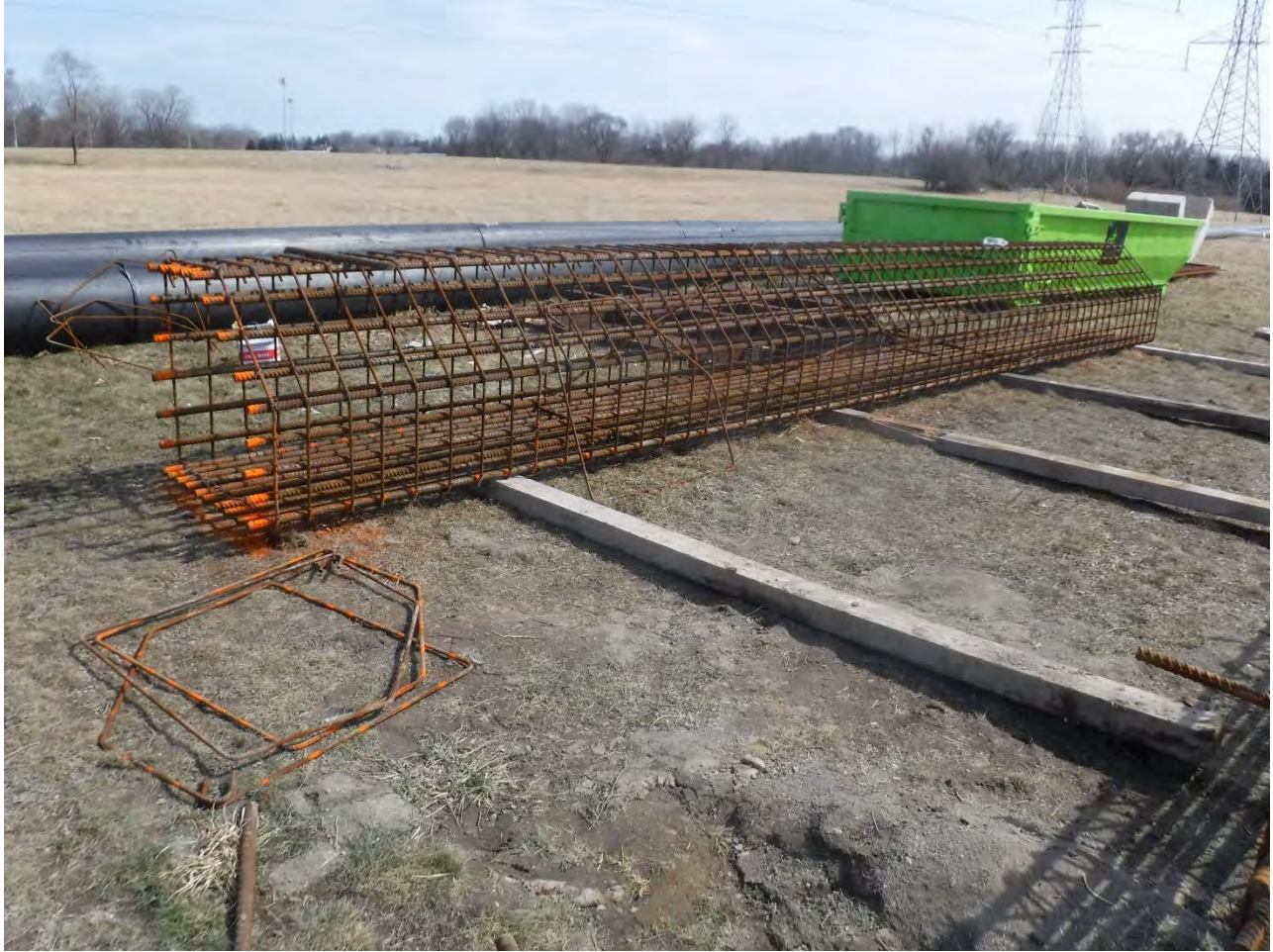
Figure 5 – CS-12 Column Steel Rebar
