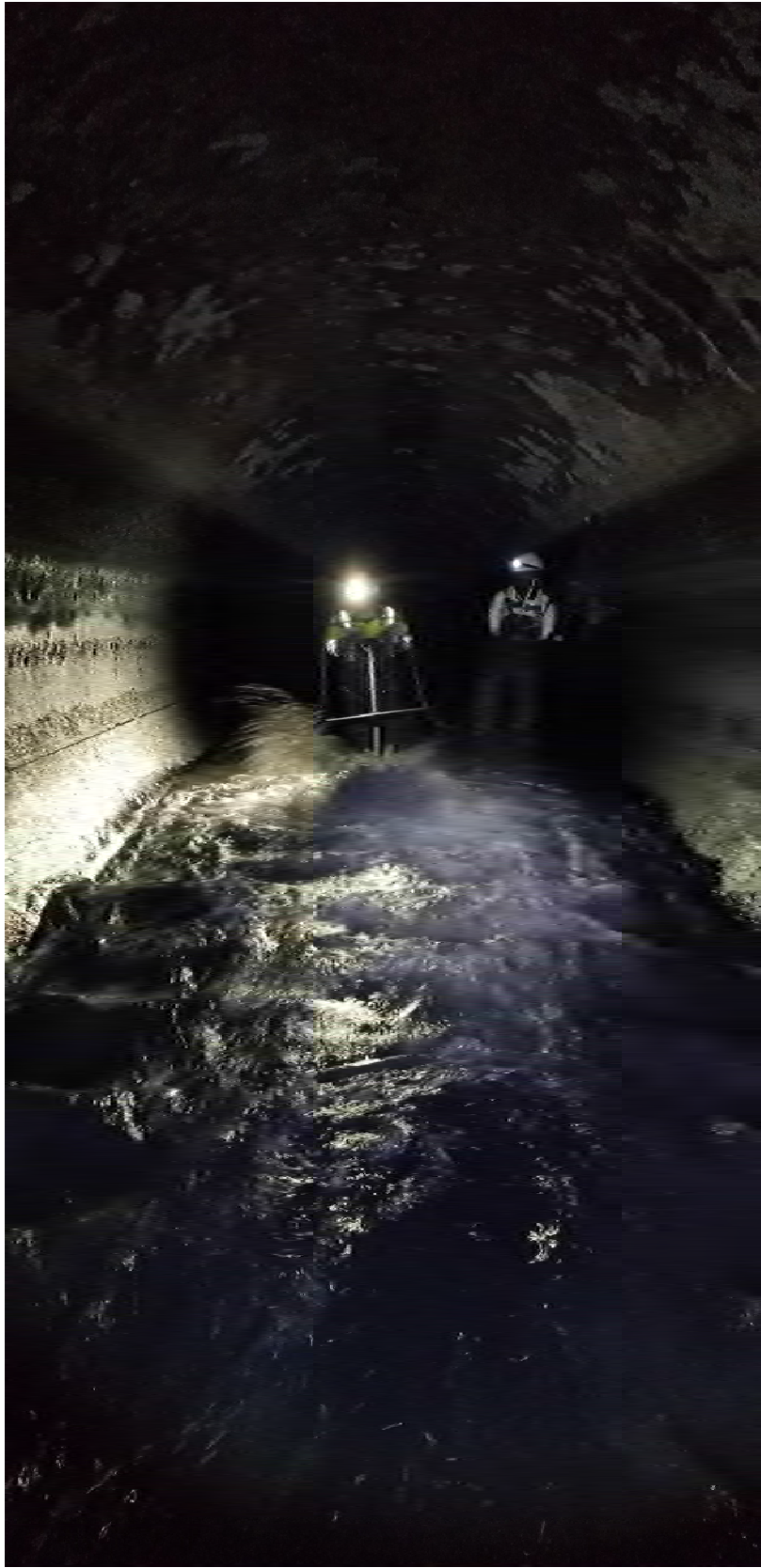
Figure 3 – Pushing Debris with Air Lancing from within the 8-Foot Interceptor
