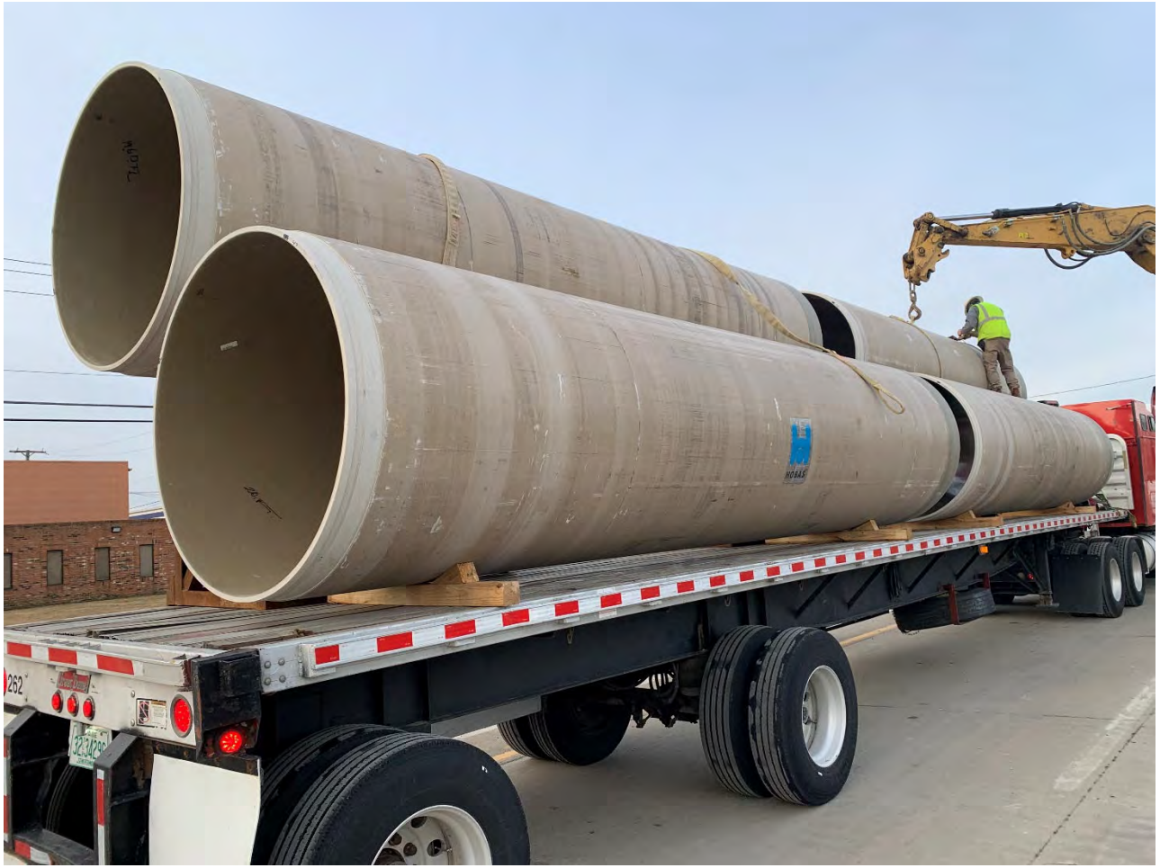
Figure 12 – Unloading HOBAS from Delivery Truck
