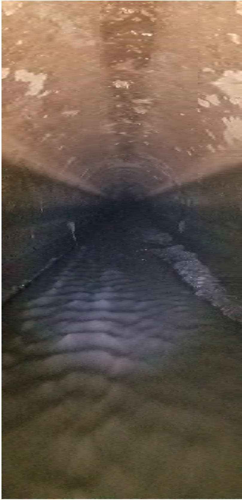
Figure 2 – View within the 11-Foot Interceptor during Dewatering
