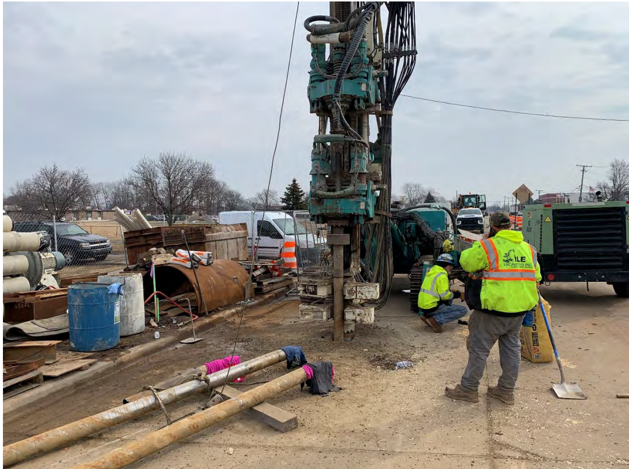
Figure 10 – Drilling the Grouting Drop Ports
