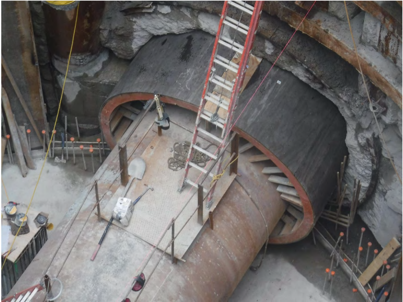
Figure 7 – Installing Formwork around the Interceptor for the CS-12 Finish Structure
