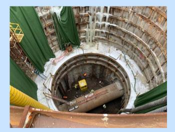
Crews at Segment 5 are working approximately 70 feet below grade and constructing what will become the permanent pump station.
