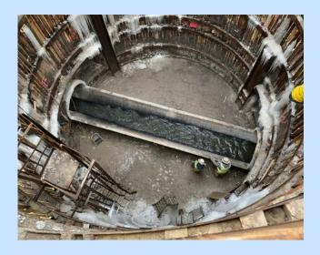
40 feet below the surface, a construction crew "exposes" the interceptor by cutting and removing a section of the concrete pipe in Segment 6 of the MIDD, on 15 Mile, east of Garfield Road.
