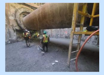
At Segment 5 of the Macomb Interceptor Drain sewer rehabilitation, on 15 Mile Road in the ITC corridor, the construction contractor works at the bottom of the shaft and next to the flume carrying the sanitary sewage from the 11 communities in the Macomb Interceptor Drain Drainage District.
