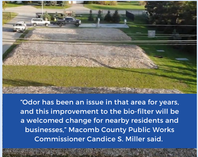
Biofilter off 15 Mile Road
