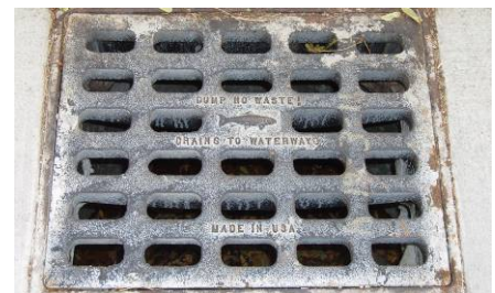
Courtesy of Center Line
