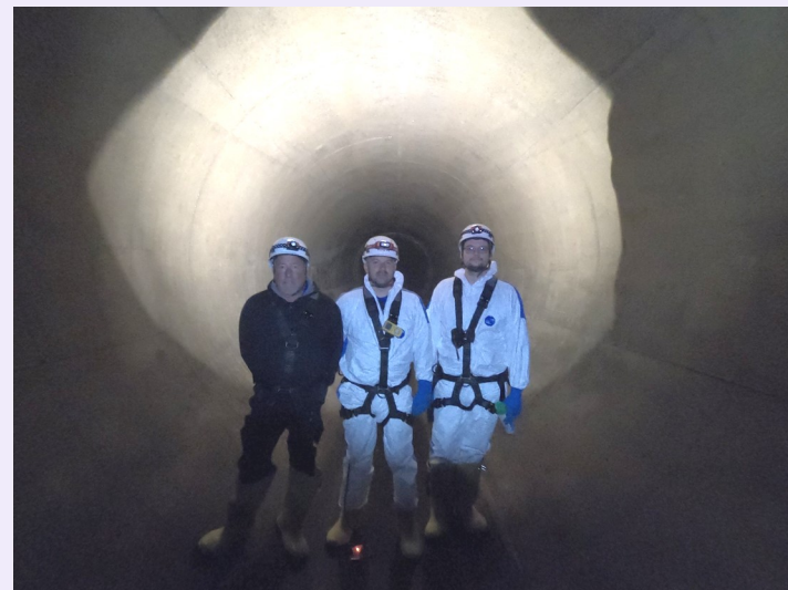
MCPWO employees in the 8 1/2 Mile Relief pipe, about 45 feet below Eastpointe. Employees make periodic walks of the pipe to look for abnormalities.
