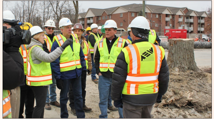
Commissioner Miller, County Executive Mark Hackel and others brief Gov. Rick Snyder during an early January visit to the sewer collapse site.
