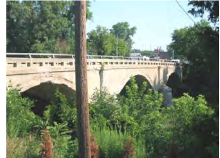
Gratiot Ave. Bridge
