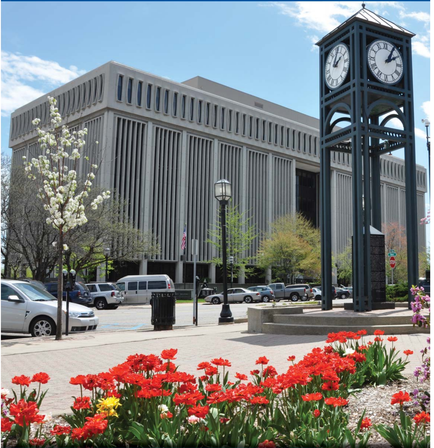
Macomb County Court Building in the Spring.
