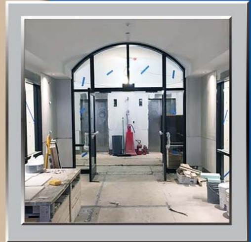
Old County Building West Entry Corridor renovations.
