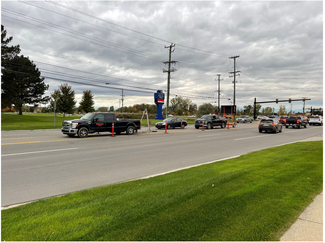
Figure 4 - Garfield Interceptor MH-19 Setup Near Hall Road
