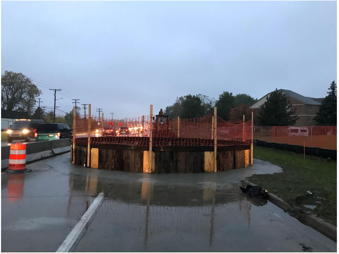
Figure 12 - CS-13 with Top Rib & Lagging Sets Installed
