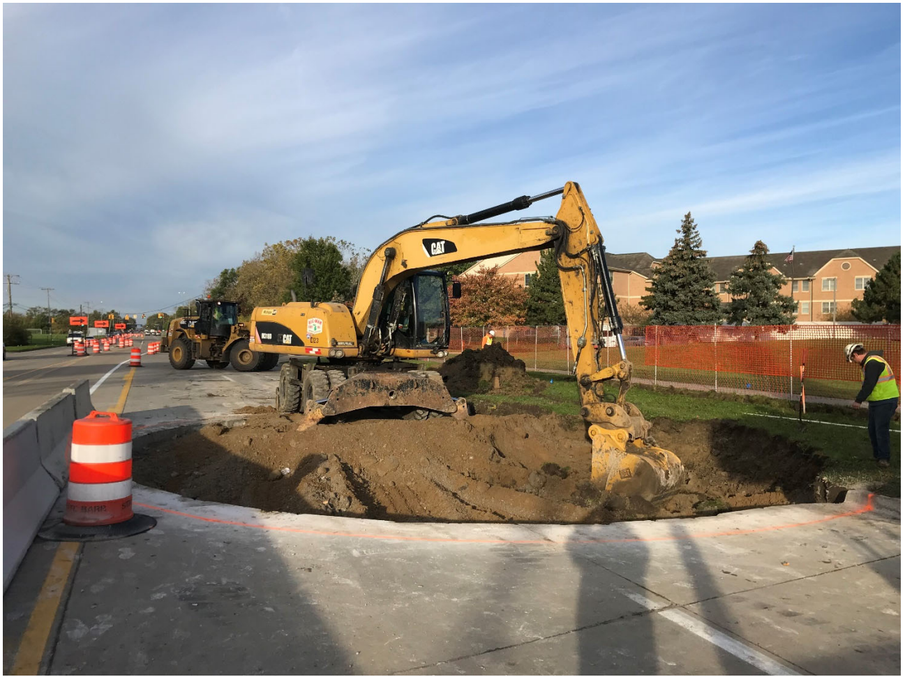
Figure 8 - Start of Excavation at CS-13
