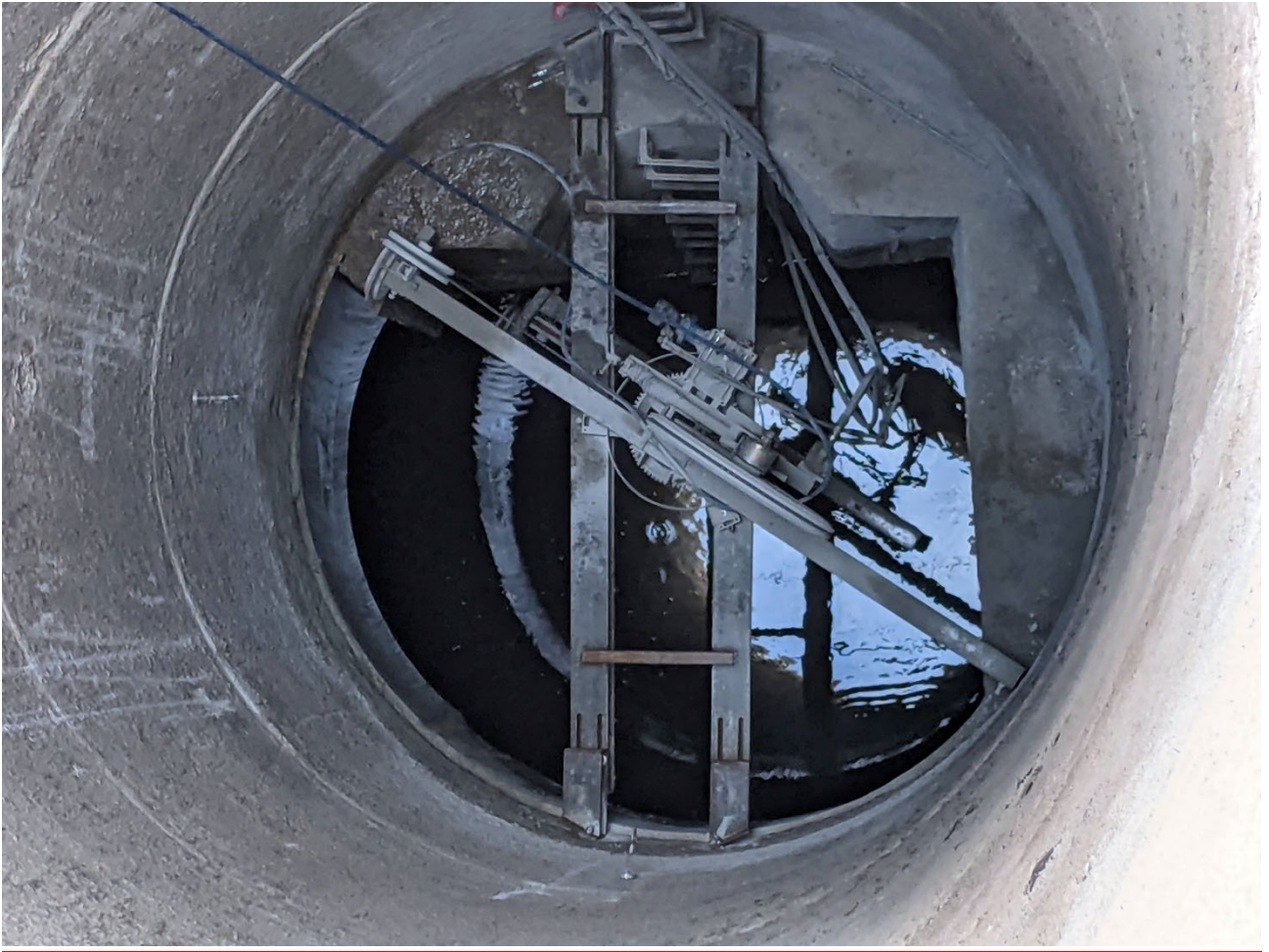
Figure 2 - Sawcutting to Increase MH-05 Opening
