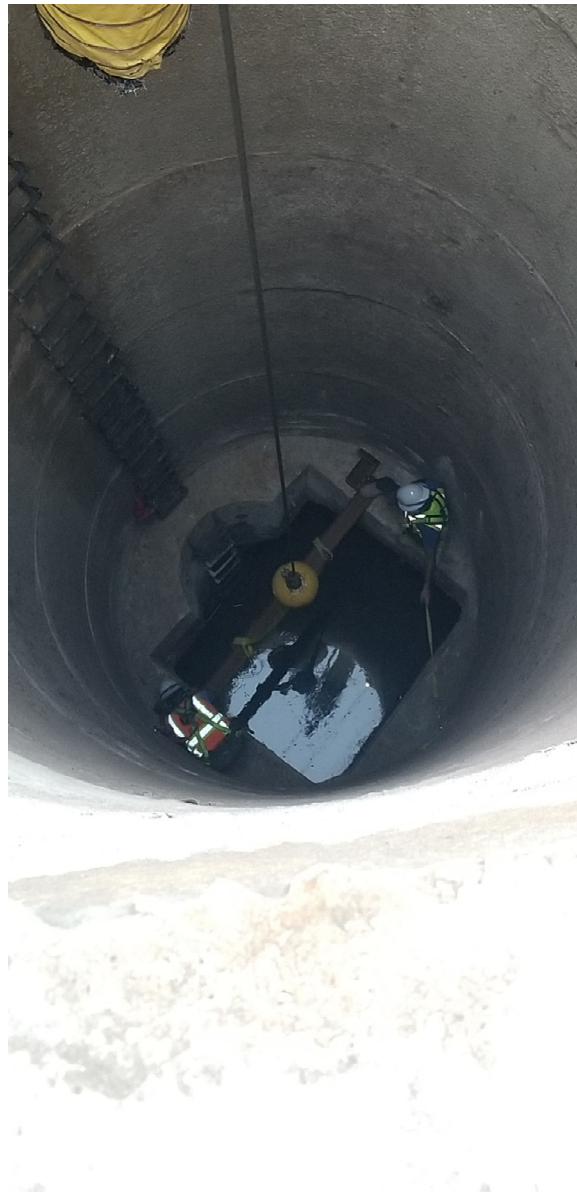
Figure 1 - Sawcut Preparation at MH-05
