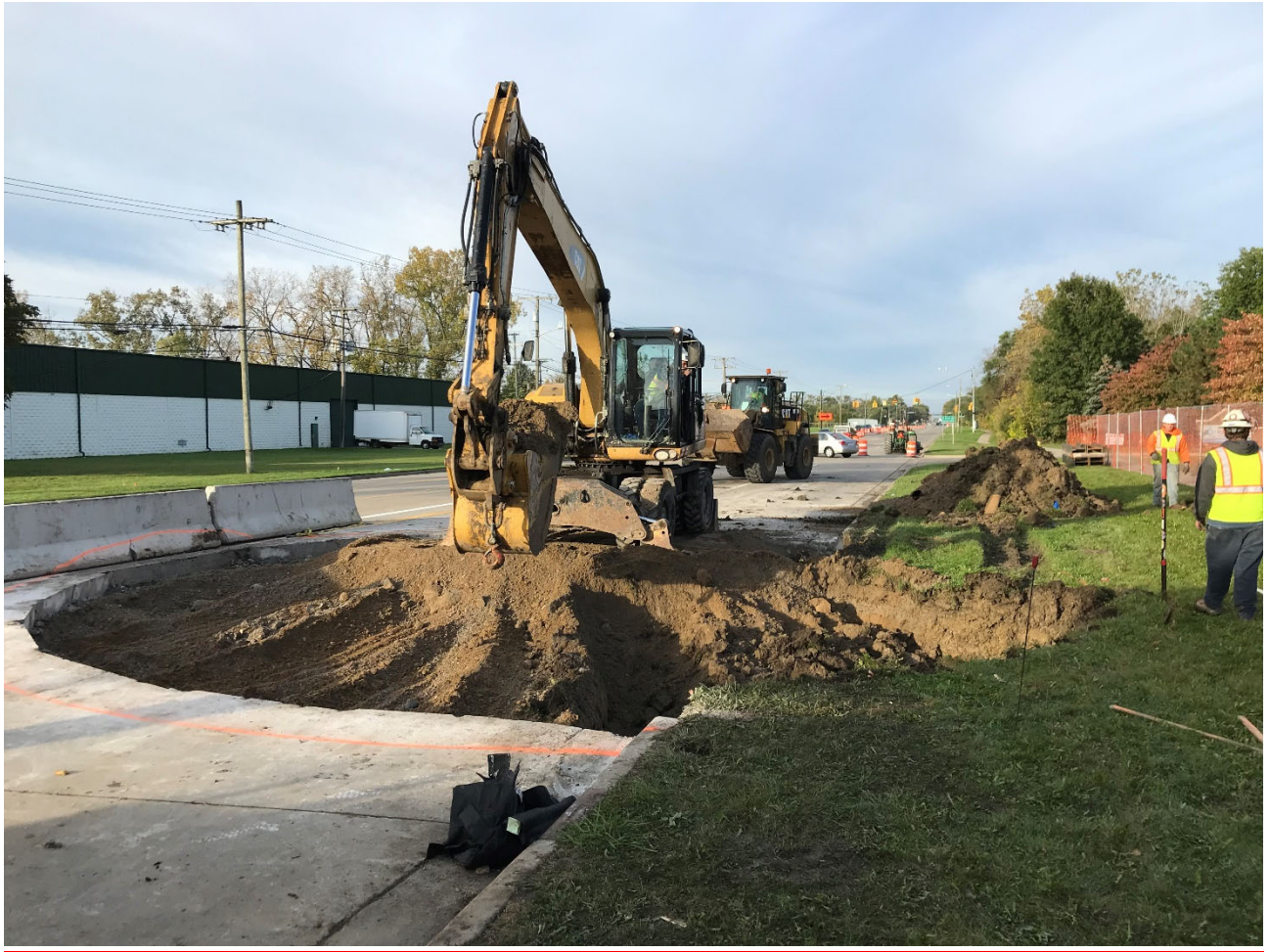
Figure 9 - Start of Excavation at CS-13
