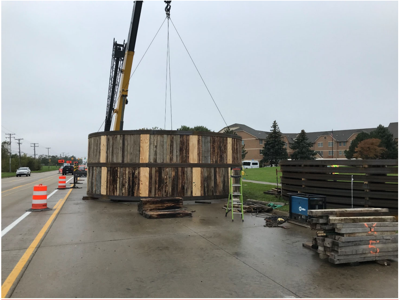
Figure 11 - Preparation to Hoist Top Rib & Lagging Sets into Excavation
