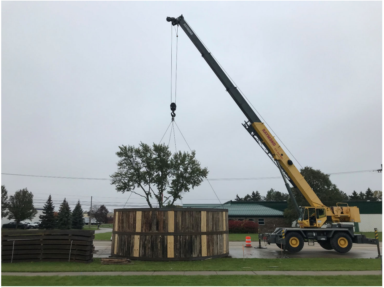
Figure 10 - Construction of the Top Two Rib & Lagging Sets
