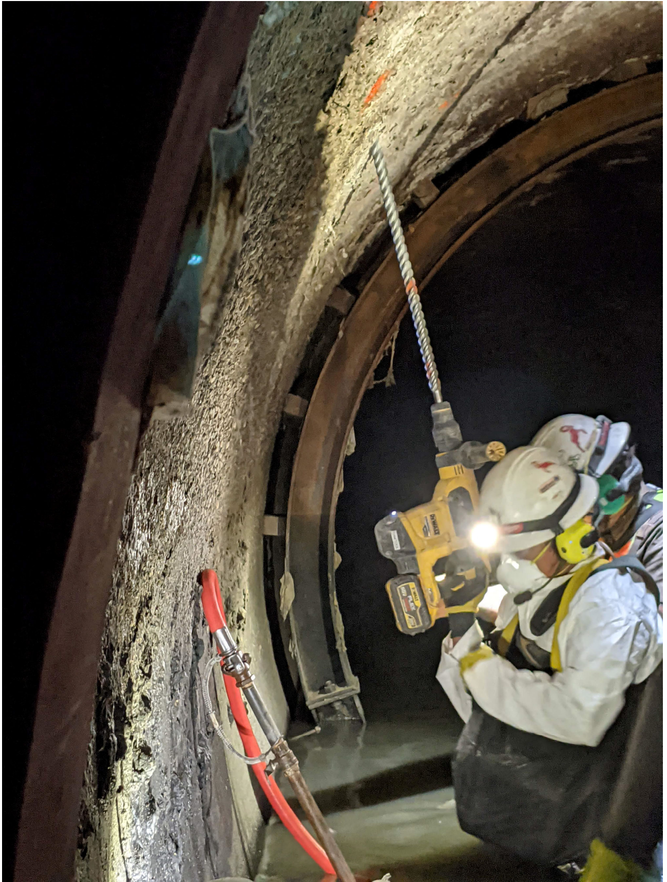
Figure 3 - Chemical Injection Grouting at MH-05
