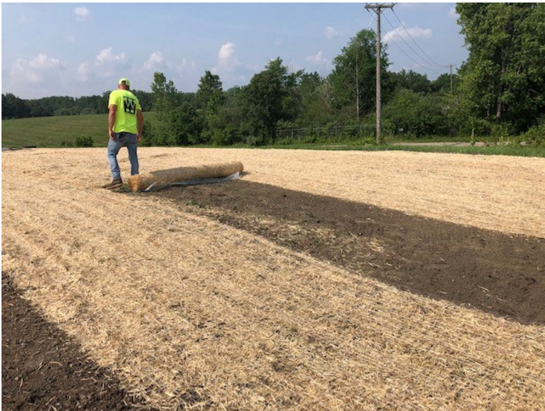
Figure 8 - Site Restoration at SY-S-2
