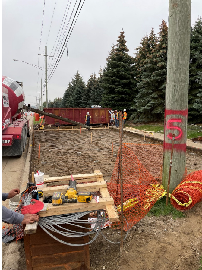
Figure 4 - Temporary Concrete Pad
