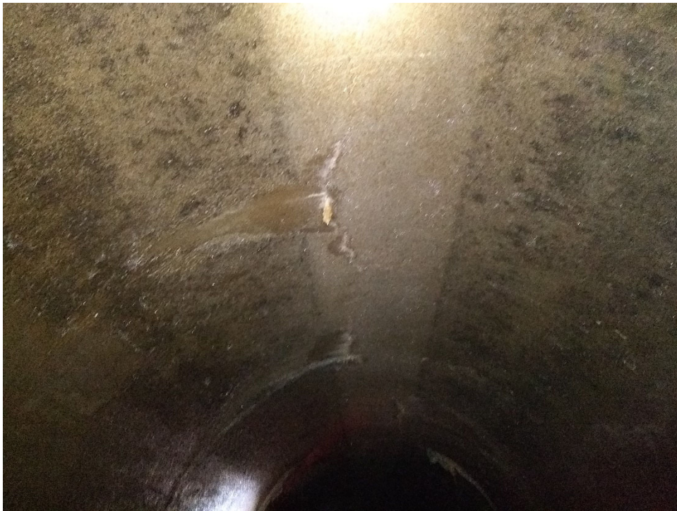
Figure 6 - Dripping Infiltration
