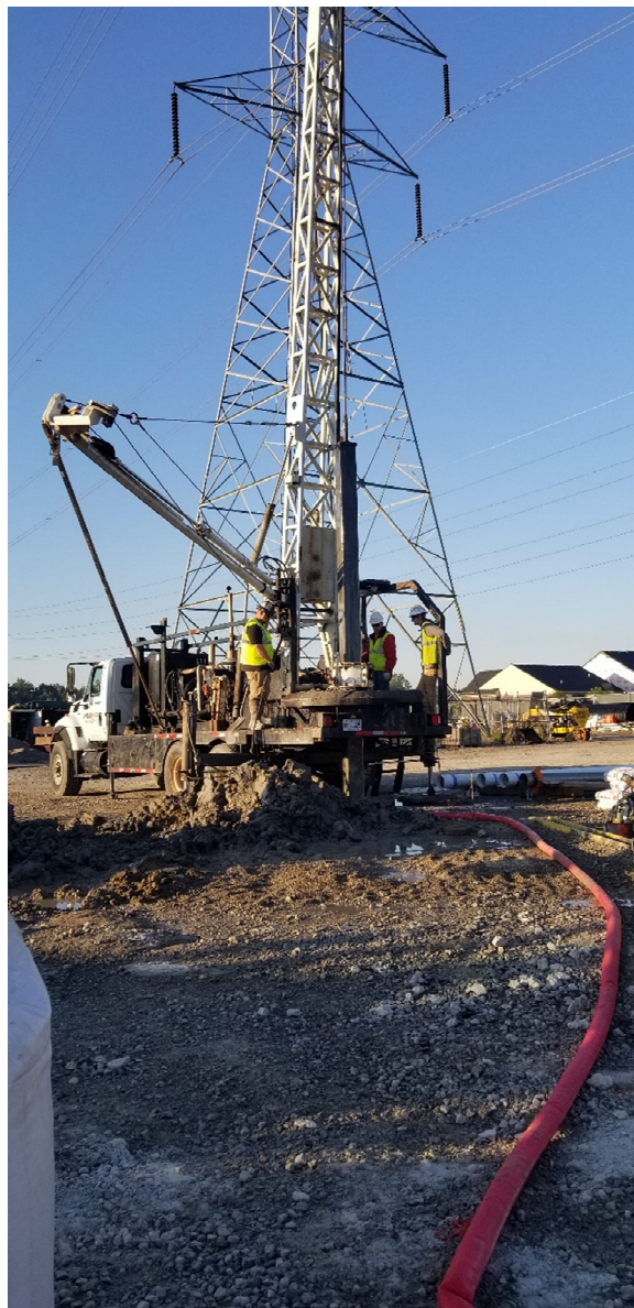
Figure 1 – Drilling Additional Dewatering Well
