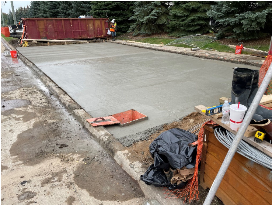
Figure 3 - Temporary Concrete Pad
