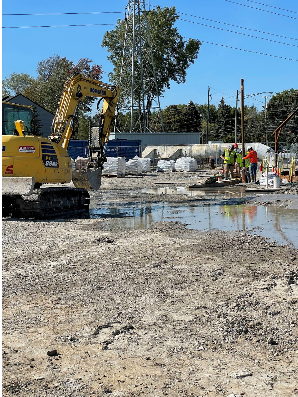
Figure 2 - Dewatering Pump Maintenance
