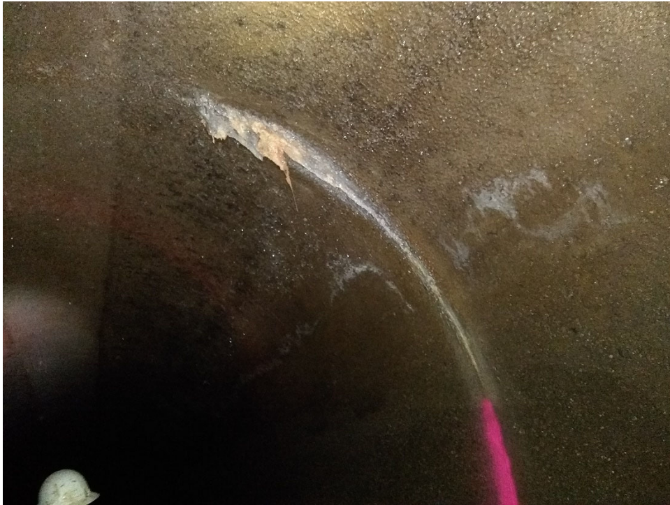
Figure 5 - Dripping Infiltration
