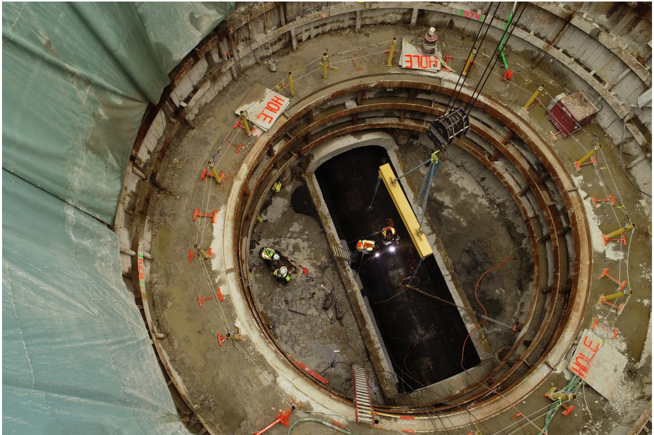
Figure 3 - Installation of Temporary Flume
