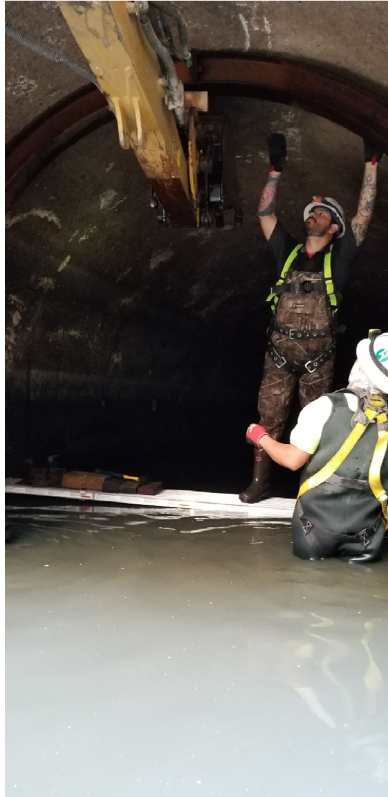
Figure 1 – Temporary Internal Steel Rib Removal
