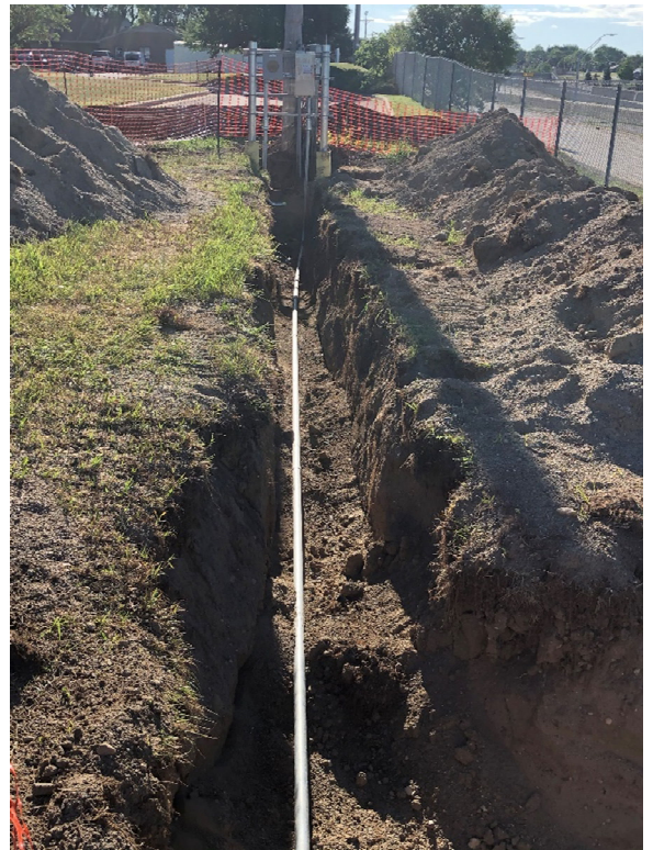
Figure 8 - New Electrical Conduit at SY-S-1
