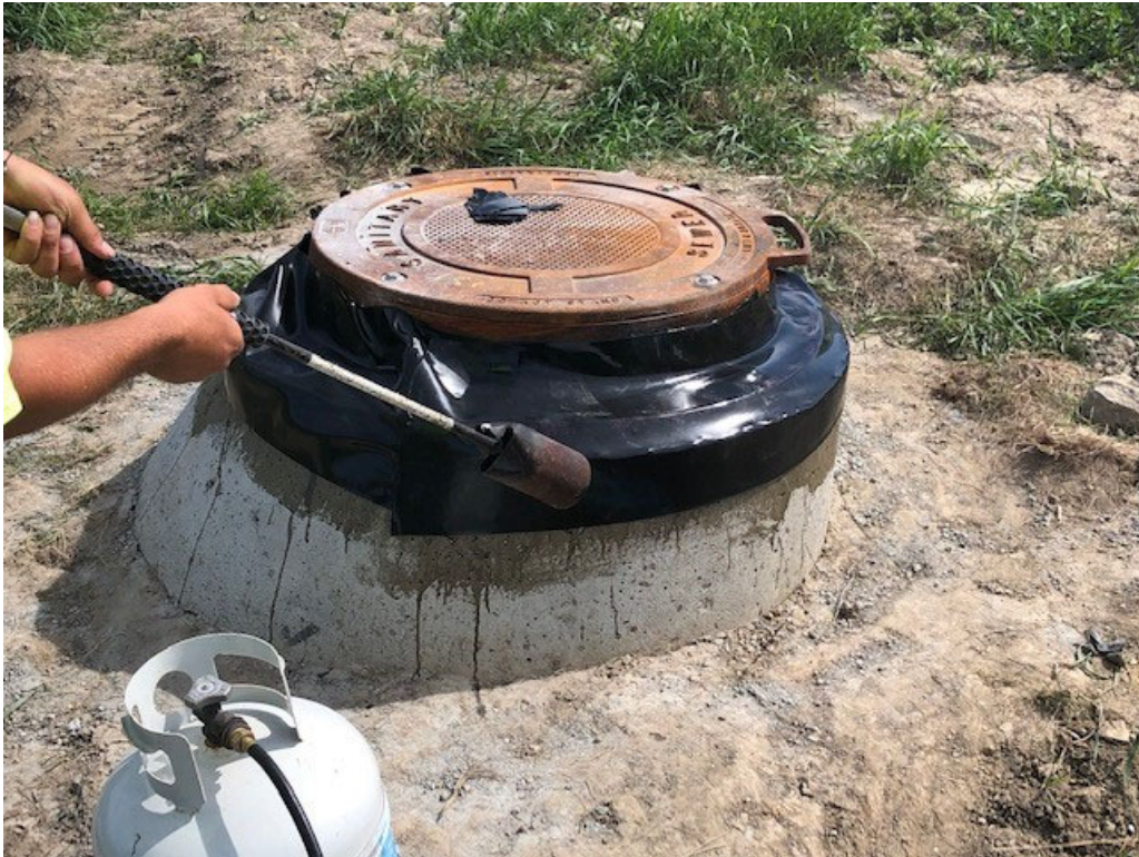
Figure 14 - Waterproofing Exterior of Manhole at SY-S-2
