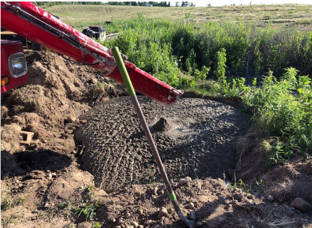
Figure 12 - Placing Flowable Fill to Abandon Old Structure
