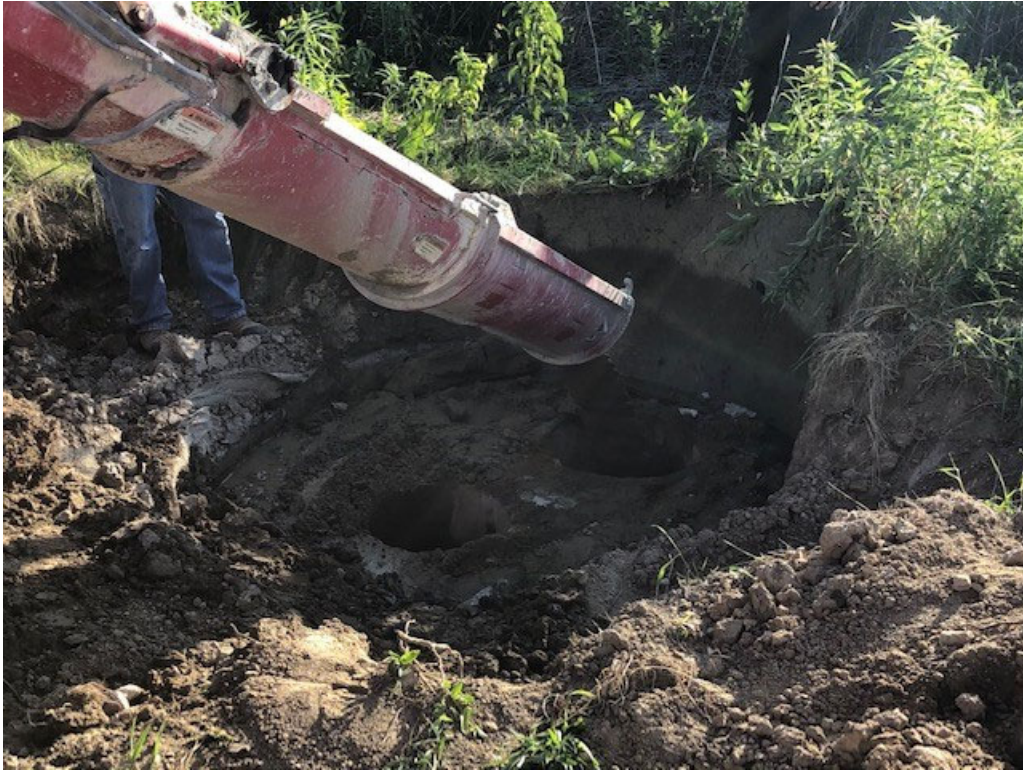
Figure 11 - Abandoning Existing Meter Pit at SY-S-2
