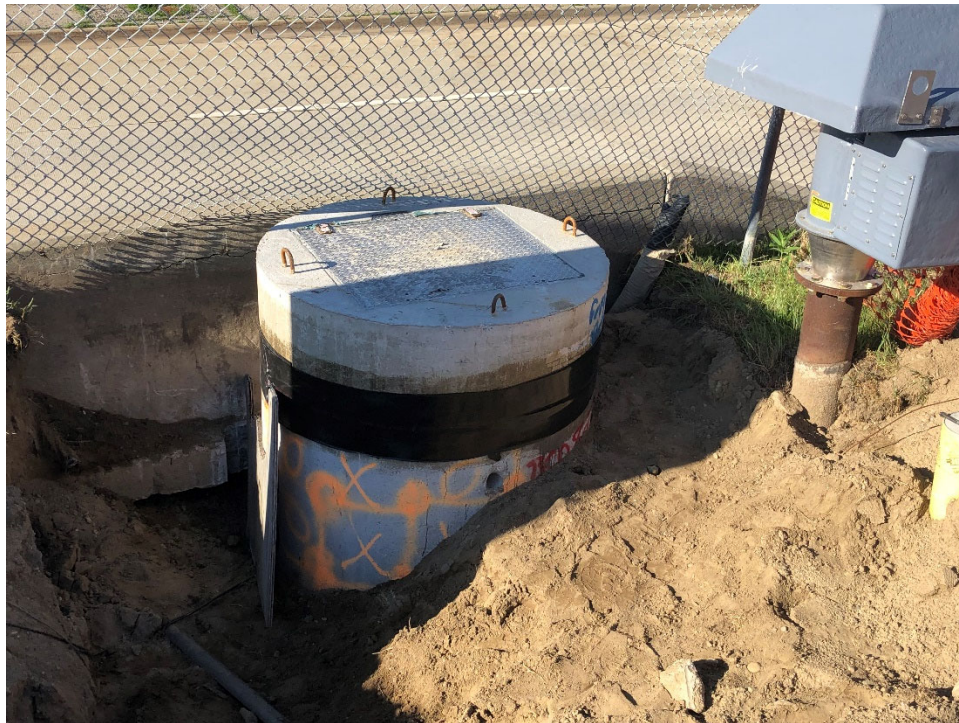
Figure 9 - Waterproofing Manhole Exterior
