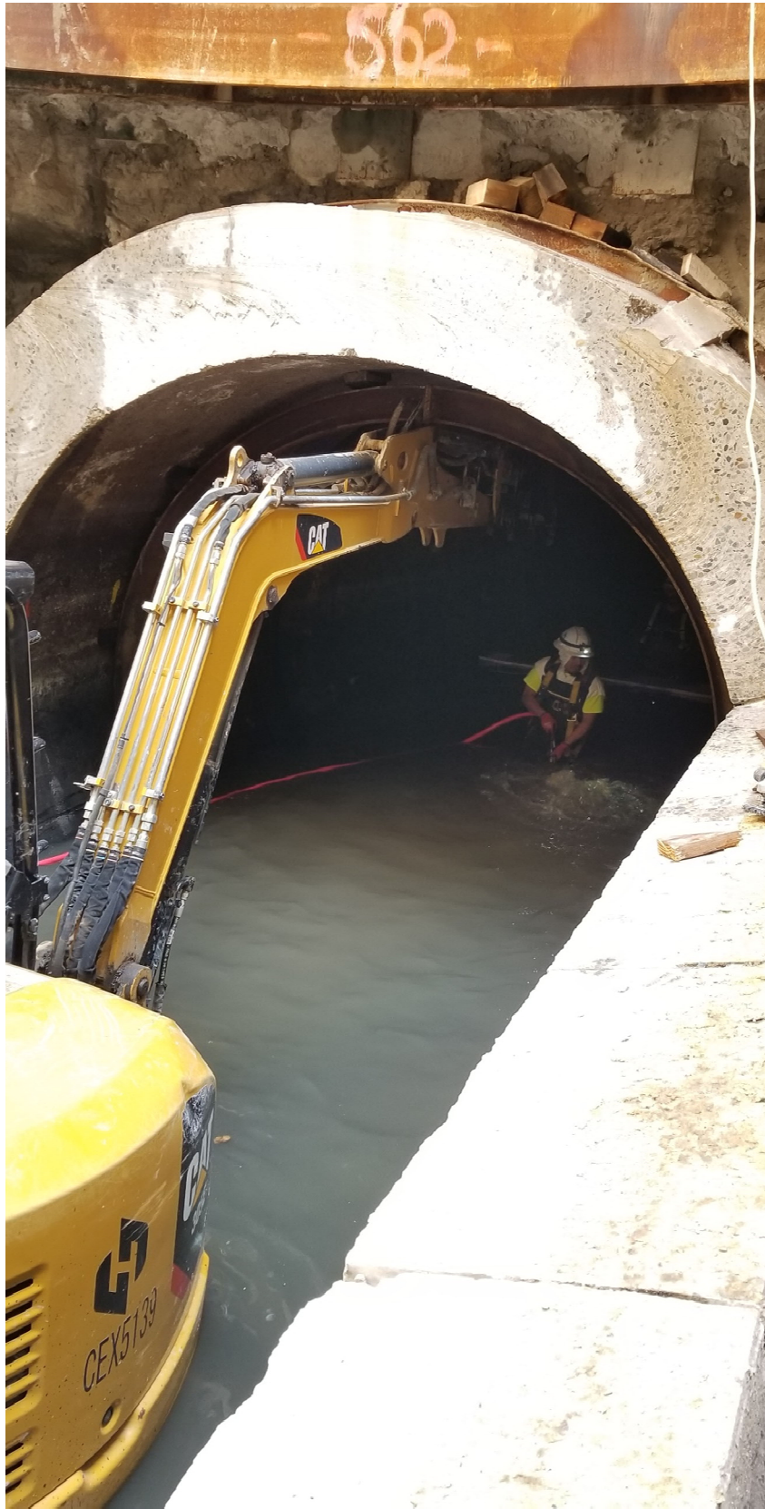
Figure 2 - Temporary Internal Steel Rib Removal
