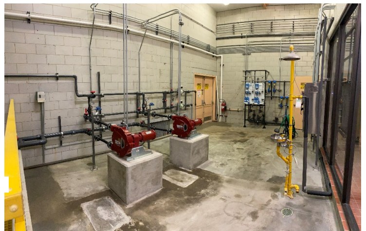
Figure 2 – Pump Room after pump and pad removal
