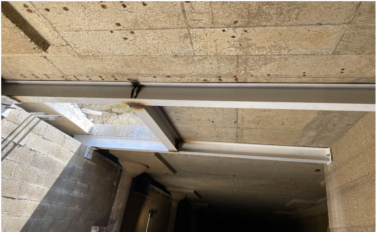
Figure 2 - Installed Steel Supports Underside of RTB Basin Roof
