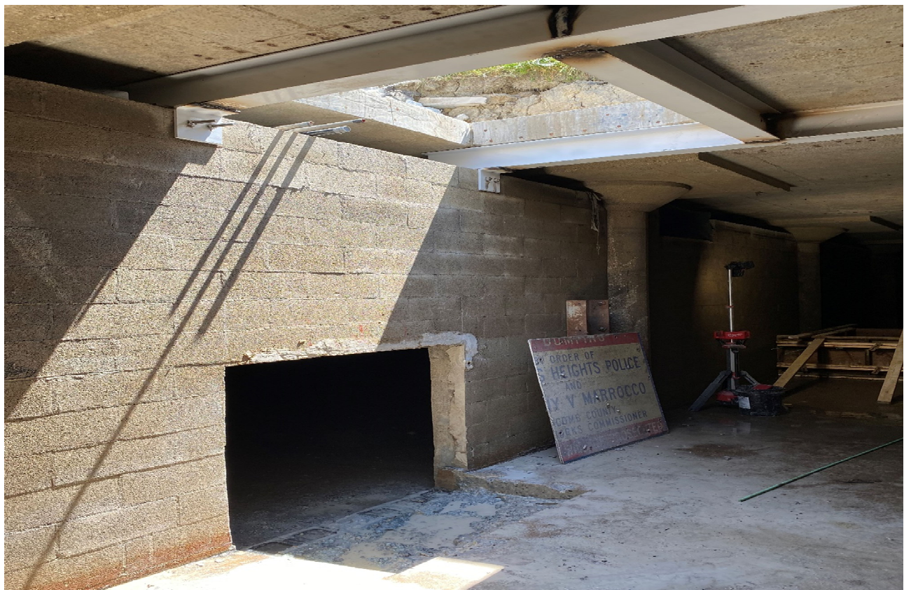
Figure 3 - Cut Block for New Hydraulic Flushing Gates
