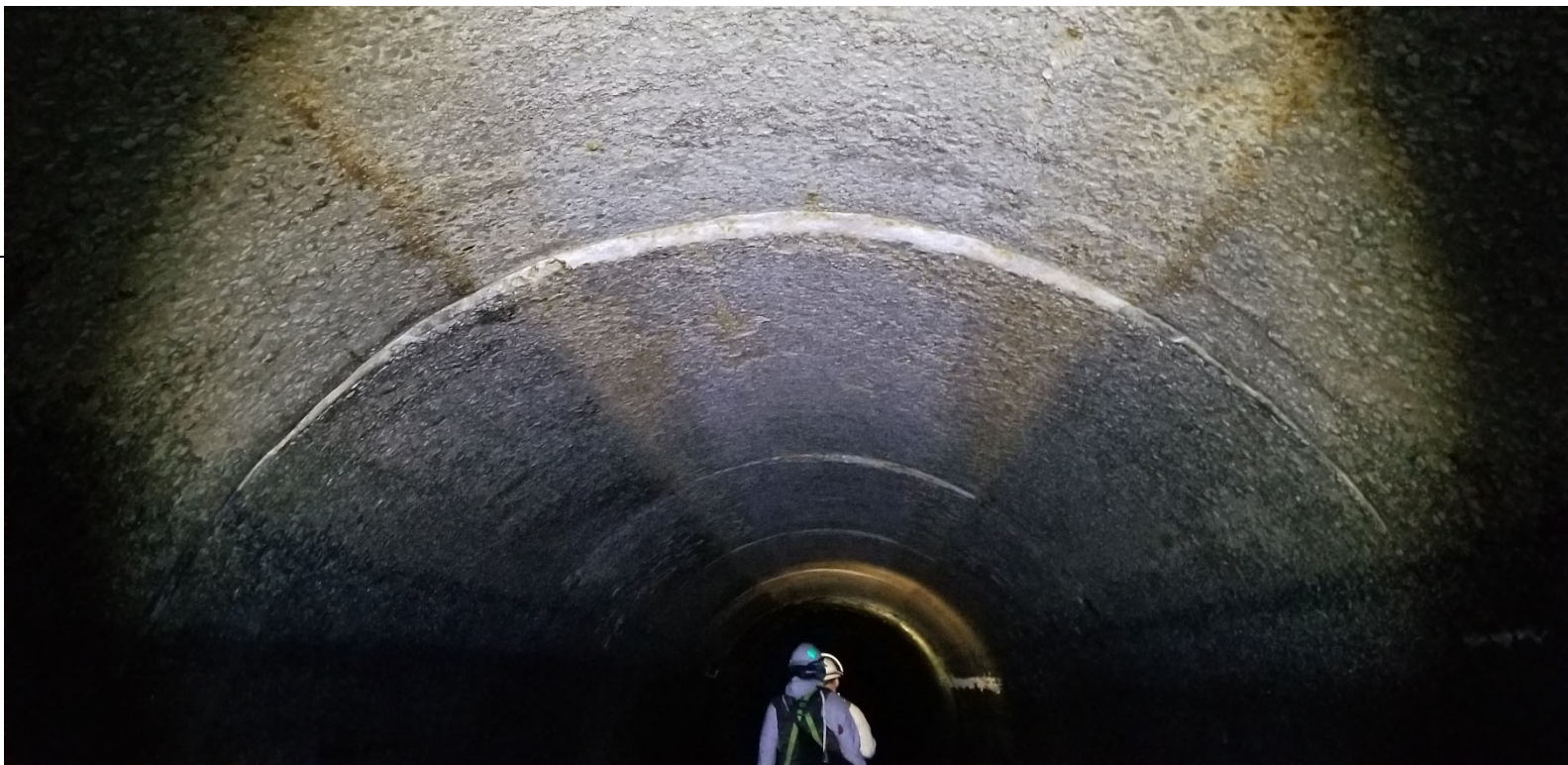
Figure 1 – PCI-37 (8-foot Pipe) Post Power Washing Inspection
