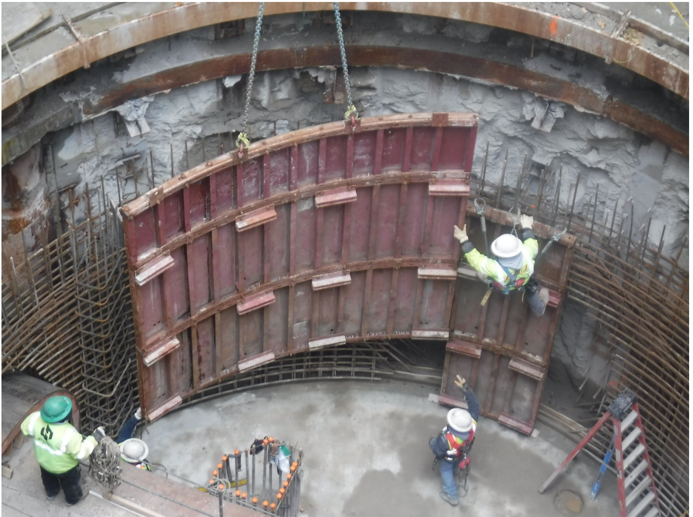
Figure 6 - CS-12 Concrete Formwork Installation
