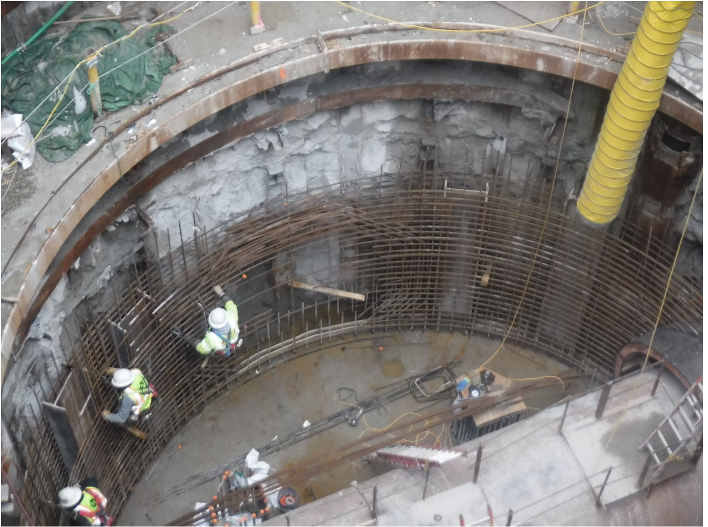
Figure 3 - CS-12 Rebar Installation
