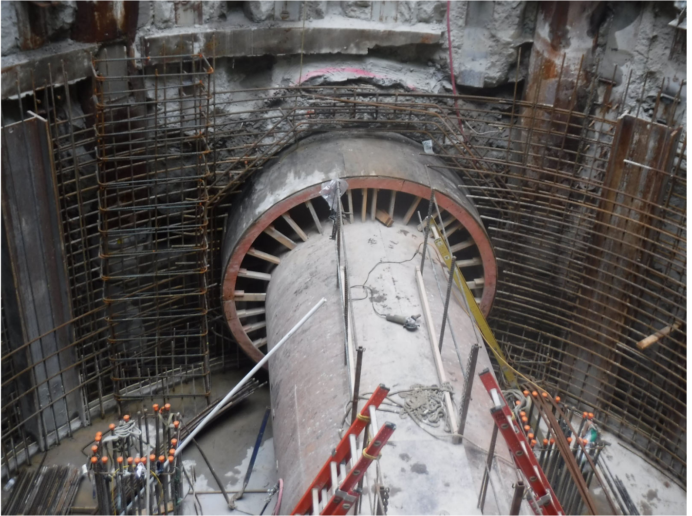
Figure 5 - CS-12 Rebar & Formwork Installation
