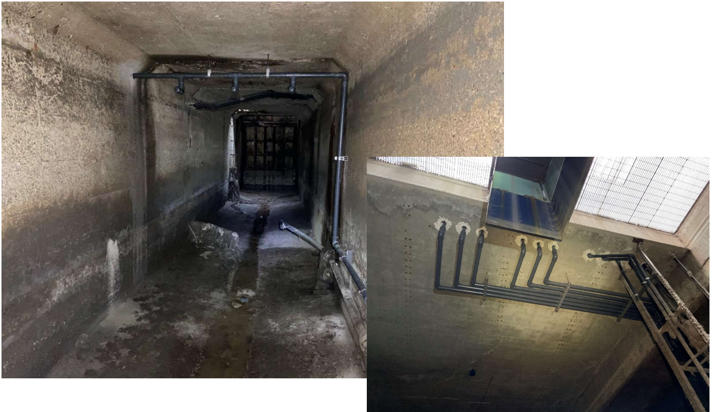
Figure 3 – New 2” sample piping through floor into Blower Room
