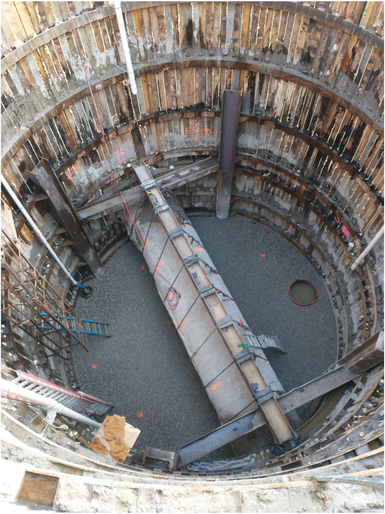
Figure 6 – CS-13 Shaft Excavation Complete & Prepared for Concrete
