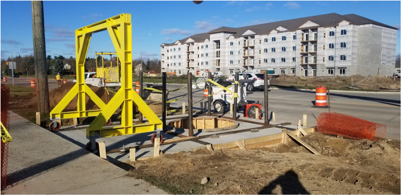
Figure 4 - MH-07 Interceptor Access Location for Spray-Lining Operation
