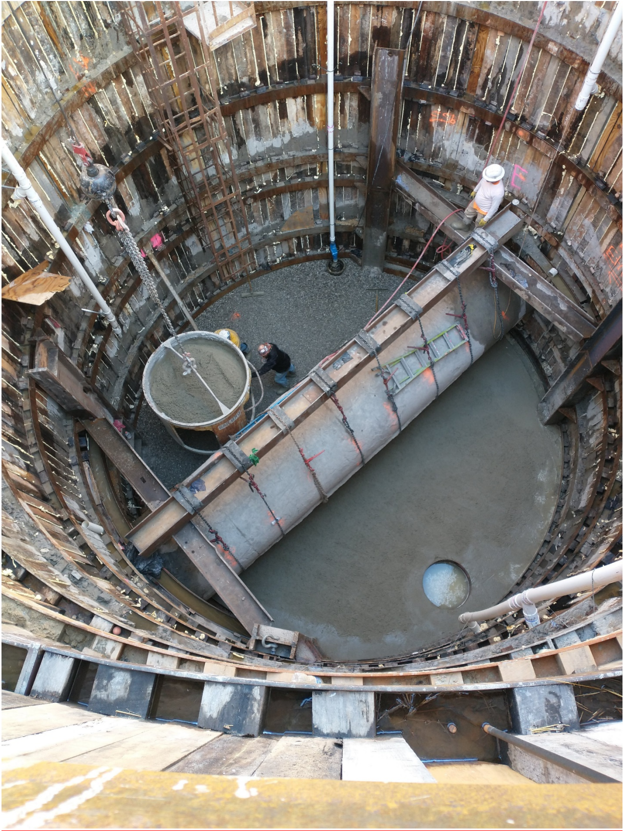
Figure 7 – Placement of the CS-13 Concrete Mud Mat
