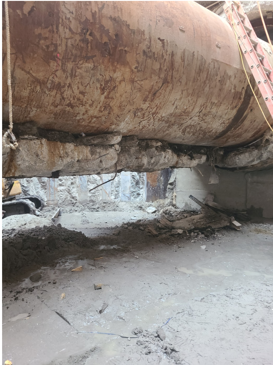
Figure 1 – Finished Excavation at CS-12
