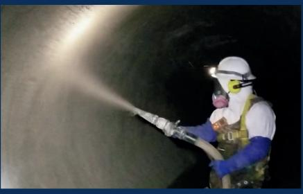
Spray lining/coating of 1,300 linear feet of 8-foot-diameter pipe with a corrosion resistant geo-polymer spray. To facilitate this work, a new control structure was built in a 70foot-deep access shaft excavated in the ITC Corridor. The new control structure provides the contractor the access to the sewer to facilitate the work and will also serve as a dewatering pump station to draw down the upstream water level in the sewer.
