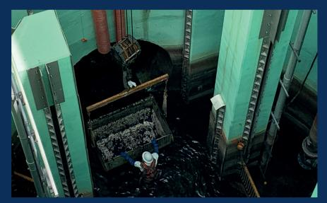
Painstaking removal of extensive sediment and debris, followed by cleaning and inspection of the pipe's invert.
