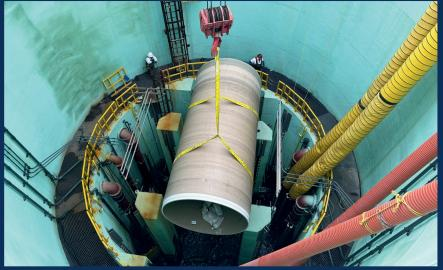
Segments of large, impervious pipe are being lowered into the interceptor to slip line 7,000 linear feet of the 11-foot diameter sewer, followed by grouting between the segments and the host concrete pipe.
