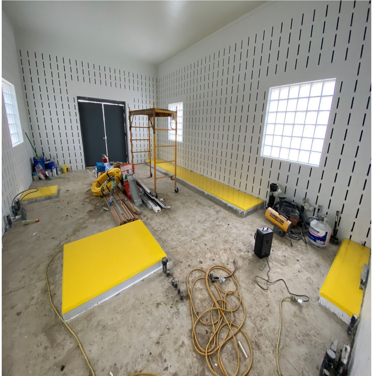
Figure 8 – New Paint in Control Bldg. @ Beaconsfield Rd.
