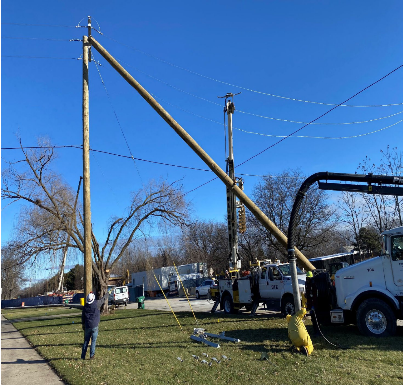
Figure 10 – DTE Placing New Poles @ Beaconsfield Rd
