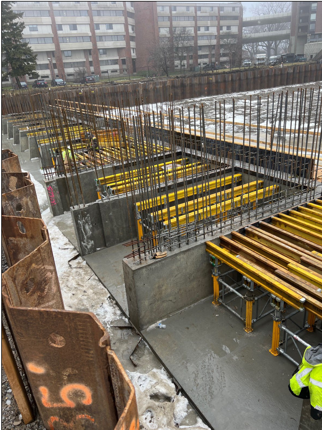
Figure 14 – Gate Slab decking and forms
