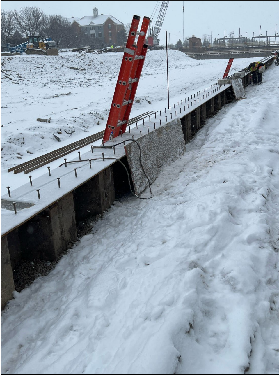
Figure 15 – New sheet pile cap and shear studs (south side)
