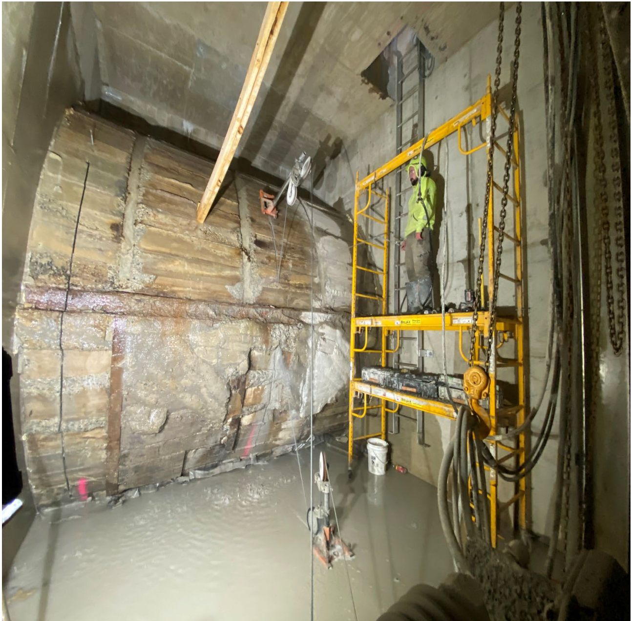
Figure 1 – Concrete Cutting @ Beaconsfield East Access Vault
