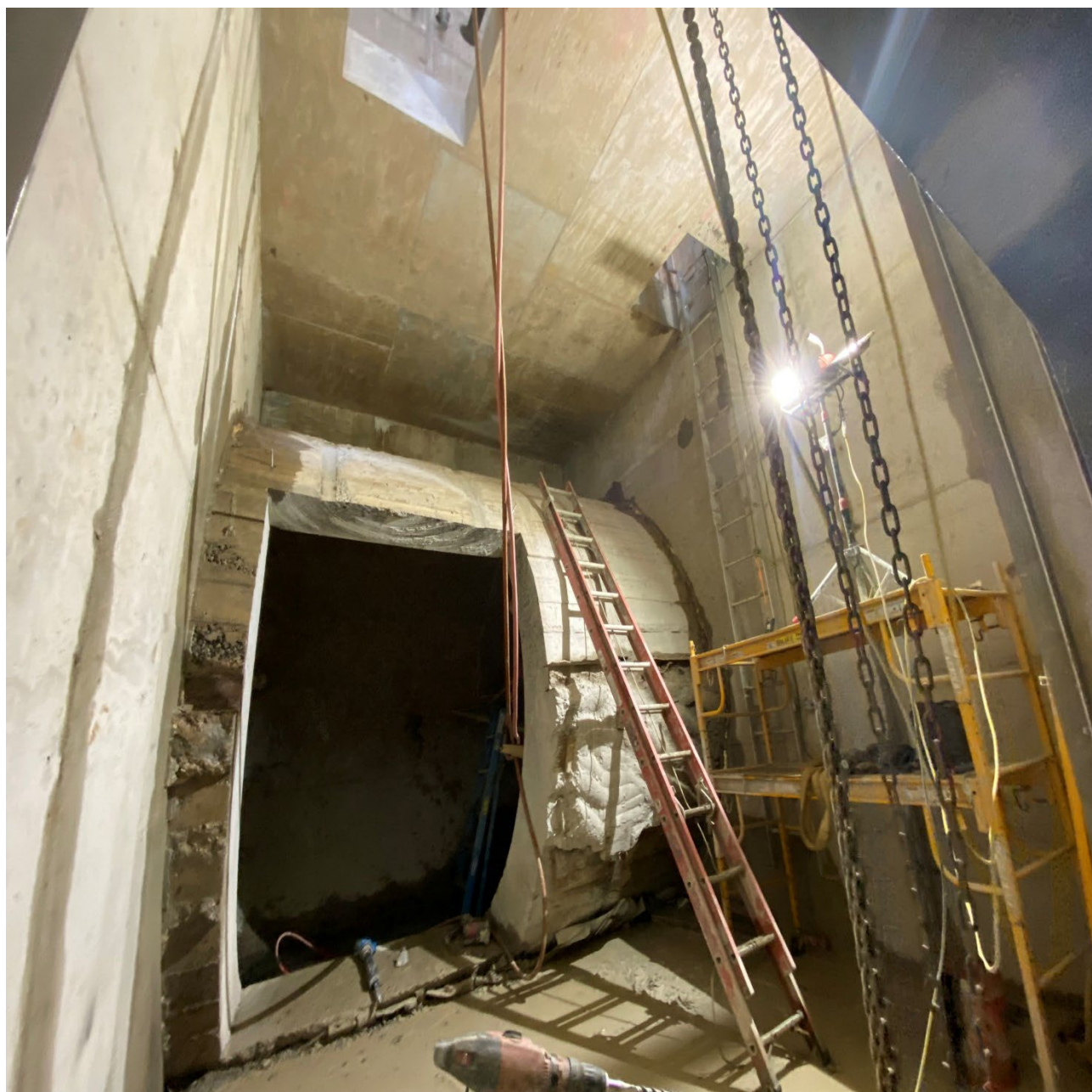
Figure 2 – Downstream Tunnel Opening @ Beaconsfield East Access Vault
