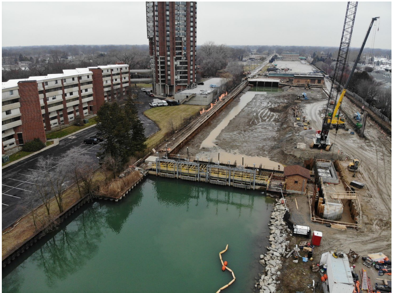
Figure 20 – Drone Aerial at 100 FT Facing West (02/01/24)
