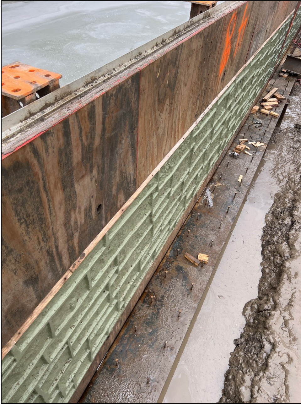
Figure 16 – Concrete pile cap forms with decorative-face forms being installed
