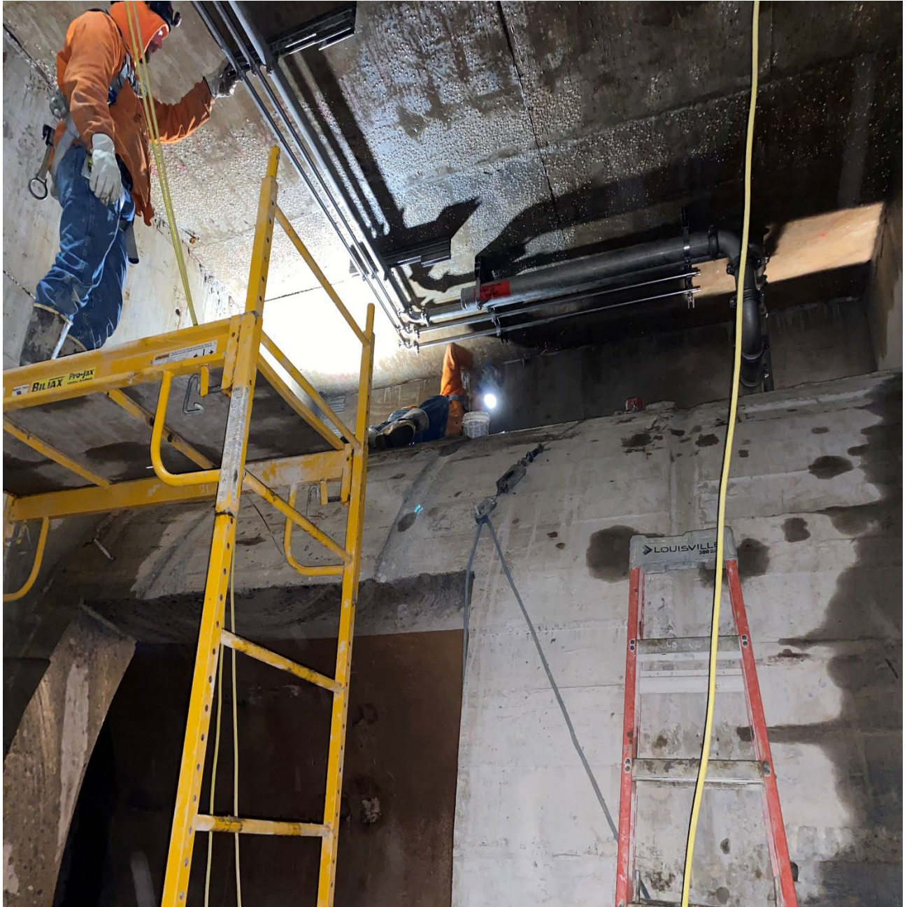
Figure 7 – Installing Process Conduit @ East Tunnel Access
