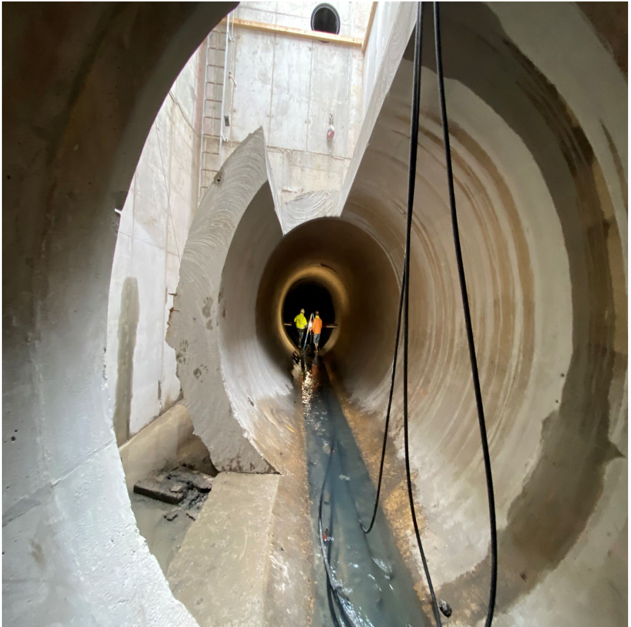
Figure 3 – Upstream Tunnel Opening @ Beaconsfield West Access Vault
