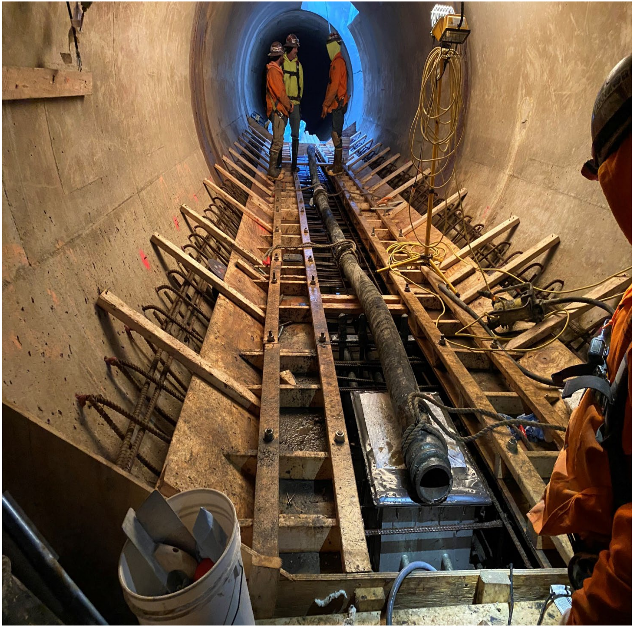
Figure 4 – Installed Steel & Conc. Forms for Rubber Dam Bench
