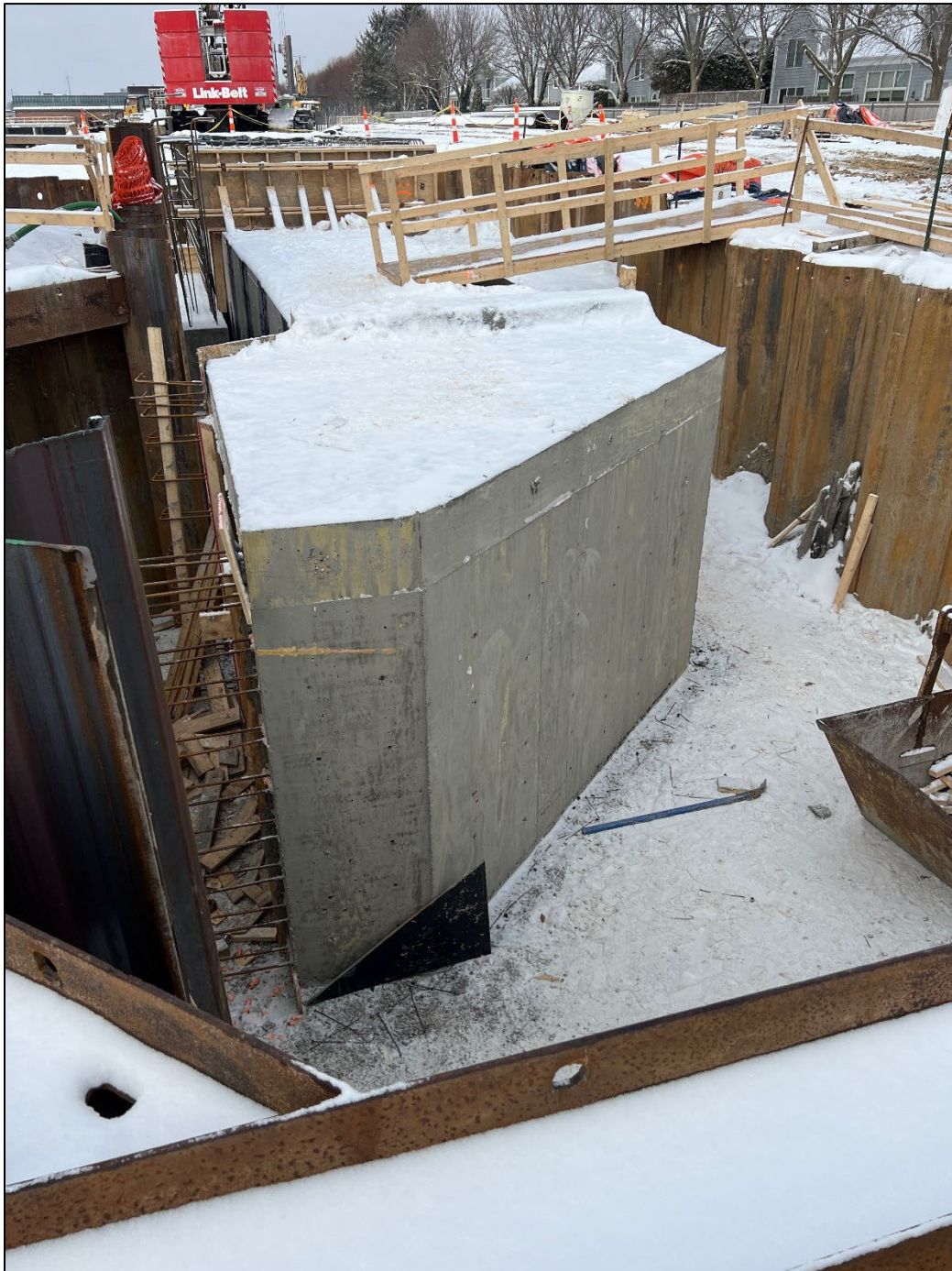
Figure 12 – Emergency Bypass Conduit ultimate outlet and headwall forms
