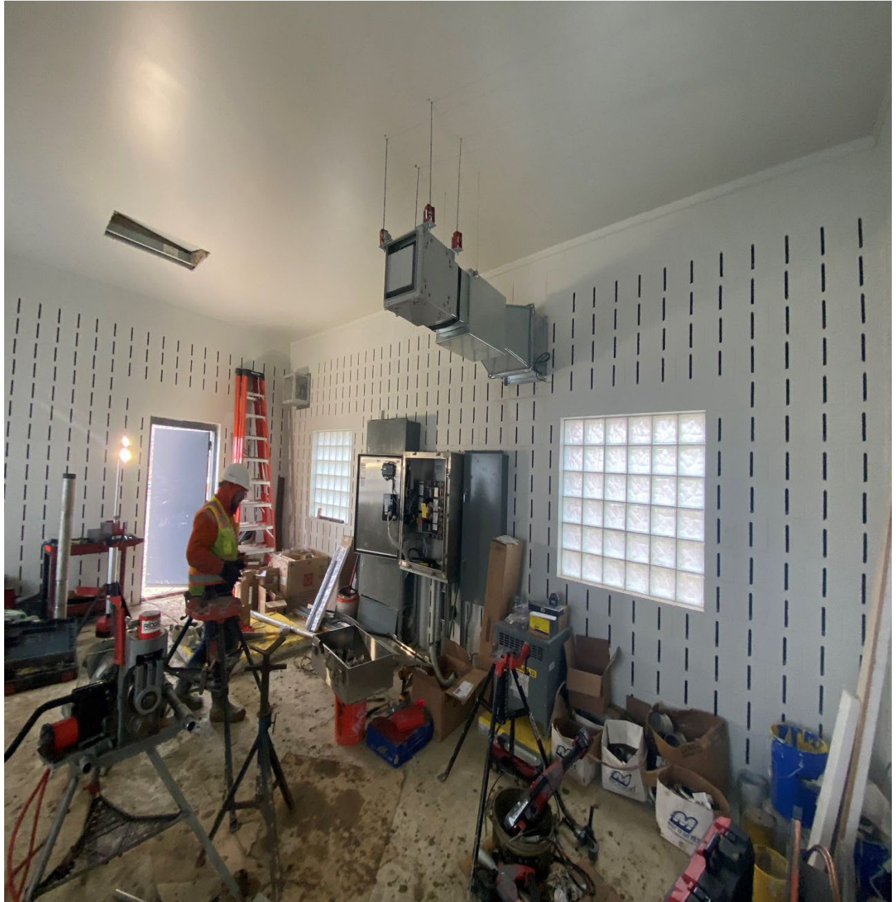
Figure 9 –Installing Elect. Panels @ Beaconsfield Control Bldg.
