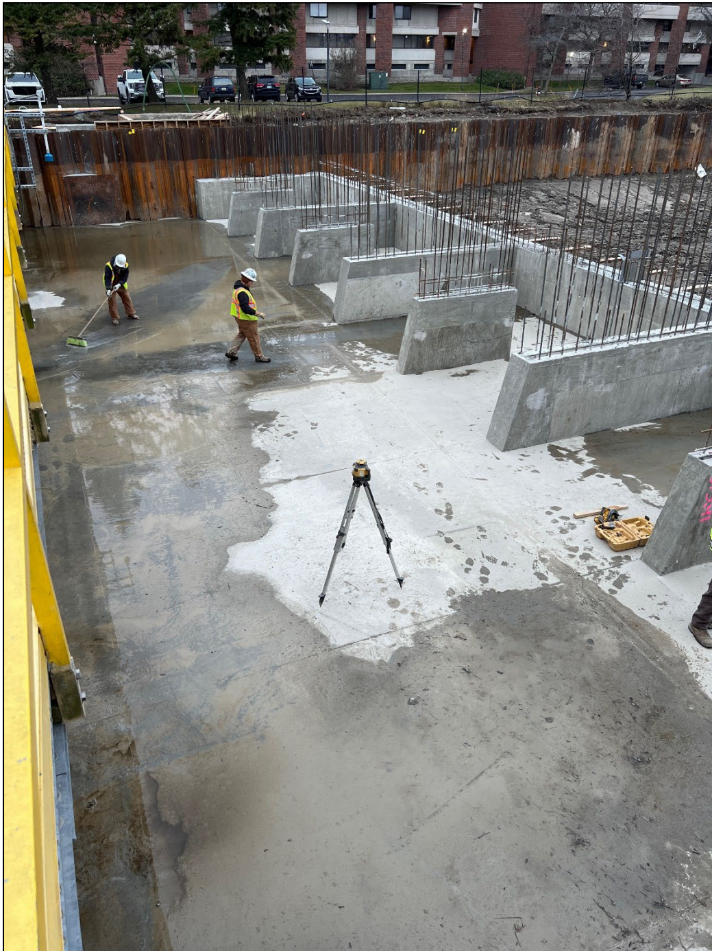
Figure 13 – Outfall Structure Base Slab and Divider Walls
