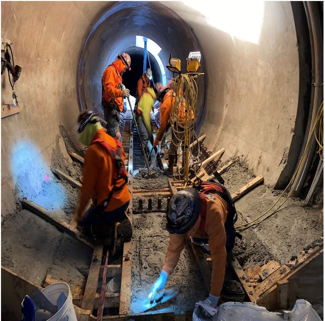
Figure 5 – Placing Concrete for Rubber Dam Bench in 8.5 Tunnel
