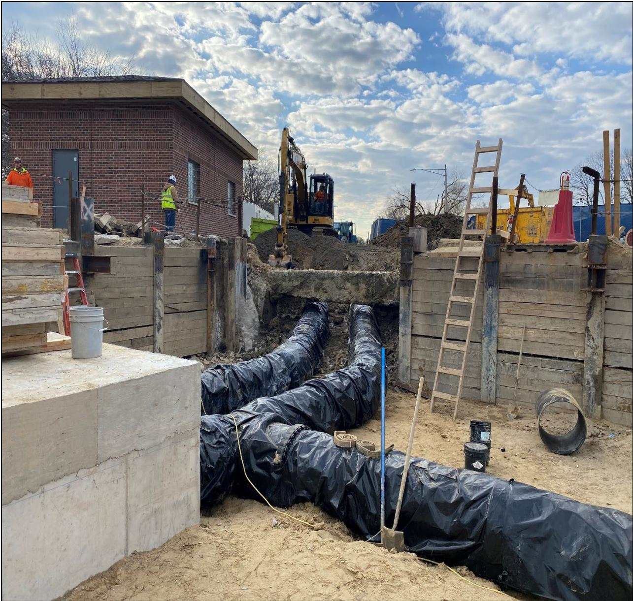
Figure 6 – Removing 8.5 Tunnel Concrete inside Beaconsfield West Vault Access
