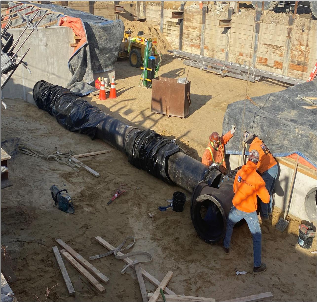
Figure 5 – Installed 24in Ventilation Pipe under Beaconsfield Road
