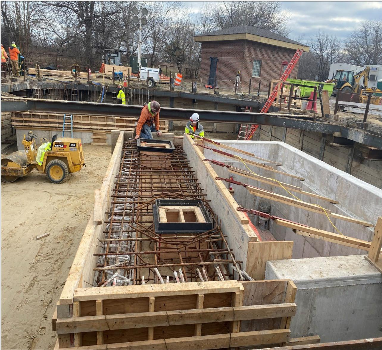
Figure 2 – Placing Concrete Deck @ Beaconsfield East Access Vault
