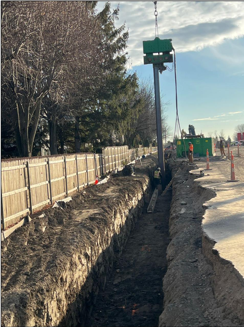
Figure 17 – 8'x8' Emergency Bypass installation (below future Outfall Building)
