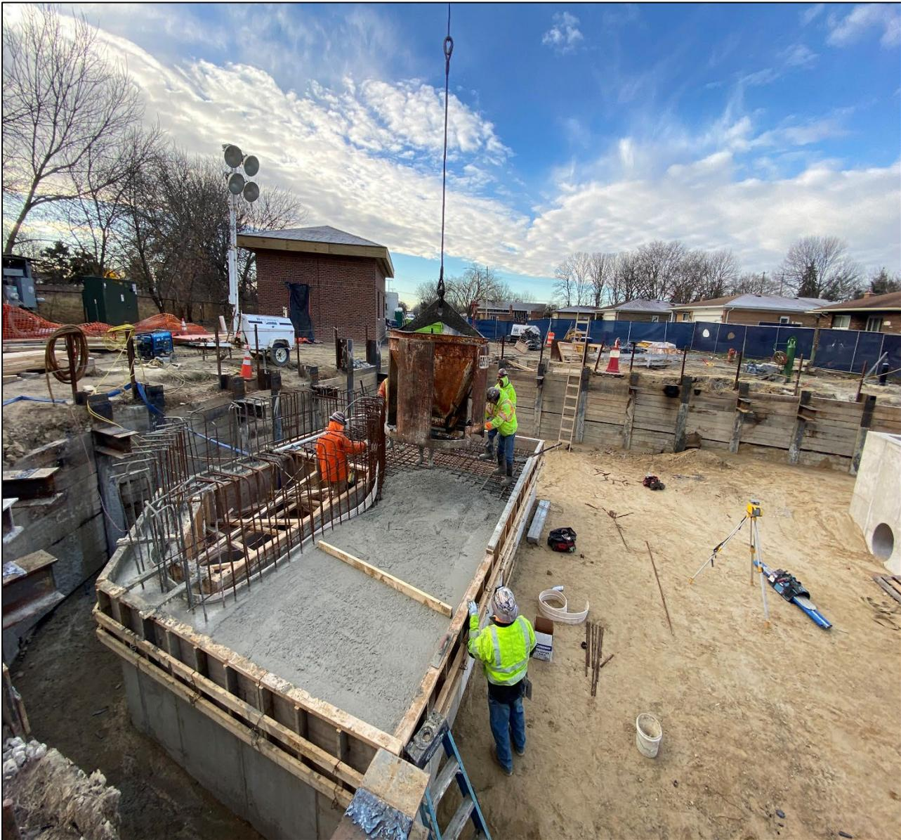
Figure 3 – Compacting & Testing Sand Backfill @ Beaconsfield Shaft
