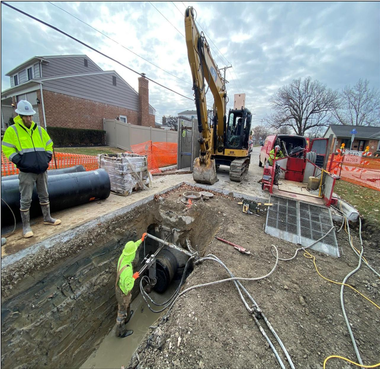
Figure 10 –Installing 24in Ventilation Pipe @ Malvern Street
