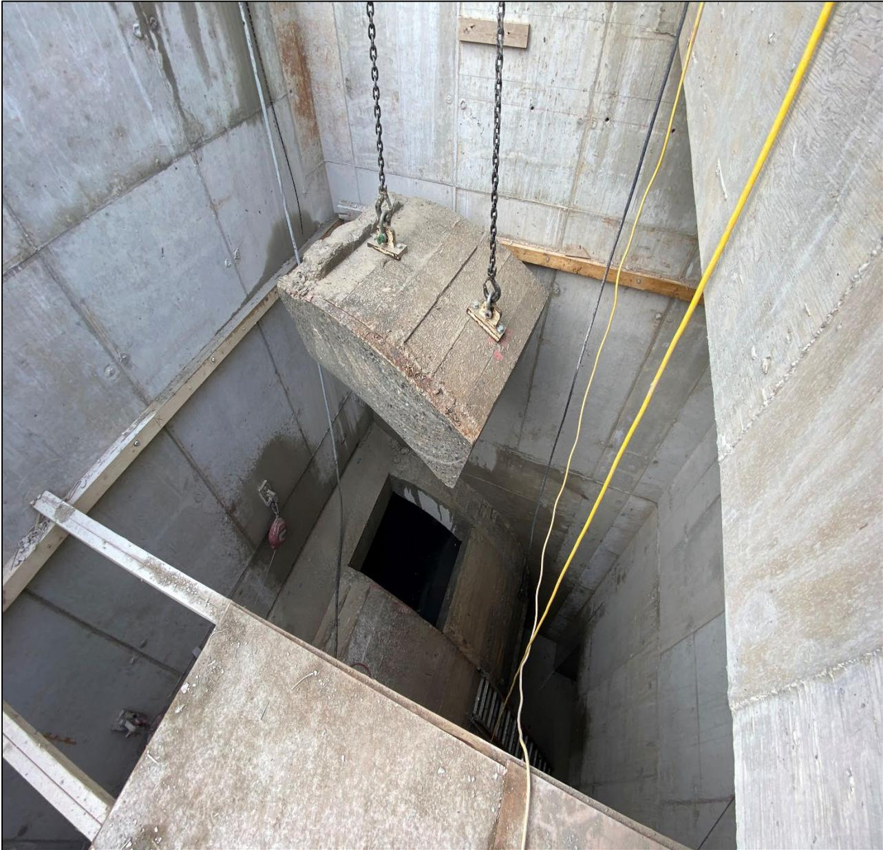
Figure 7 – Cutting 8.5 Tunnel Concrete inside Beaconsfield West Vault
