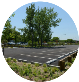
Parking areas incorporating green stormwater infrastructure
