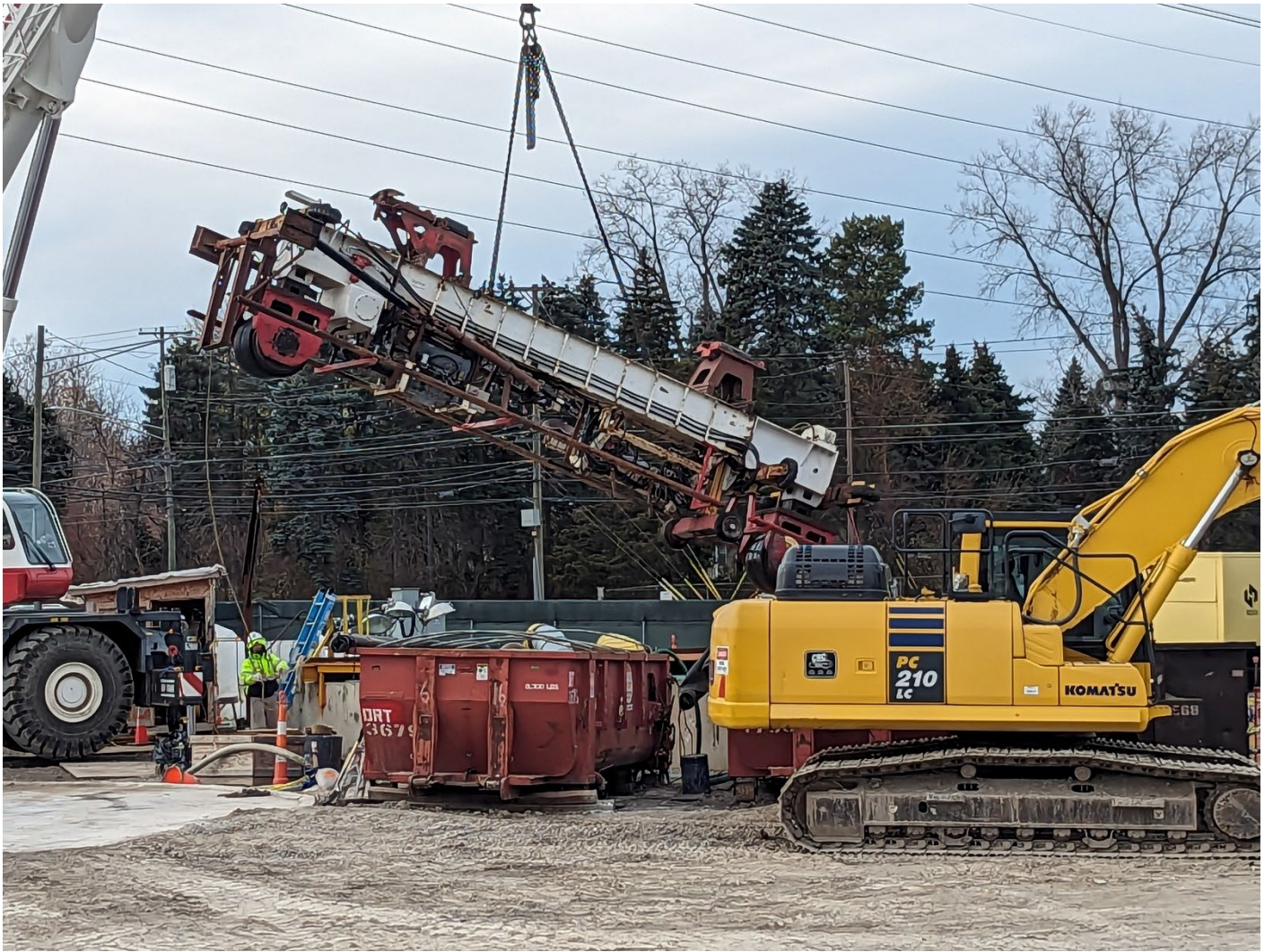
Figure 2 – Pipe Carrier Testing
