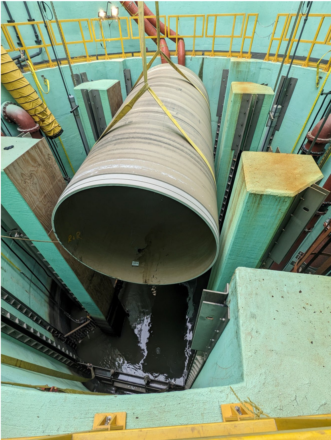
Figure 6 – Lowering in HOBAS to Test Pipe Carrier
