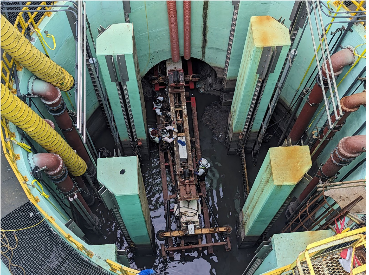
Figure 3 – Pipe Carrier Testing
