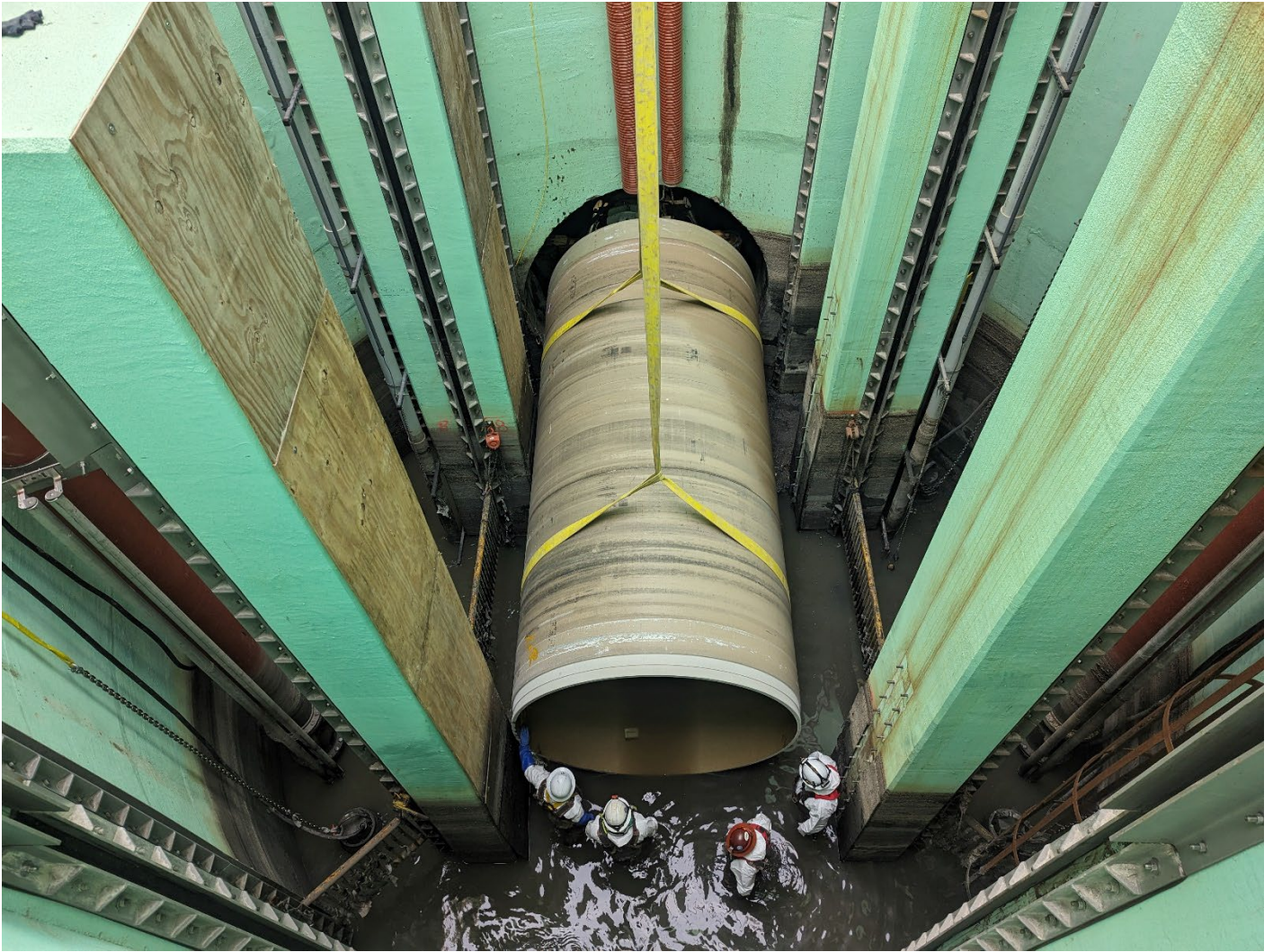
Figure 5 – Pipe Carrier Testing with HOBAS Pipe
