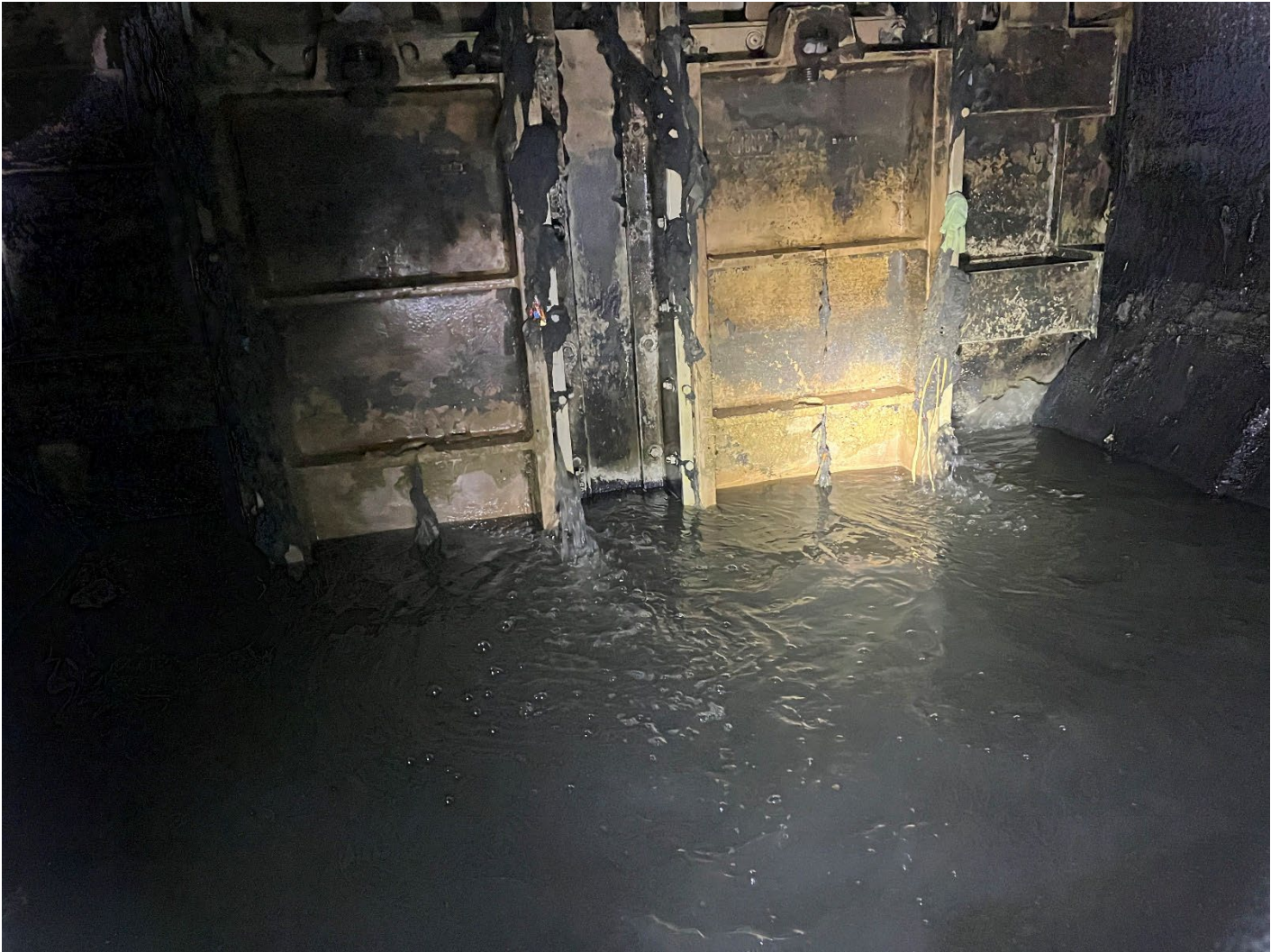
Figure 11 – CS-3 Gates – View from Upstream
