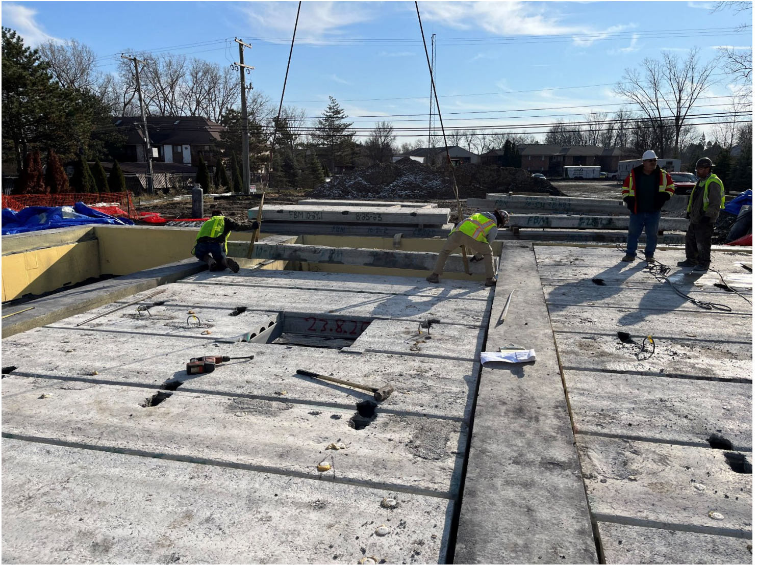
Figure 20 – Fraser Bio-Filter Roof Slab Installation
