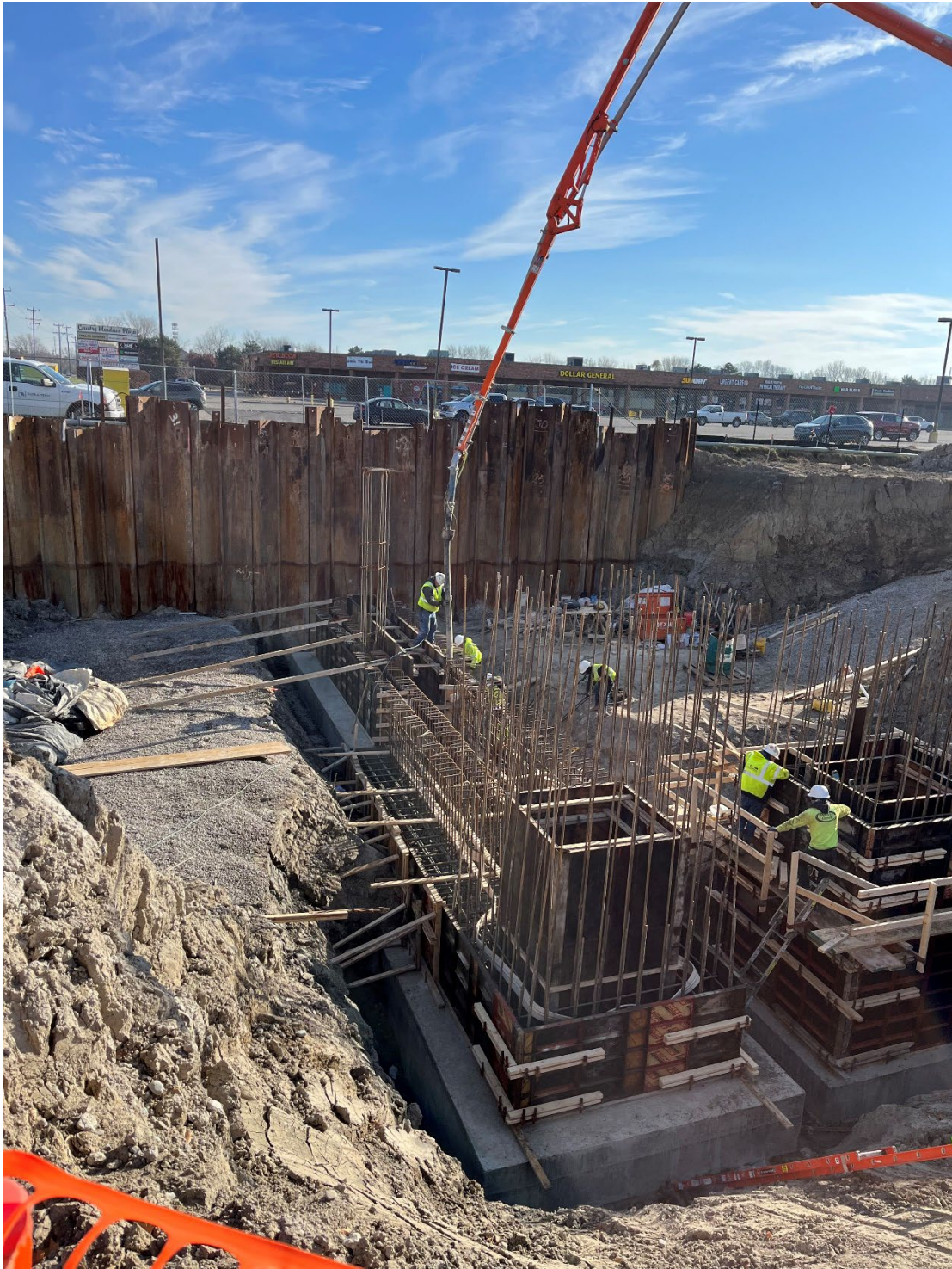
Figure 23 – Macomb Bio-Filter Media Chamber Foundation Construction
