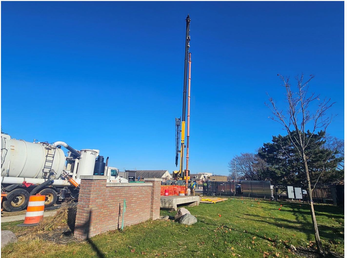
Figure 9 – Cleaning Setup at CS-3
