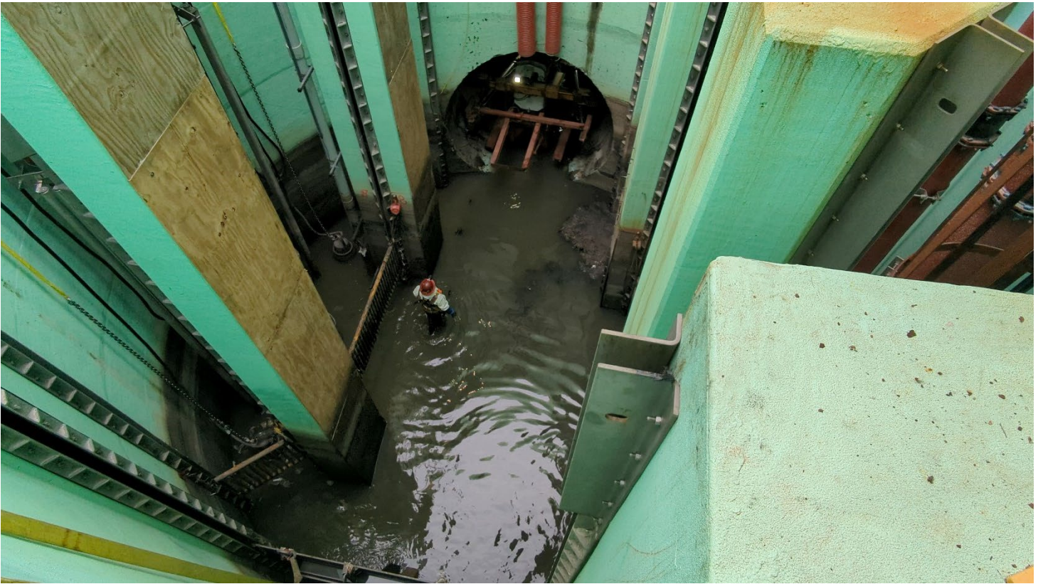
Figure 4 – Pipe Carrier Testing
