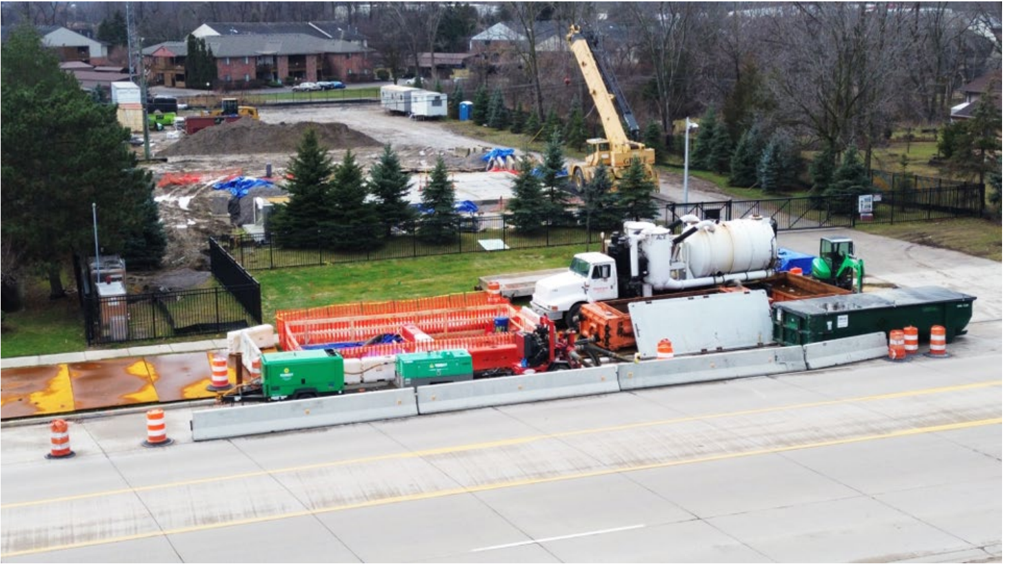
Figure 7 – Aerial View at CS-3 of Debris Removal Equipment
