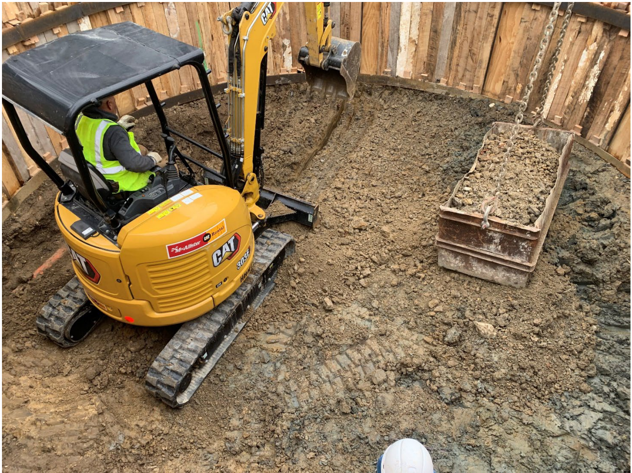
Figure 15 – Lining Completion Shaft Excavation
