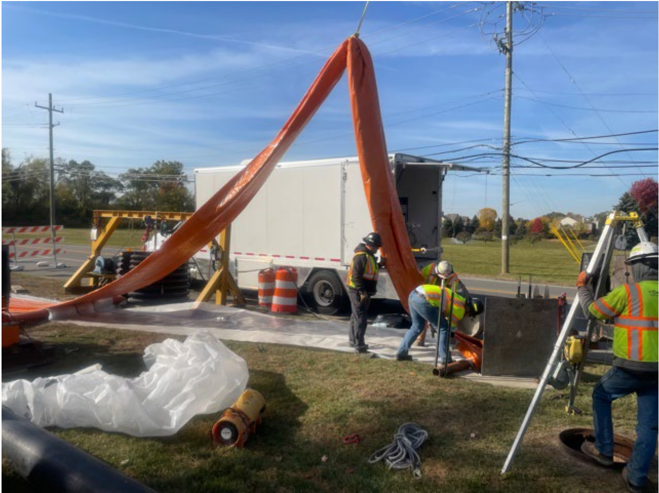
Figure 6 – CT-S-7 CIPP Liner Installation
