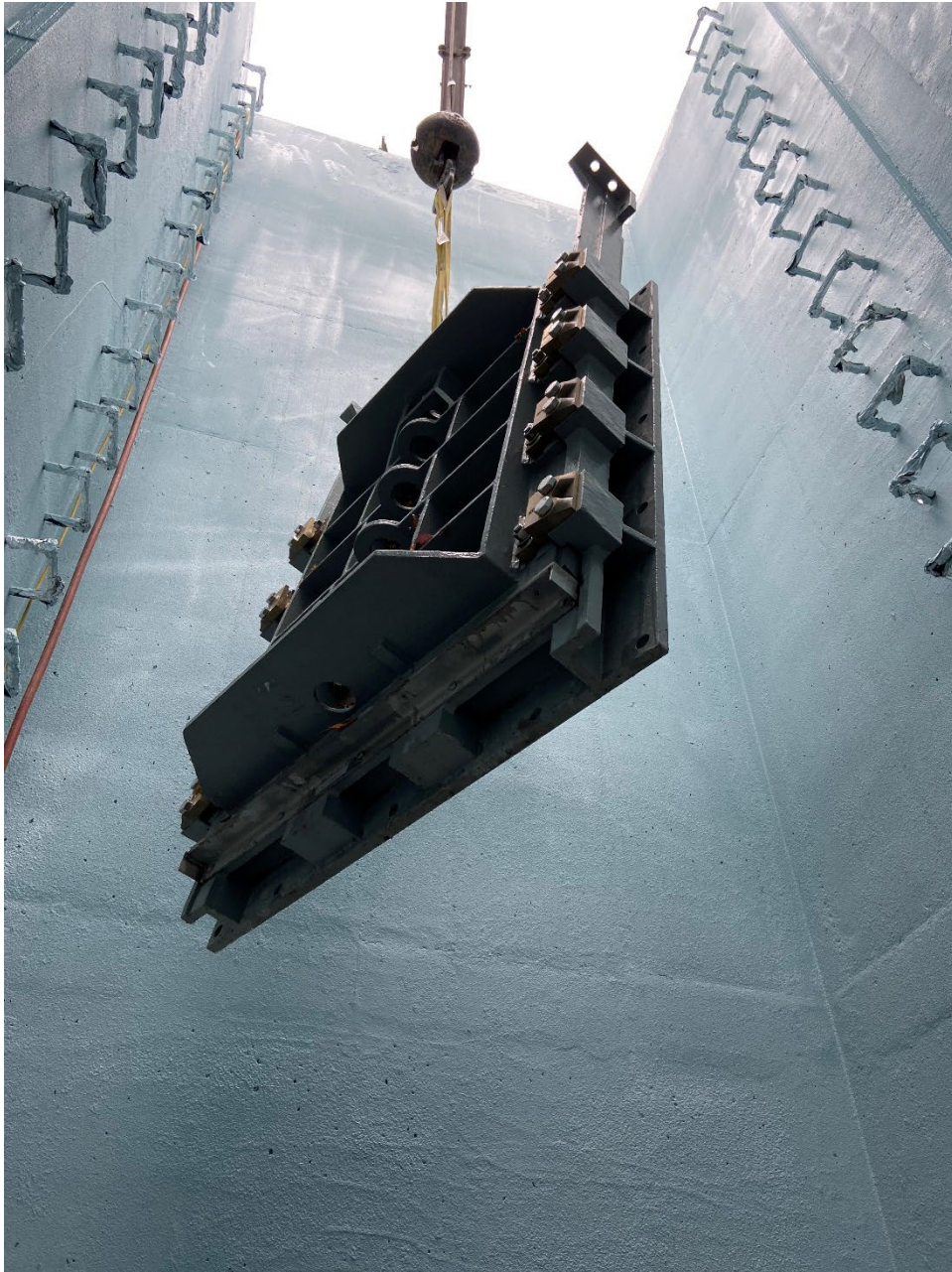
Figure 11 - CS-13 Gate Installation
