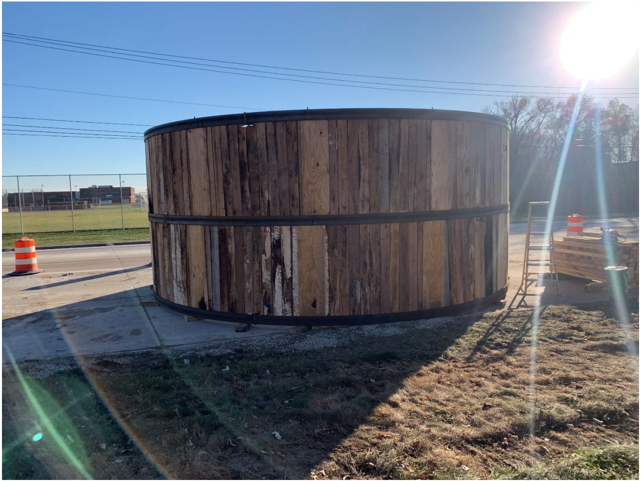
Figure 14 – Lining Completion Shaft TERS
