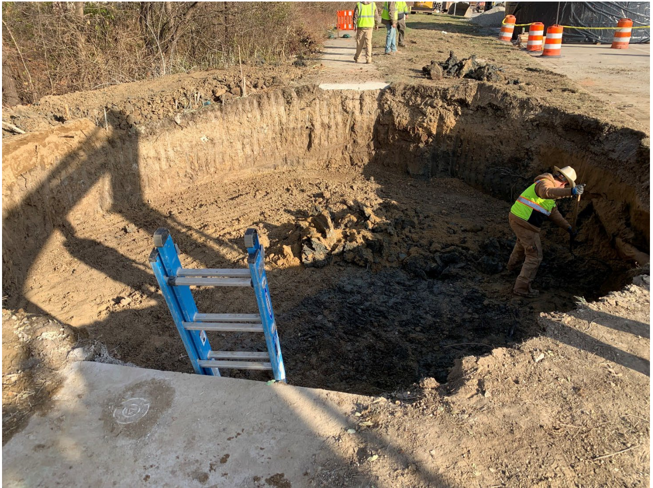
Figure 13 – Lining Completion Shaft Excavation
