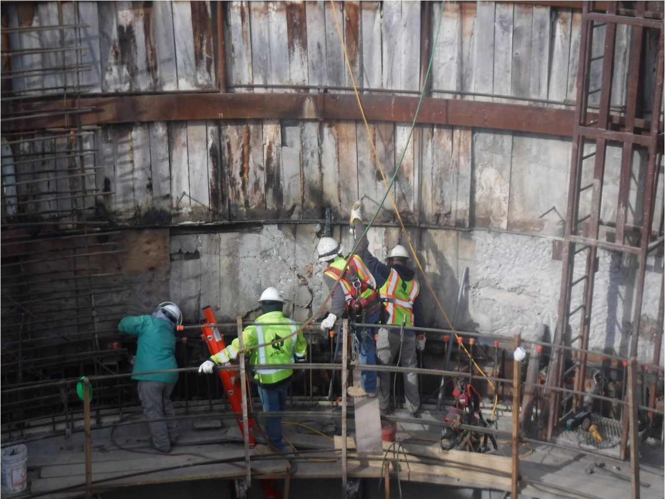
Figure 3 – CS-12 Partial TERS Removal to Facilitate Re-bar Installation
