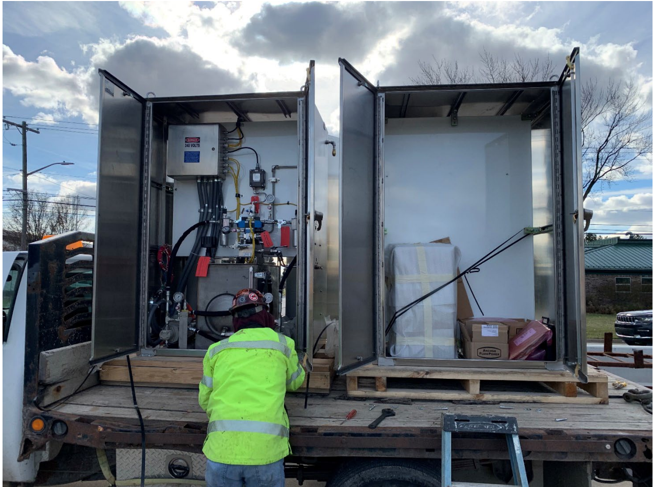
Figure 8 - CS-13 Equipment Cabinets Delivered
