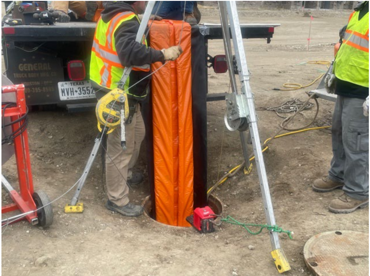
Figure 7 – CT-S-7 CIPP Liner Installation
