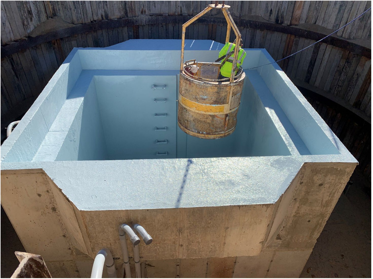
Figure 10 - CS-13 Application of Protective Epoxy Coating
