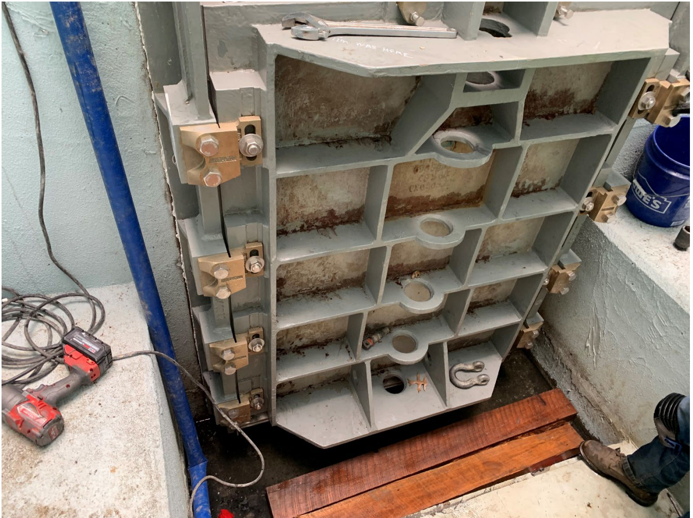
Figure 12 – CS-13 Gate Installation
