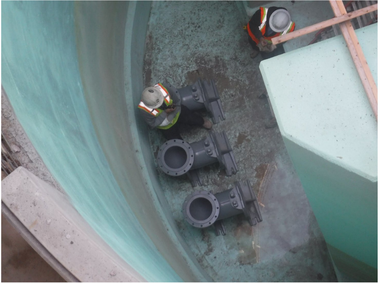
Figure 5 - CS-12 Dry-fitting Pumps
