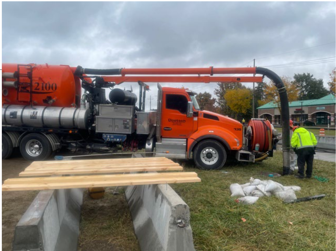
Figure 1 – Cleaning CT-S-7 Drop Manhole Prior to Spray-Lining
