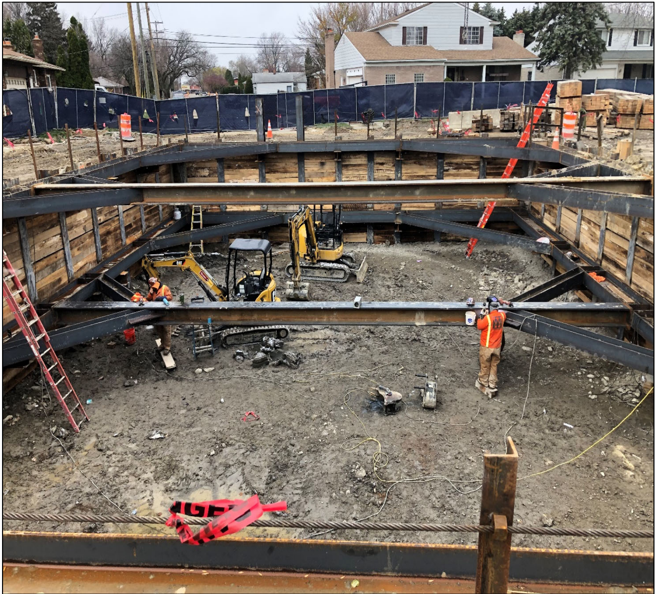
Figure 2 – Middle Tier Bracing and Support Layout
