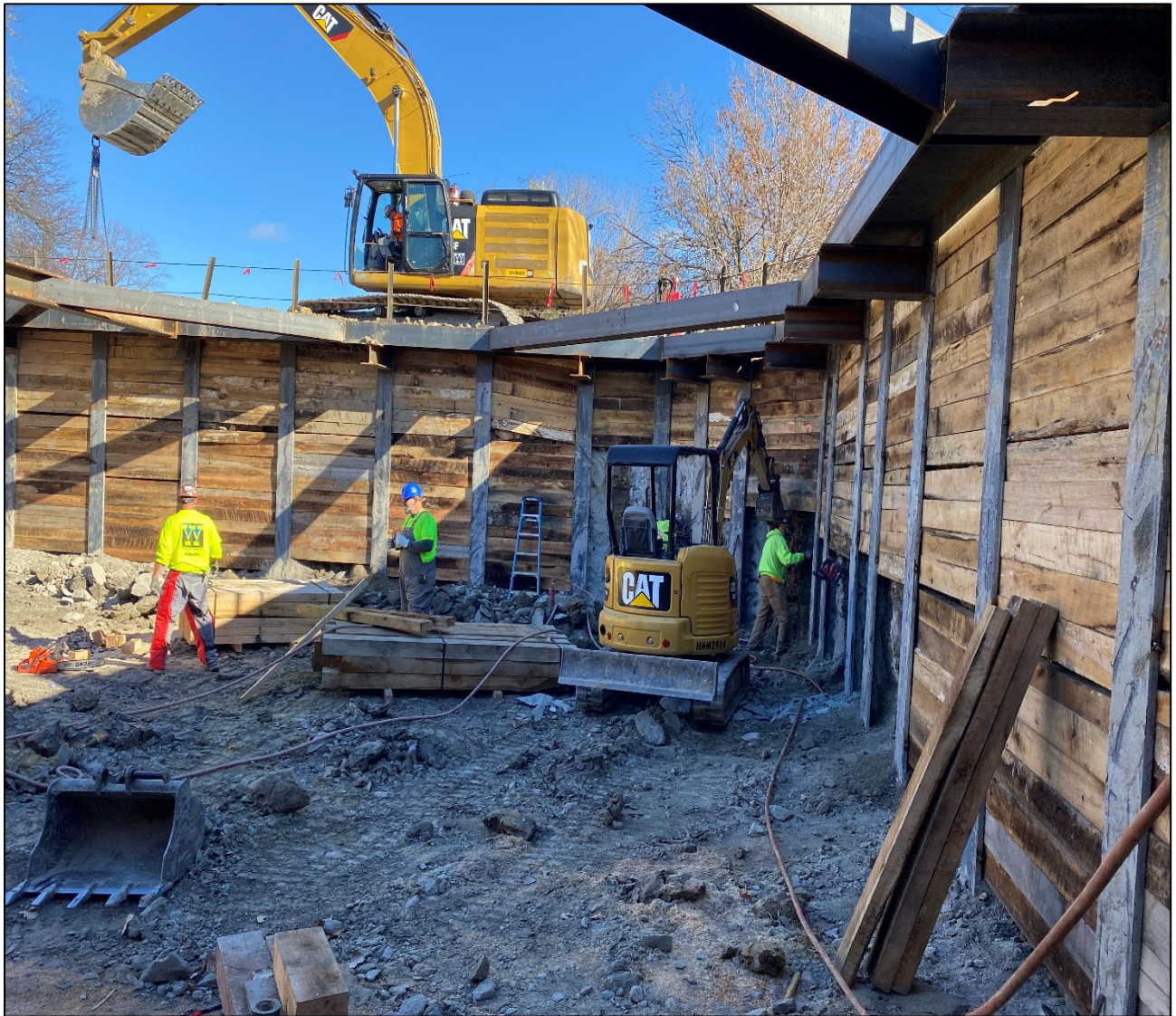
Figure 1 – Installing Timber Retaining Walls
