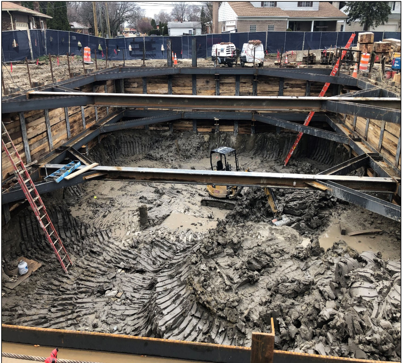
Figure 3 – Beaconsfield Shaft Excavation @ Approx. 20FT
