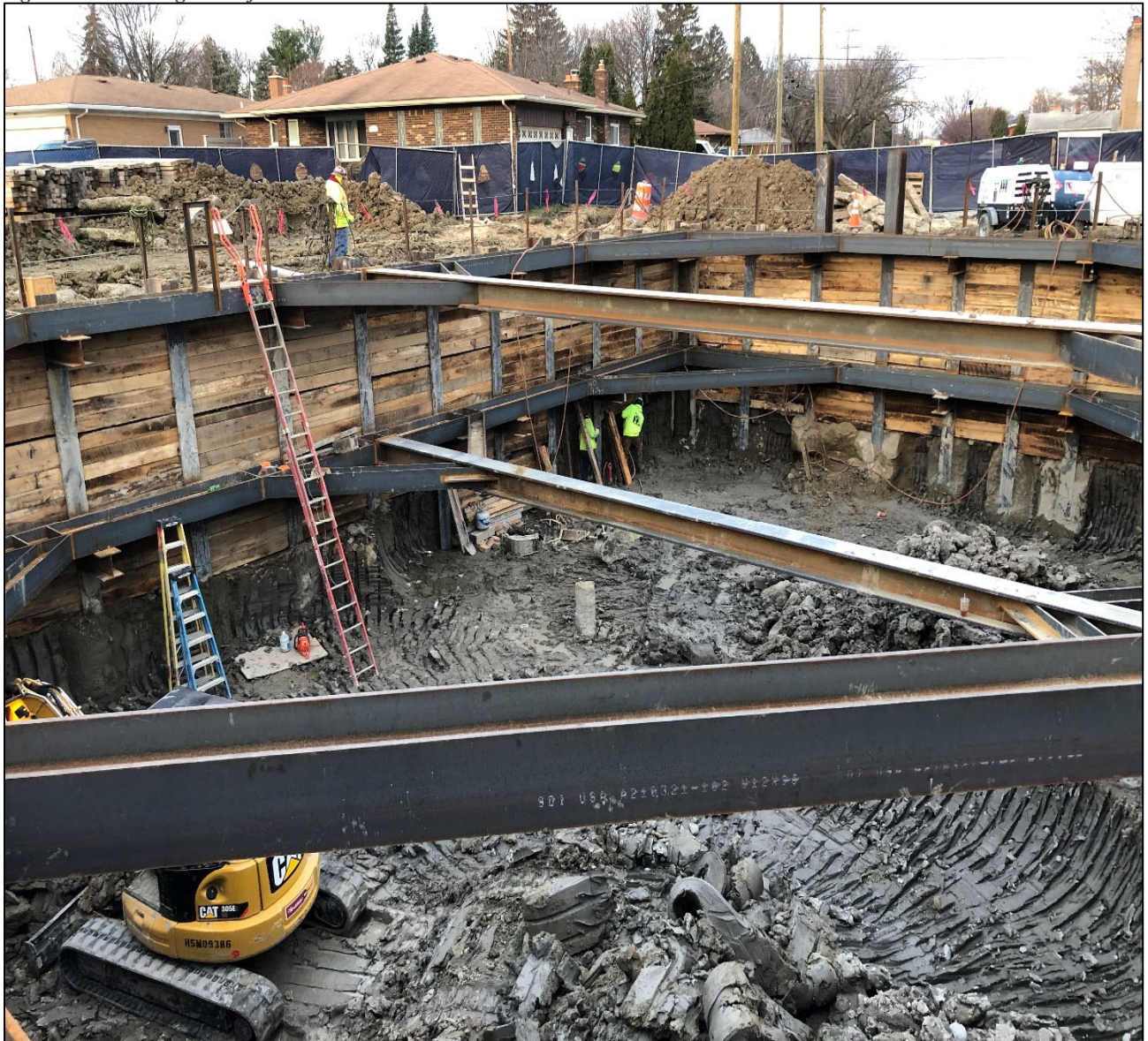
Figure 4 – Removing Grout from Drilled I-Beams
