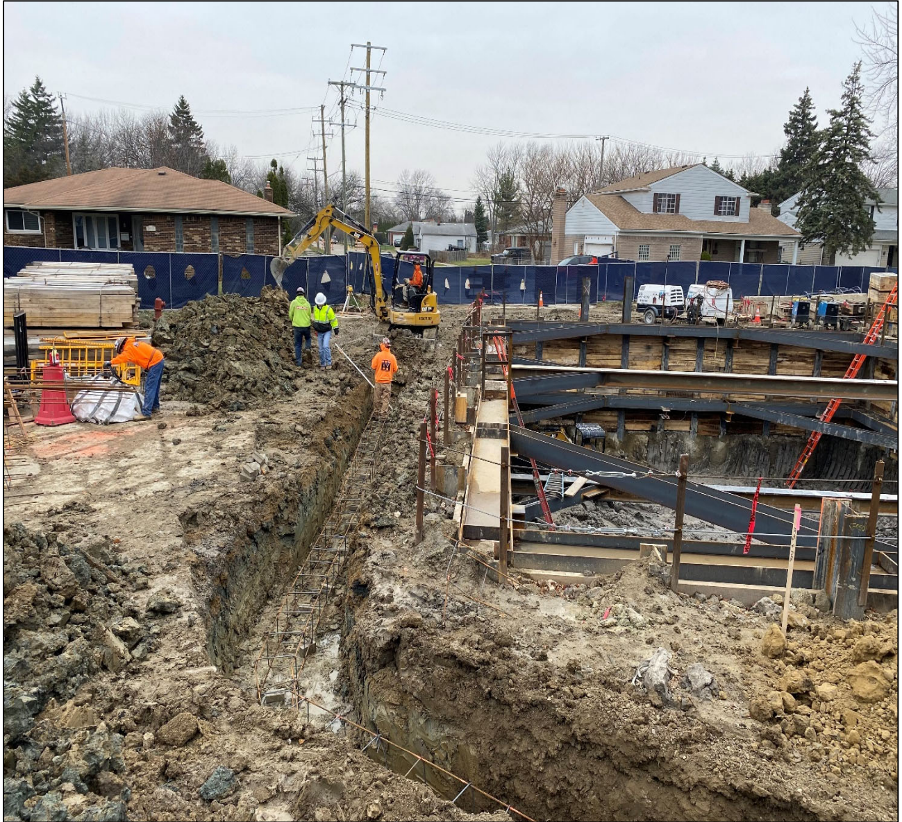
Figure 6 – Beaconsfield Electrical Duct Bank Excavation
