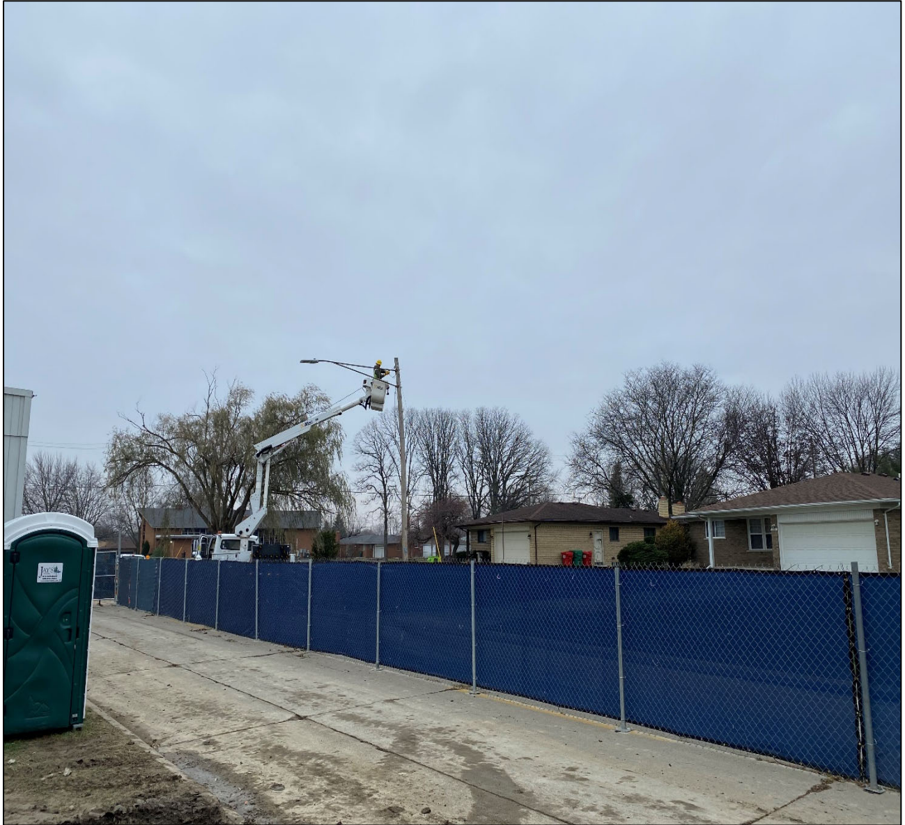
Figure 5 – Reconnecting Street Lighting on Beaconsfield
