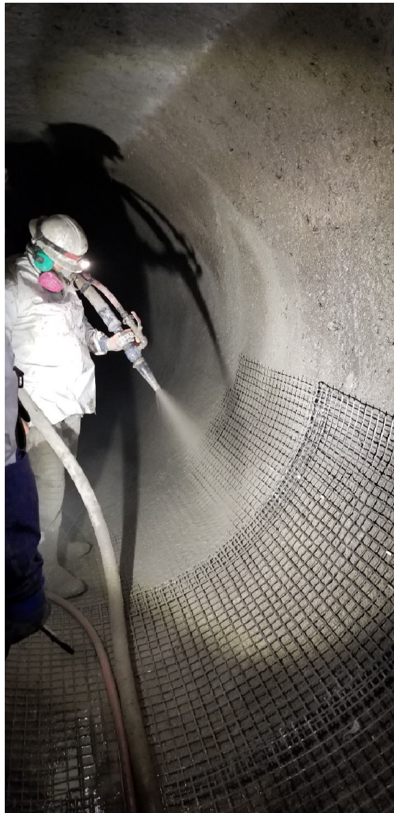
Figure 1 - Geo-Polymer Spray Lining in PCI-37
