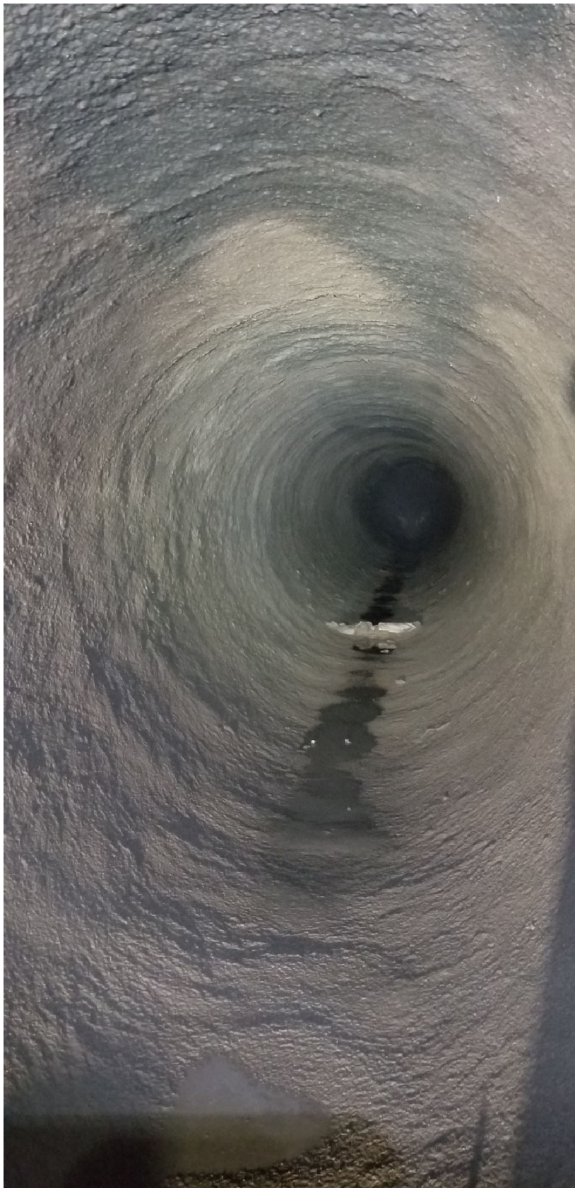
Figure 7 - PCI-37 Dewatered Post Spray Lining
