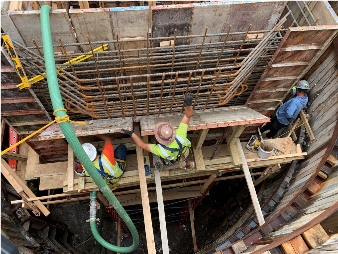
Figure 8 - CS-13 Formwork Installation
