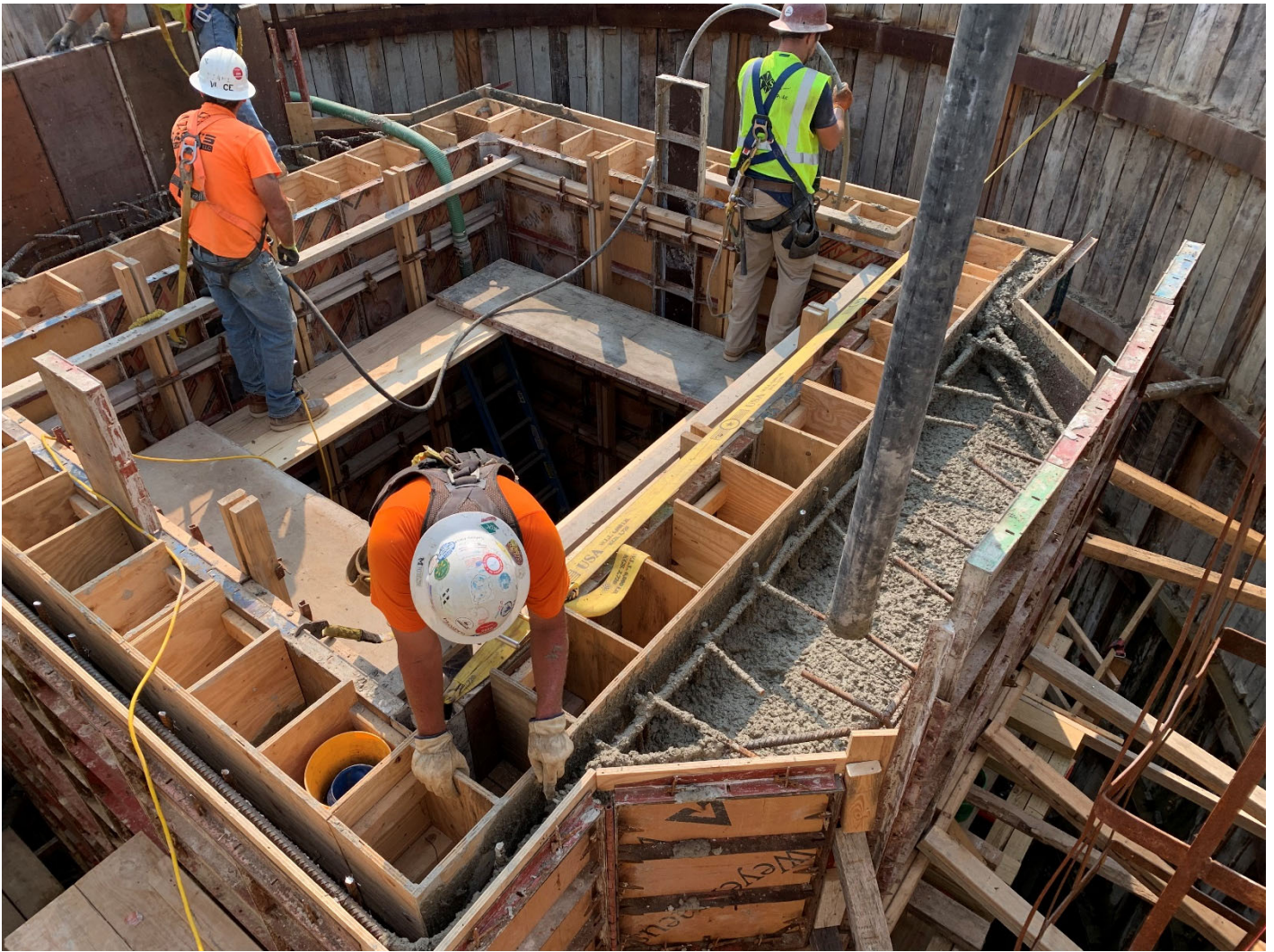
Figure 9 - CS-13 Concrete Placement
