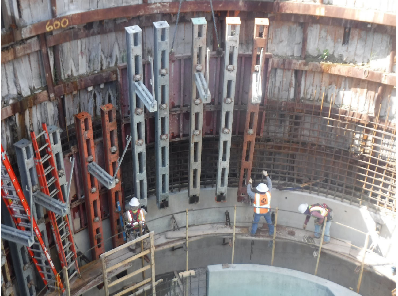
Figure 4 - CS-12 Wall Formwork Installation
