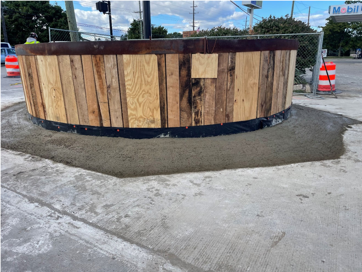
Figure 14 - Manhole #1 TERS after backfill
