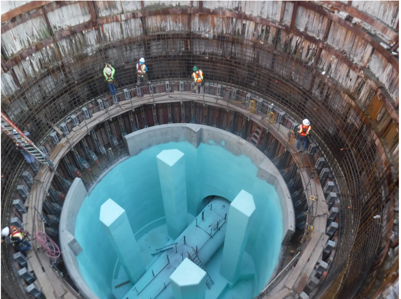
Figure 2 - CS-12 Rebar Installation
