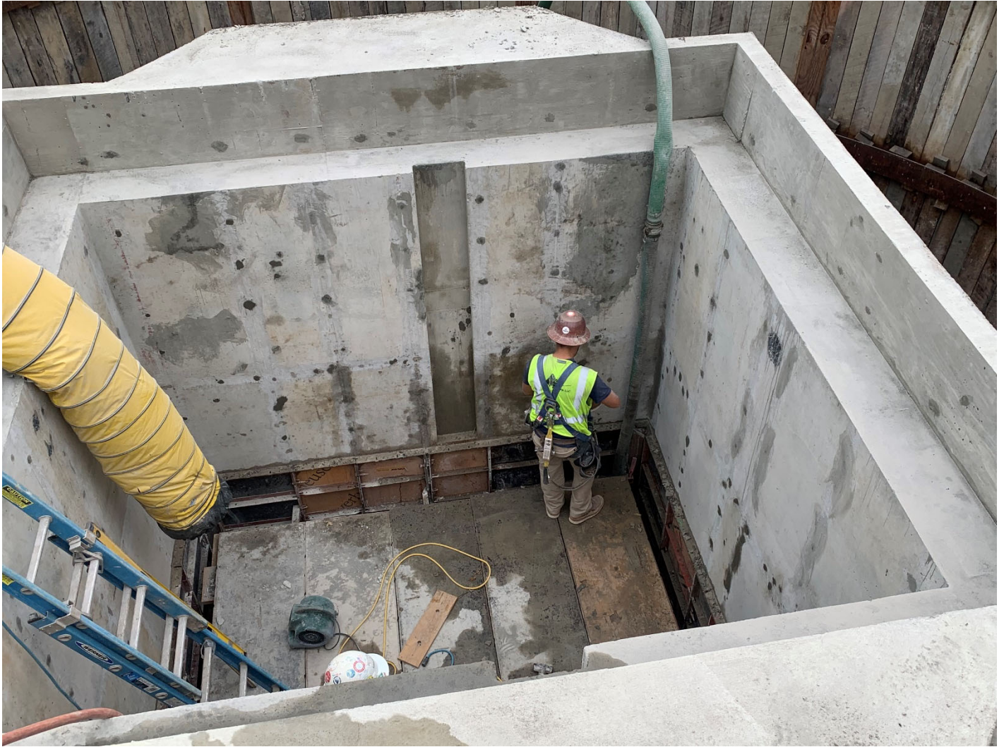
Figure 10 - CS-13 Formwork Removal
