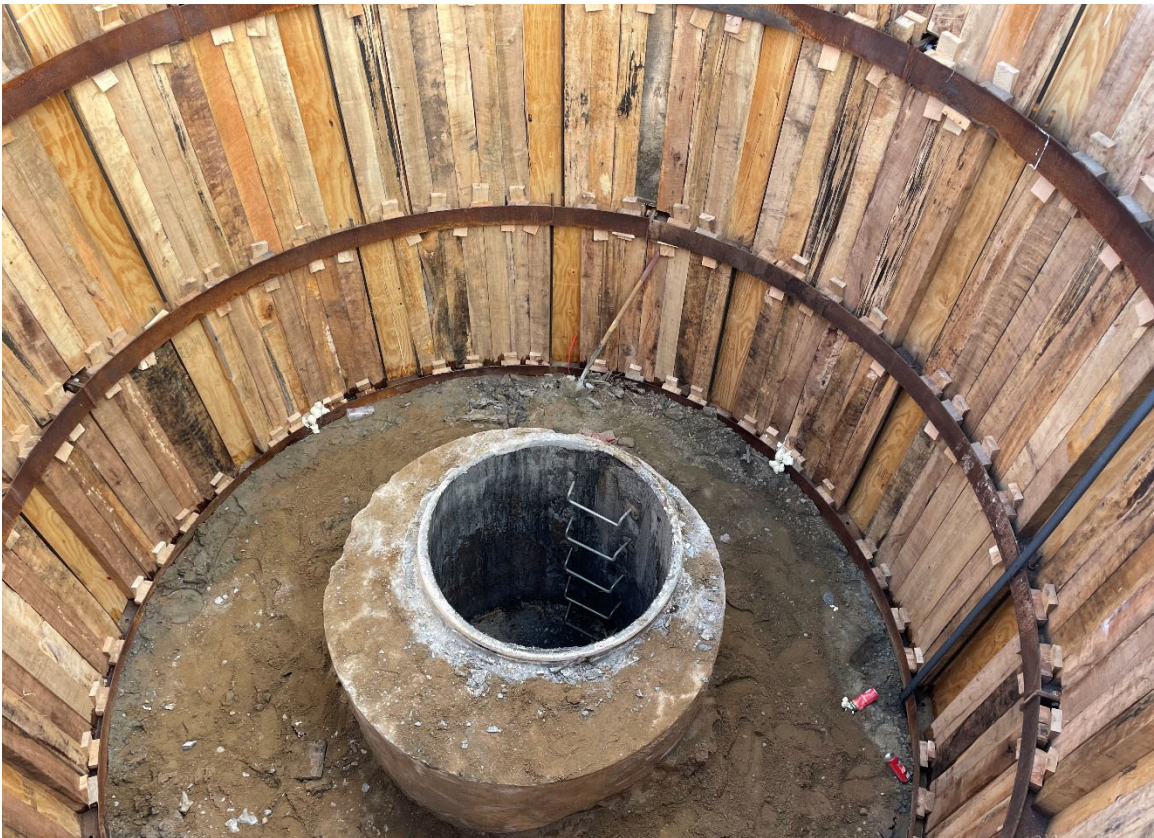
Figure 15 - Manhole #1 TERS Shaft
