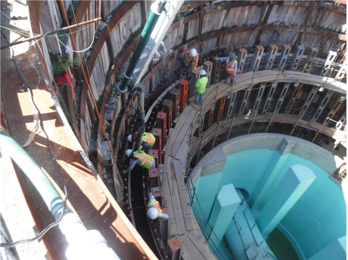
Figure 3 - CS-12 Wall Concrete Placement
