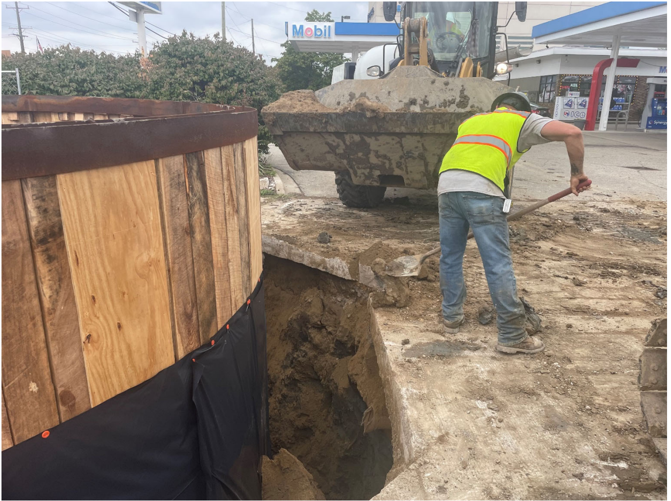
Figure 13 - Manhole #1 TERS Placed in Excavation
