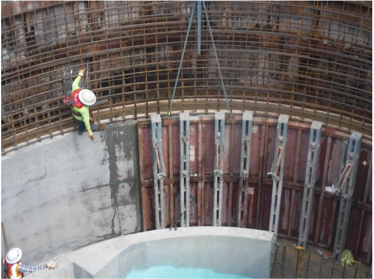
Figure 5 - CS-12 Wall Formwork Removal
